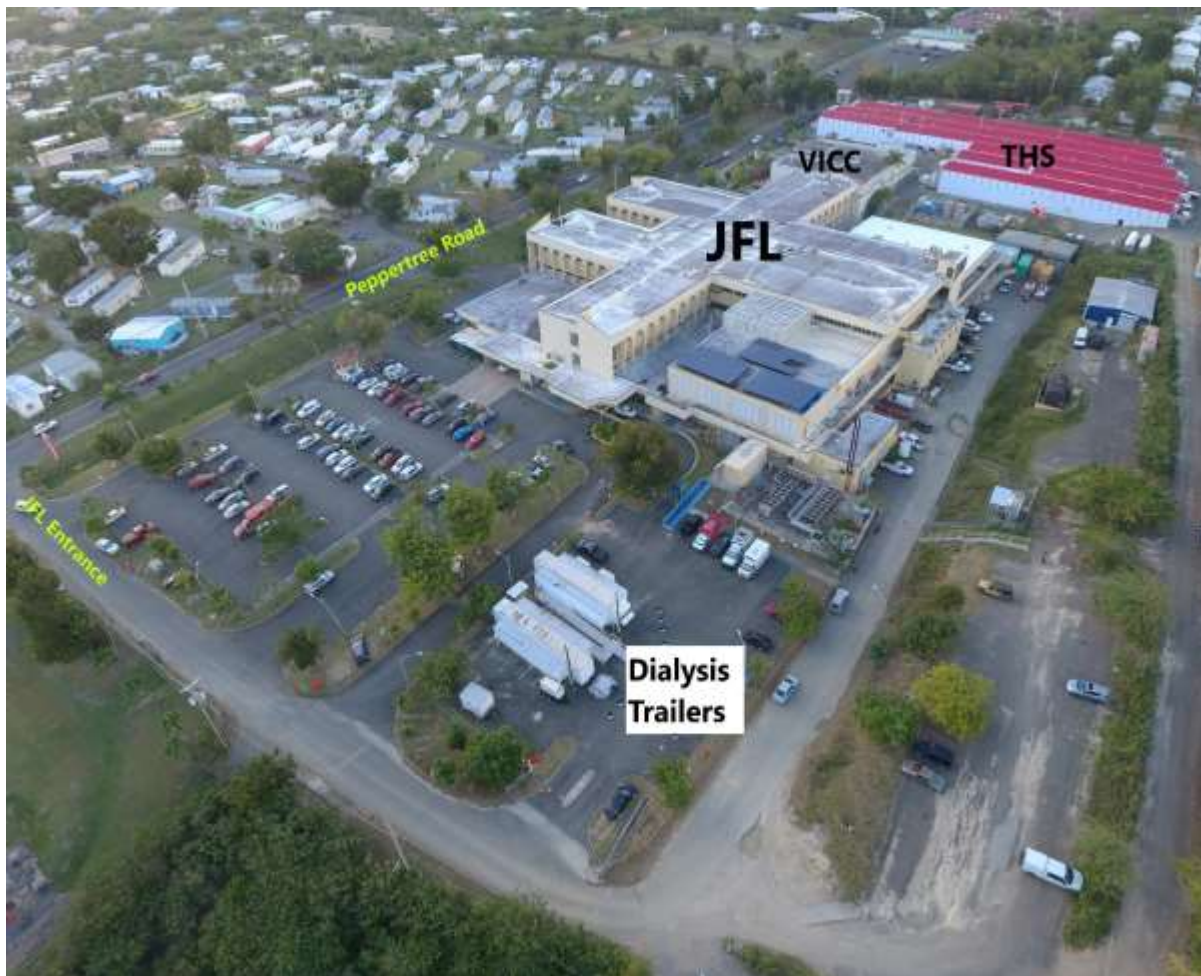
Figure 1 of 5: Aerial View of the JFL Campus at 4007 Estate Diamond Ruby
