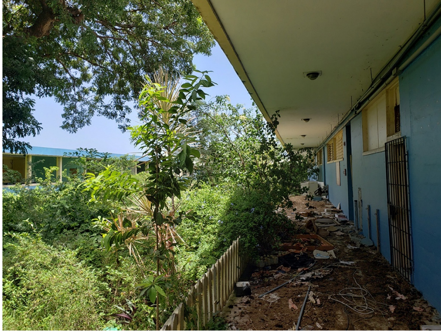
Photo 3: View of Existing Buildings Condition
