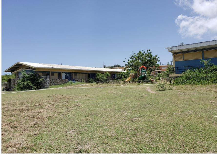
Photo 5: View of Existing Buildings and Playground
