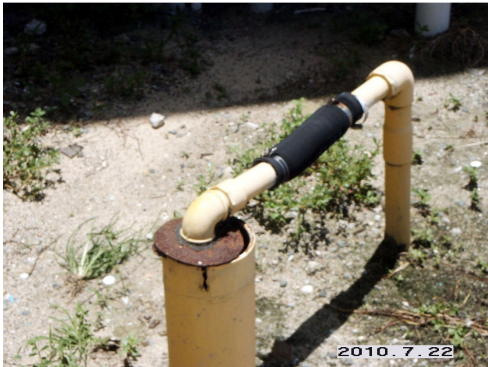
Figure IV.C.11. Laundromat well without effective seal.
