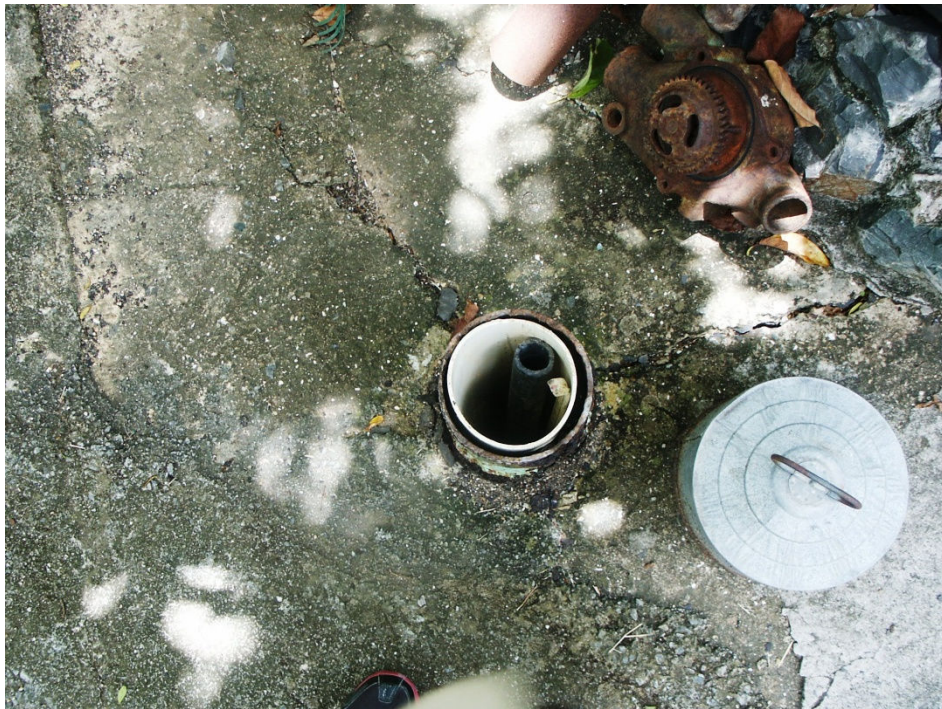
Figure IV.C.14. What's under the cover; this abandoned well is adjacent to a production well providing potable water.
