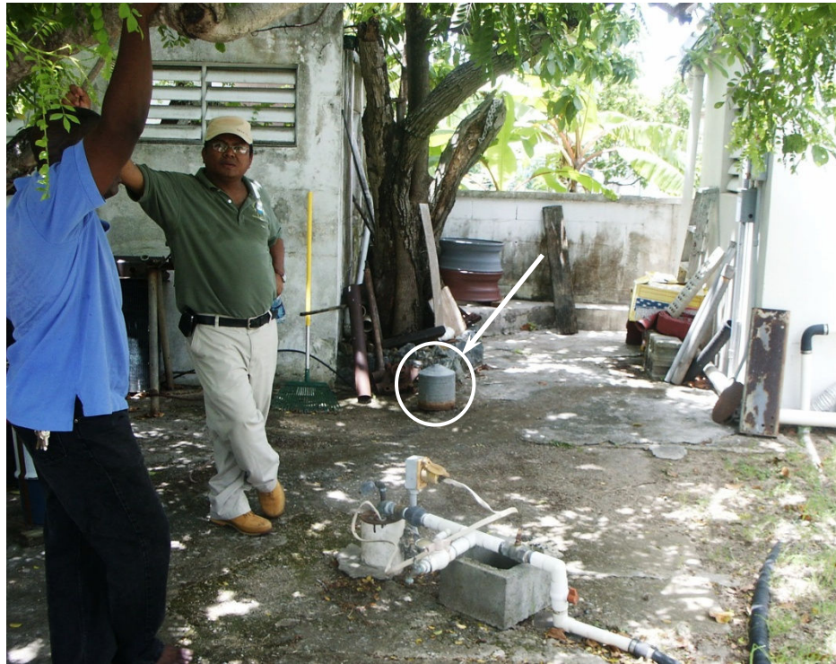
Figure IV.C.13. Production well for vendor; note the galvanized cover.
