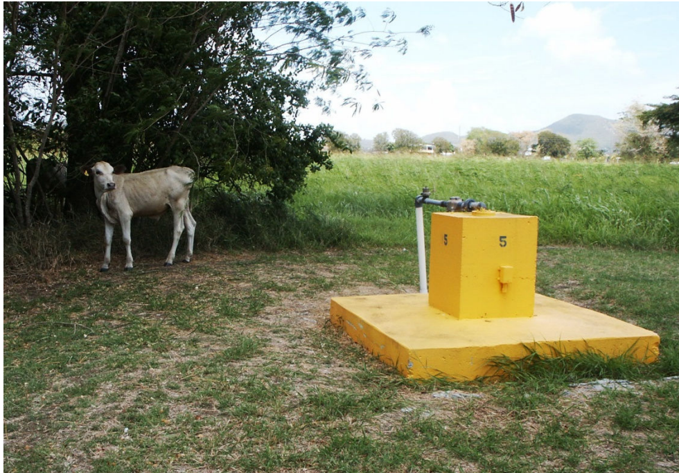
Figure IV.C.1. WAPA well with typical platform and riser.
