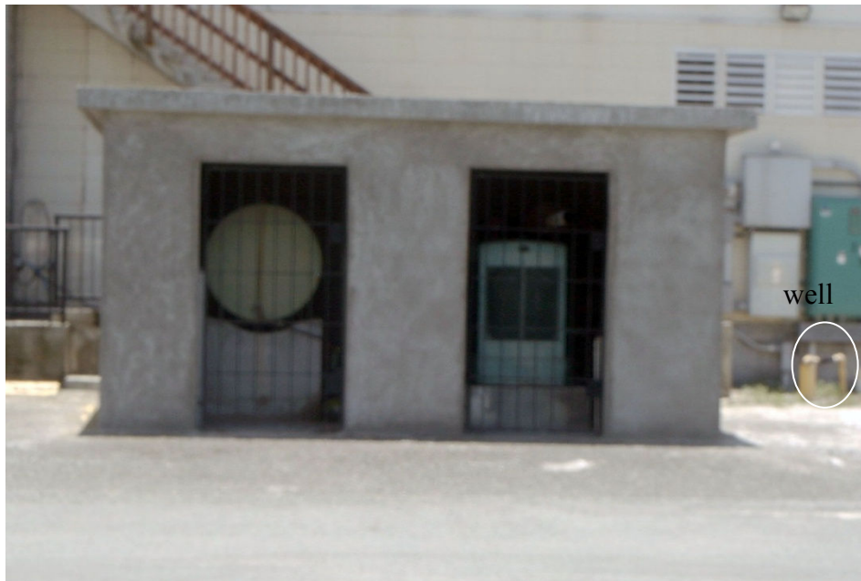
Figure IV.C.12. Diesel tank without containment adjacent to well.
