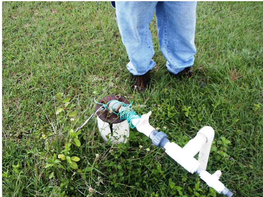
Figure IV.C.6. Wellhead with compromised sanitary seal and cut in casing.
