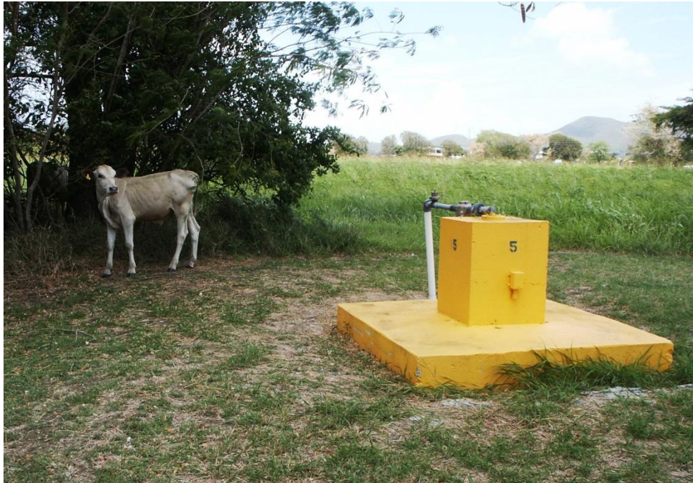
Figure IV.C.10. WAPA well with typical platform and riser.
