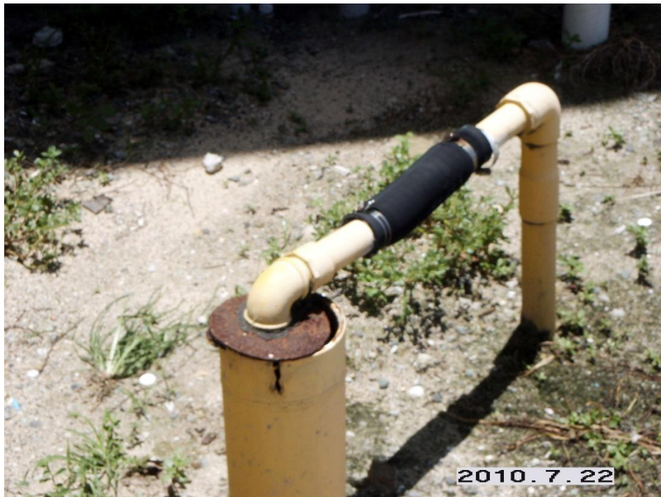
Figure IV.C.20. Laundromat well without effective seal.
