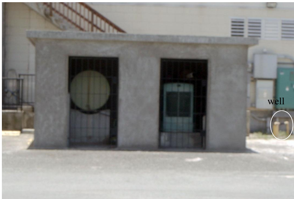
Figure IV.C.21. Diesel tank without containment adjacent to well.
