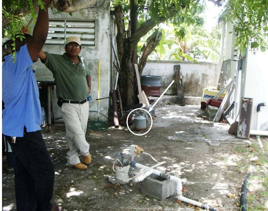
Figure IV.C.22. Production well for vendor; note the galvanized cover.
