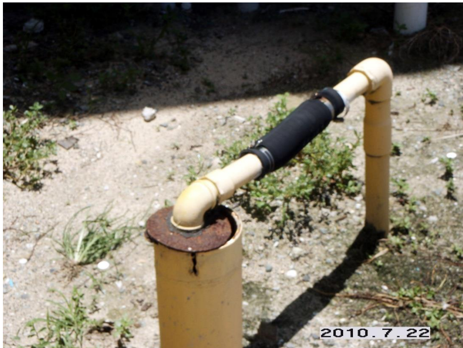
Figure IV.C.20. Laundromat well without effective seal.
