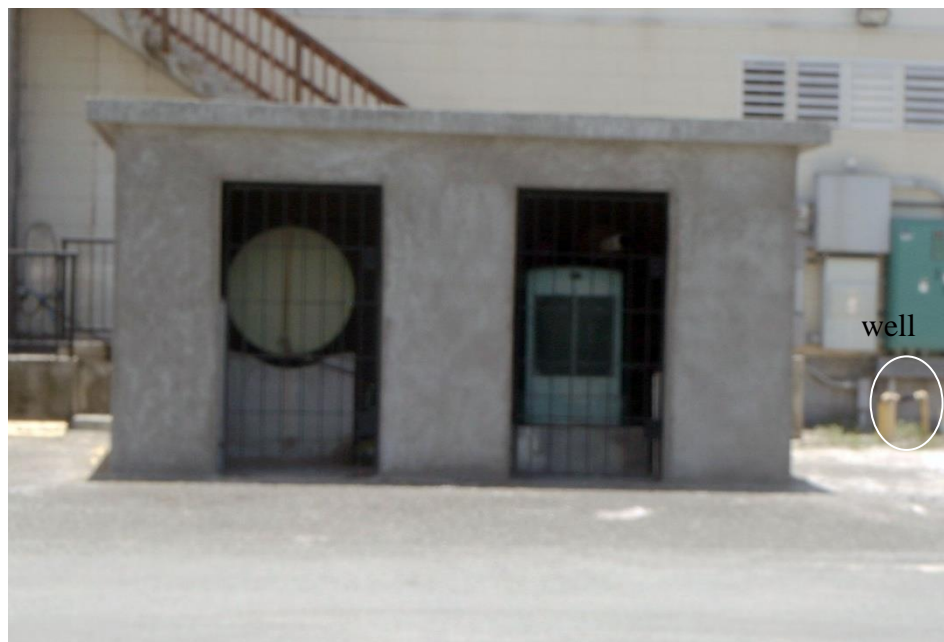
Figure IV.C.21. Diesel tank without containment adjacent to well.
