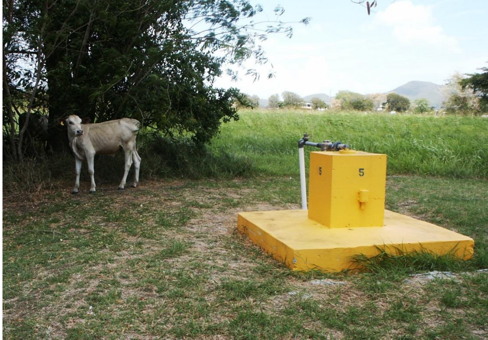
Figure IV.C.10. WAPA well with typical platform and riser.
