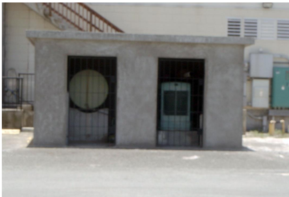
Figure IV.C.21. Diesel tank without containment adjacent to well.
