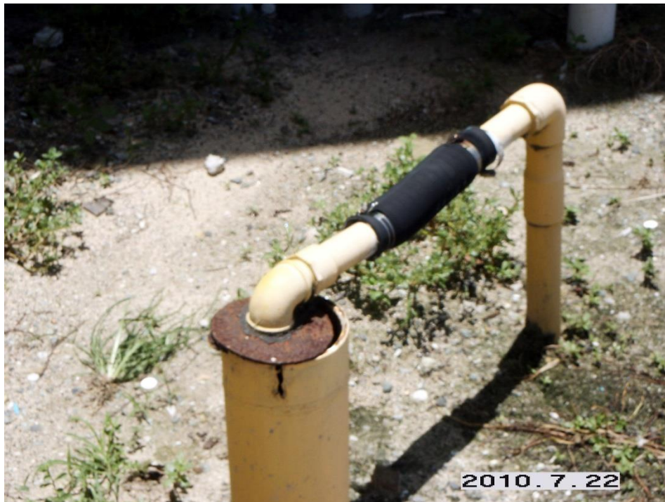
Figure IV.C.20. Laundromat well without effective seal.
