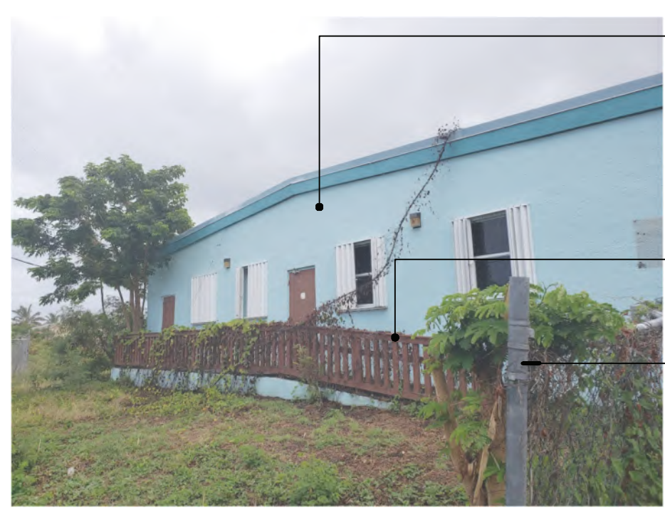
VIEW TOWARDS BUILDING - SOUTH 3
