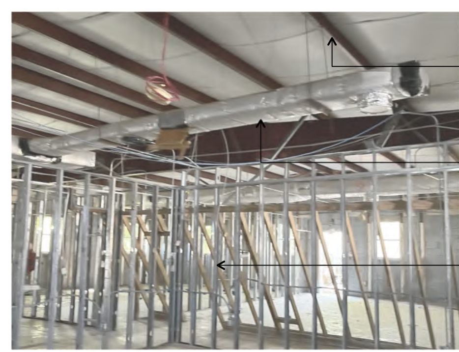
INTERIOR BUILDING VIEW 8
