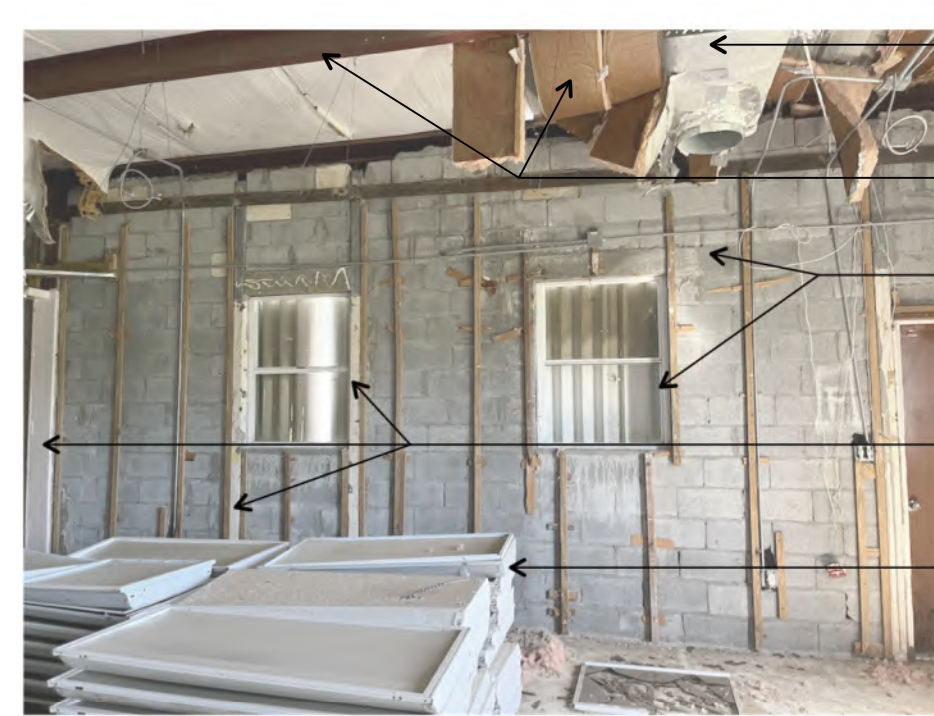
INTERIOR BUILDING VIEW 7
