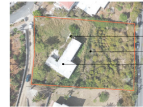
AERIAL VIEW OF BUILDING
