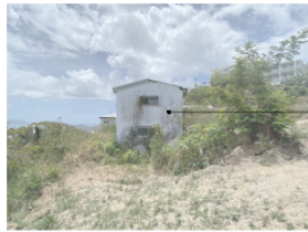
VIEW TOWARDS BUILDING - NORTHWEST SIDE
