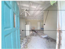
INTERIOR VIEW OF BUILDING - ENTRY
