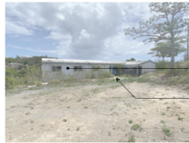
VIEW TOWARDS BUILDING FROM STREET ENTRY
