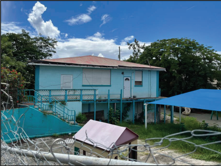
Photo 1: Side View from the Main Roadway
