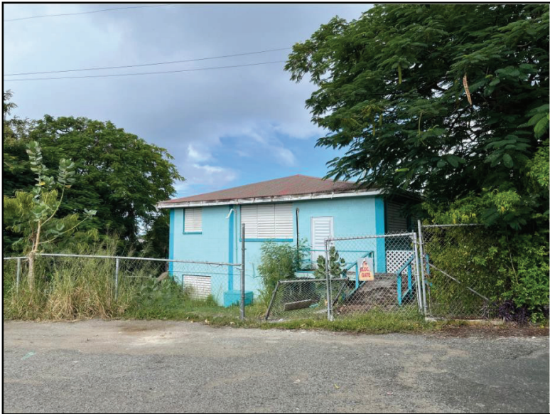
Photo 2: Front View from street
