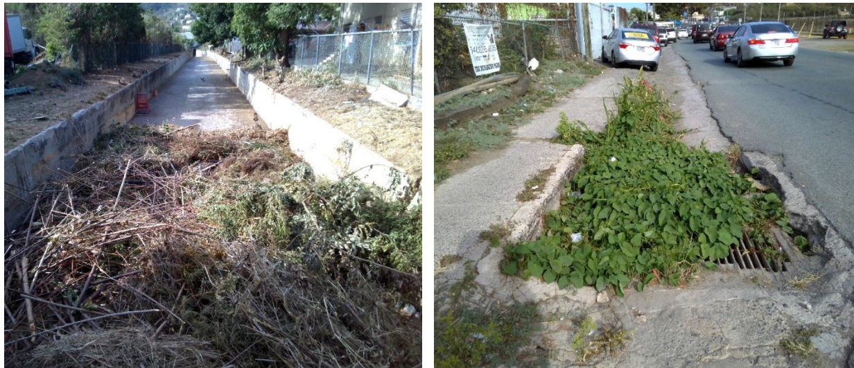
Figure 39. Concrete gut channel clogged by brush and trash (left) and a catchbasin plugged by vegetation with damage to the road to the right of the grate (right).
