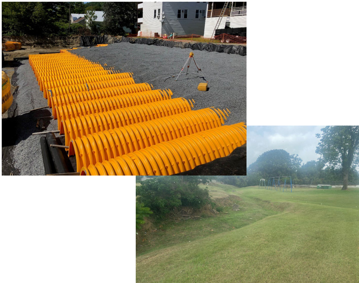
Figure 72. Example photo of subsurface infiltration chambers (above) and greenspace at the Lorraine apartment complex (below).
