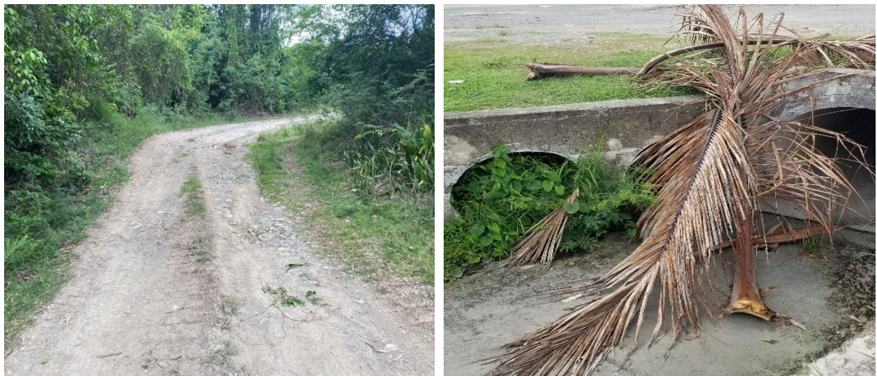
Figure 37. Road erosion (left) and clogged stormwater infrastructure (right).
