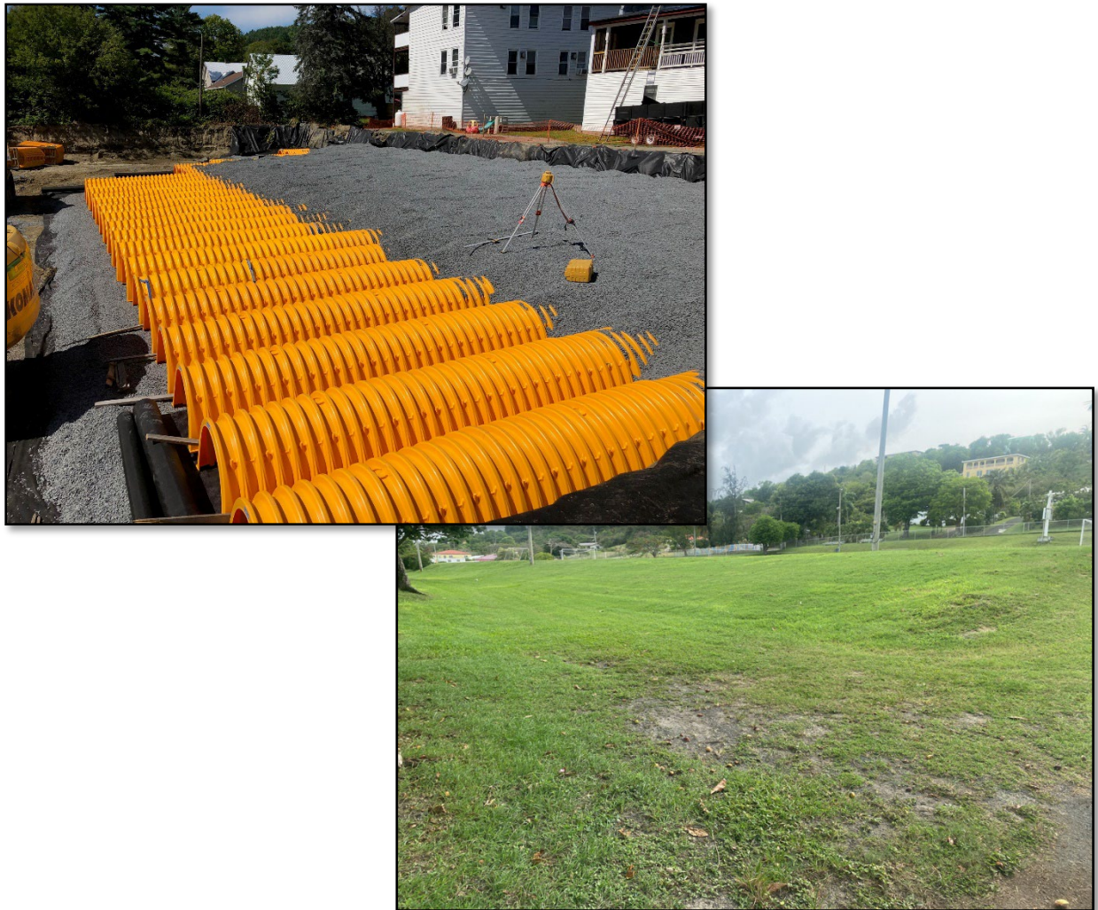
Figure 81. Example photo of subsurface infiltration chambers (above) and recreation field at Freewill Baptist Church (below).
