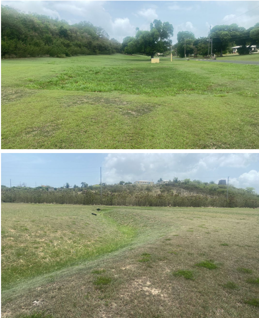
Figure 52. Existing stormwater BMPs in Hovenssa. BMP #6 basin (above) and BMP #1 basin (below).
