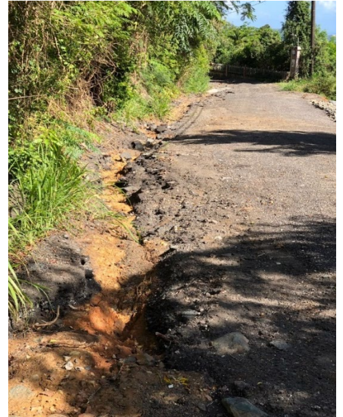
Figure 12. Photo of road erosion taken by resident on a road on the north side of St. Thomas.
