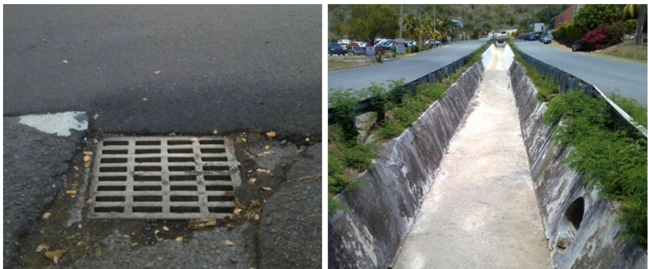
Figure 51. Examples of stormwater infrastructure. A catch basin (left) and a paved swale (right).
