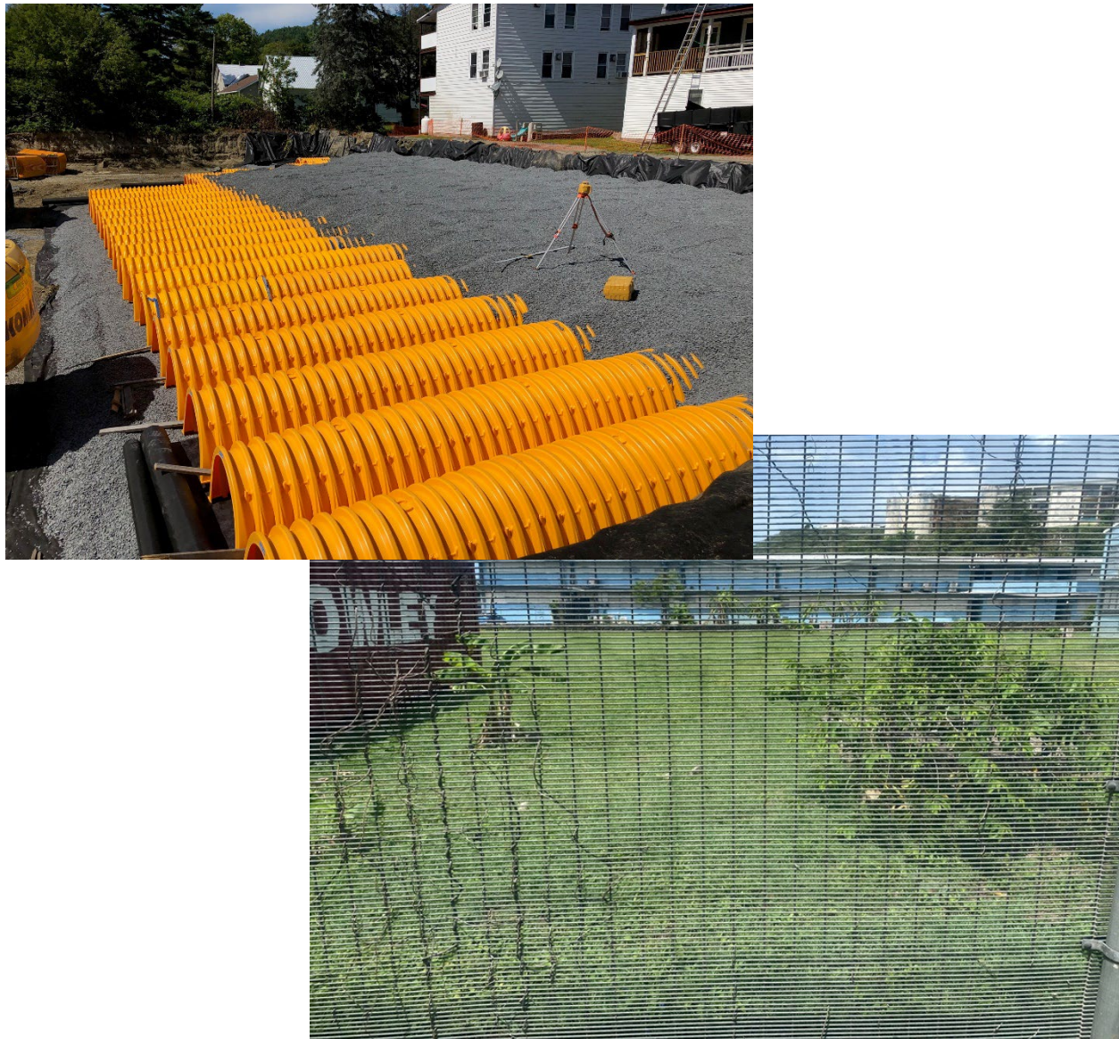
Figure 86. Example photo of subsurface infiltration chambers (above) and Ulla F. Muller Elementary School yard off (below).
