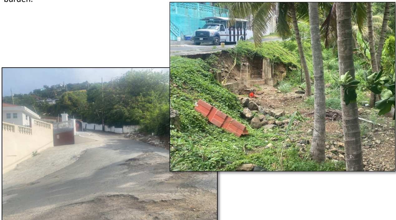
Figure 39. Road erosion (left) and undermined roadway due to unmanaged stormwater (right).
