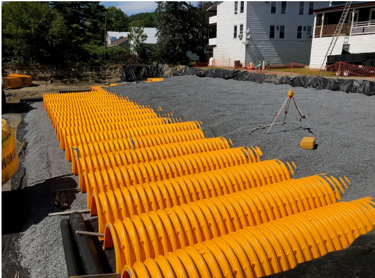
Figure 88. Example photo of subsurface infiltration chambers.
