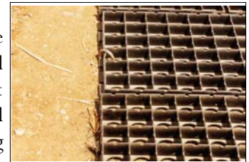
Figure C.13. Geoblock installation close-up, note j-bars used to anchor blocks in place (photo by Dale Morton, 1999).
