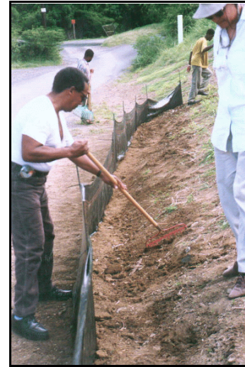
Figure 3.21. Properly installed silt fence (Estate St. George's Hill, St. Croix, 1998).
