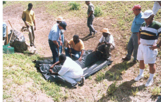
Figure 3.24. Installation of a triangular dike as a check dam in a drainage swale ( Estate St. George’s Hill, St. Croix, 1998 ).
