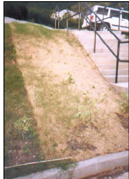
Figure 3.11. Straw mat used to stabilize seeded slope (UVI St. Thomas, 1999).
