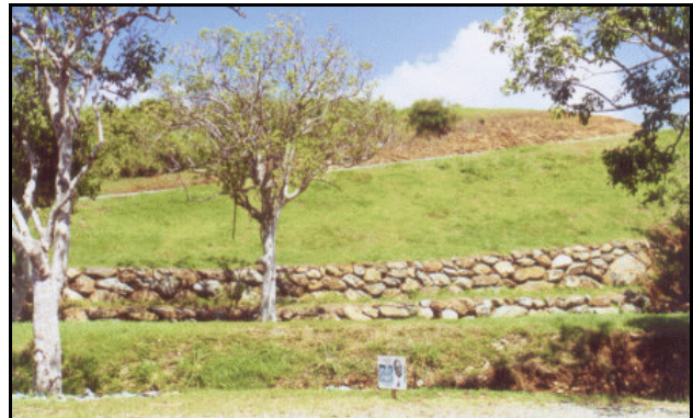
Figure 3.13. Rock retaining walls installed to stabilize base of steep slope above a sediment basin ( Estate New Hernhut, St. Thomas, 2000 ).
