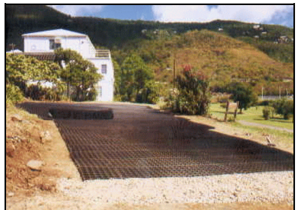
Figure C.12. Geoblock pavement installed at UVI-CES St. Thomas office, prior to filling with soil and seeding (photo by Dale Morton, 1999).
