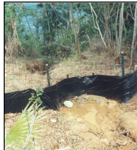
Figure 3.20. Properly installed reinforced silt fence - note trenching, wire mesh and steel bars (Estate Caret Bay, St. Thomas, 1999).
