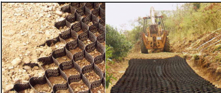
Figure C.14. Close-up of Geoweb® cells being filled with soil (left). Installation of Geoweb® at the UVI-CES St. Thomas driveway (photos by Dale Morton, 1999).
