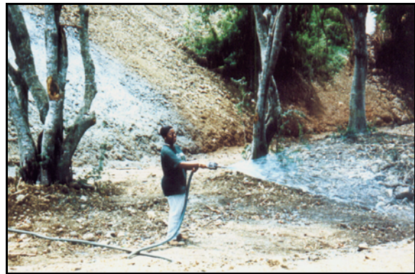
Figure 3.8. Hydroseeding side slopes and outside rim of a sediment basin ( Estate New Hernhut, St. Thomas, 1998 ).
