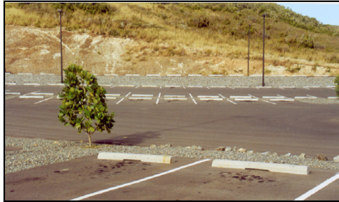
Figure 4.12. Graveled infiltration areas in a parking lot, St. Croix (photo by Dale Morton, UVI-CES).
