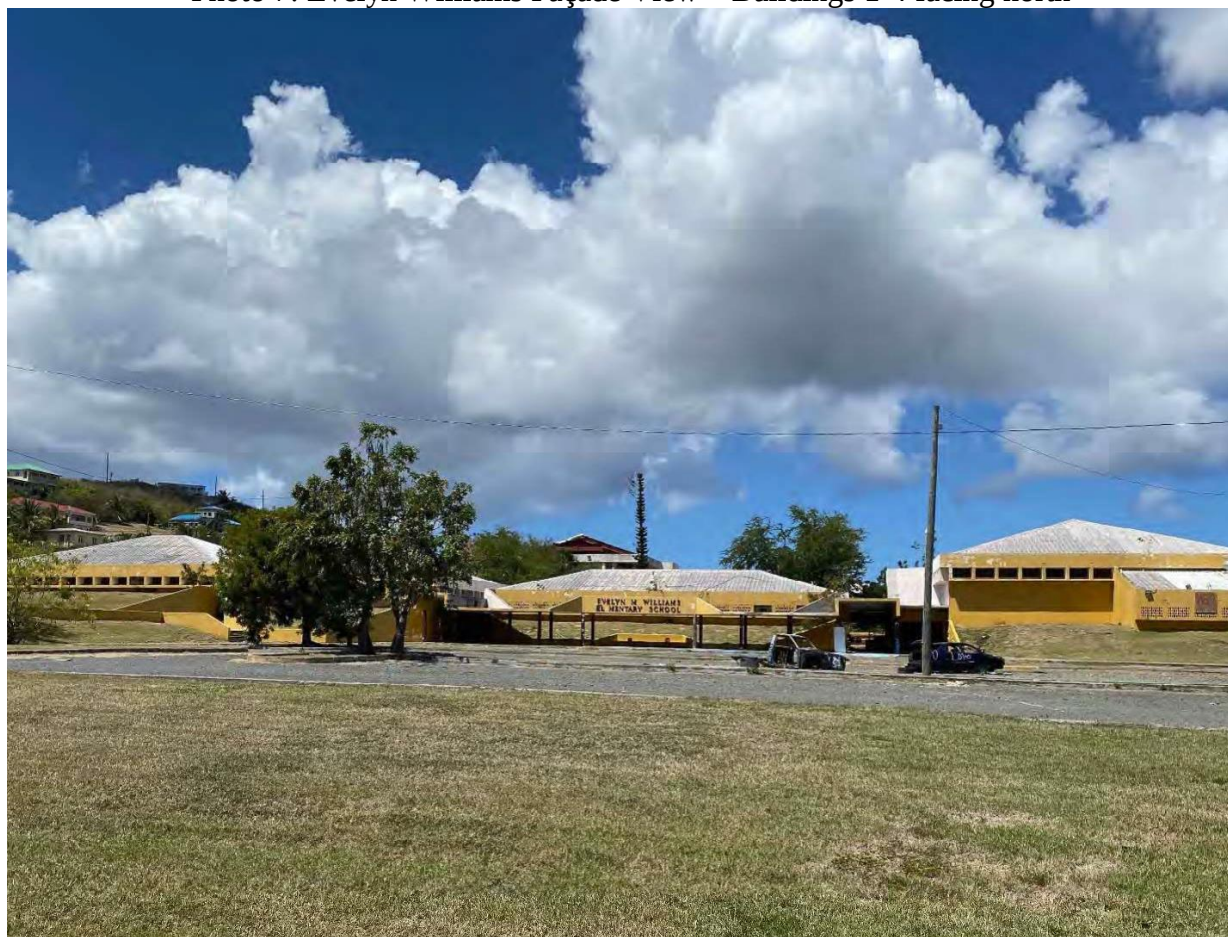
Photo 7: Evelyn Williams Façade View – Buildings 1-4 facing north
