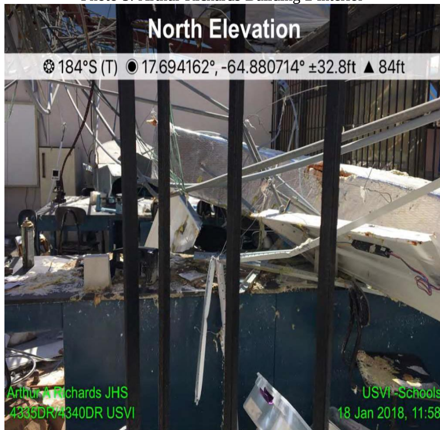
Photo 5: Arthur Richards Building 2 interior
