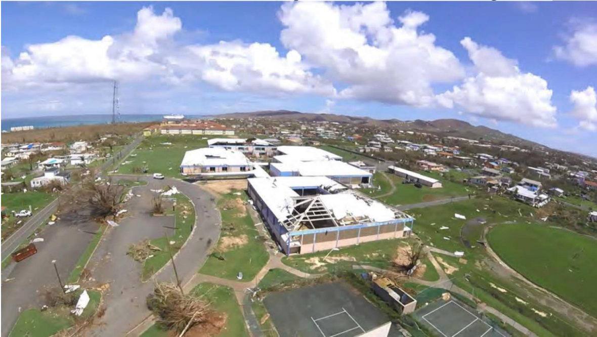
Photo 1: Arthur Richards Junior High School – Aerial View facing north
