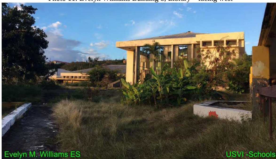
Photo 11: Evelyn Williams Building 8, Library – facing west
