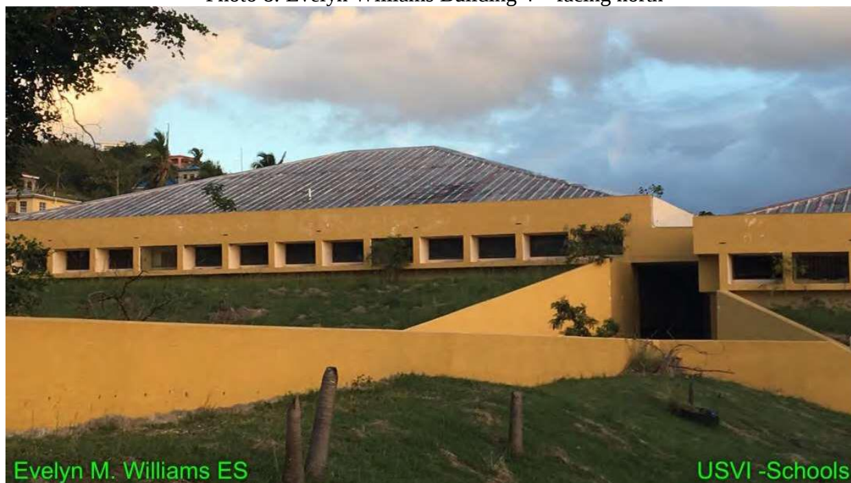
Photo 8: Evelyn Williams Building 4 – facing north
