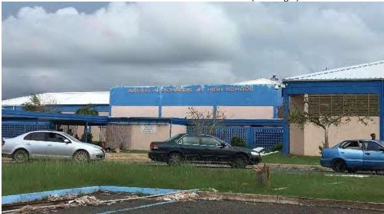
Photo 2: Arthur Richards west elevation (Building 1)
