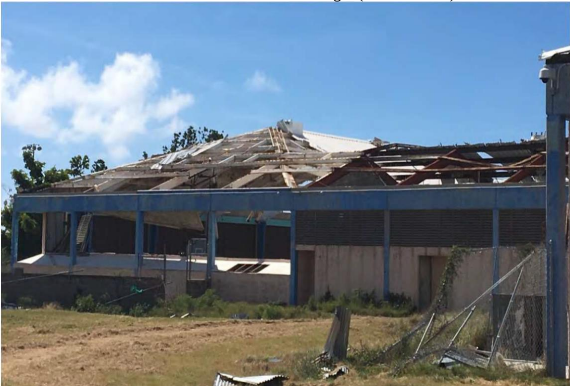
Photo 4: Arthur Richards Building 5 (east elevation)
