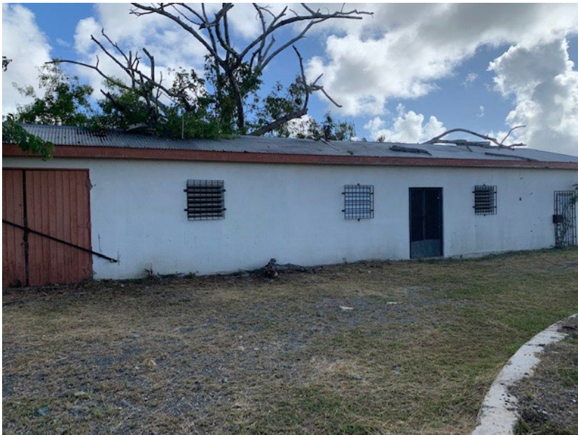
Exhibit 6 – Storage Building (to Remain)
