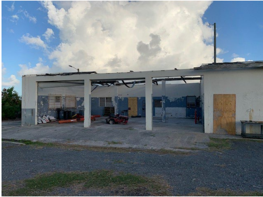
Exhibit 4 – Front of Equipment Storage Bays – Building North View (To be Demolished)
