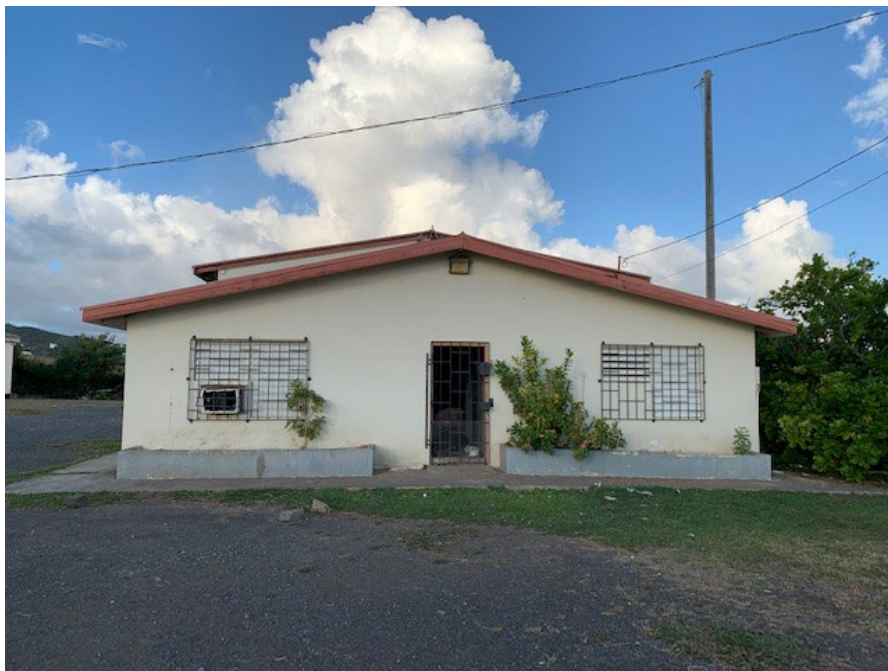
Exhibit 2 – Front of Main Office –Building West View (To be Demolished)
