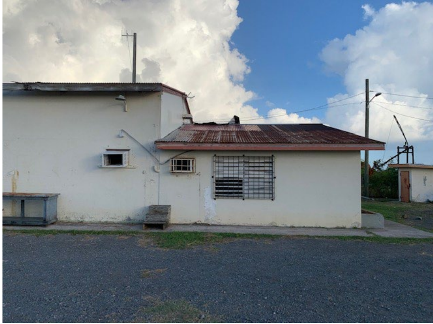
Exhibit 3 – Side of Main Office – Building North View (To be Demolished)
