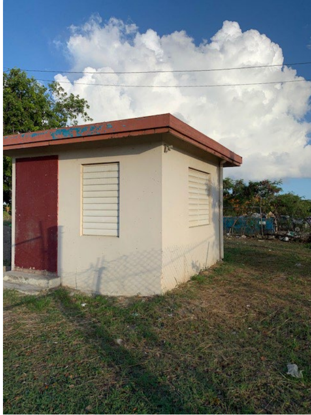
Exhibit 7 – Utility Building No. 1 (To be Demolished)
