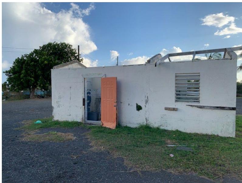
Exhibit 8 – Utility Building No. 2 (To be Demolished)
