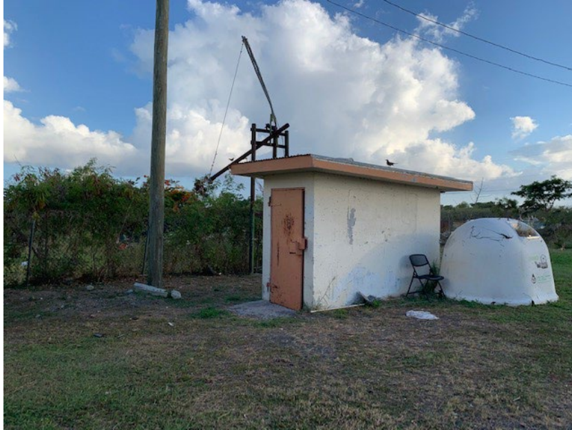
Exhibit 9 – Utility Building No. 3 (To be Demolished)
