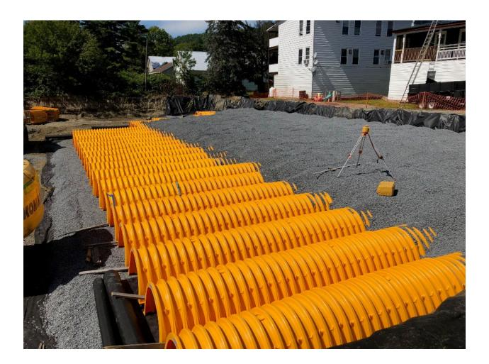
Figure 68. Example photo of subsurface infiltration chambers.
