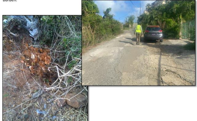
Figure 36. Culvert inlet plugged by sediment (left) and roadway erosion (right).
