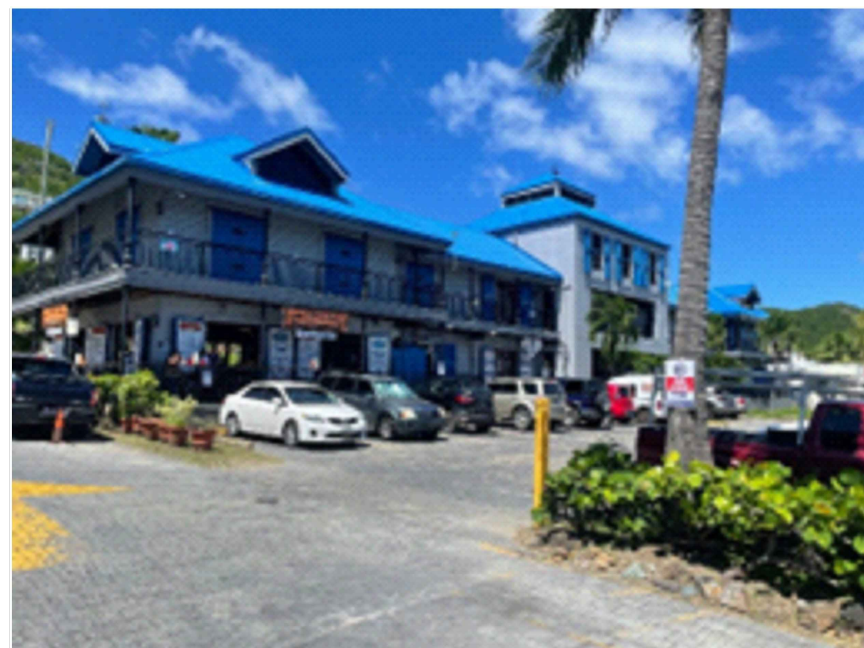
PHOTO 01: VIEW OF SOUTH FACADE - BUILDING A
