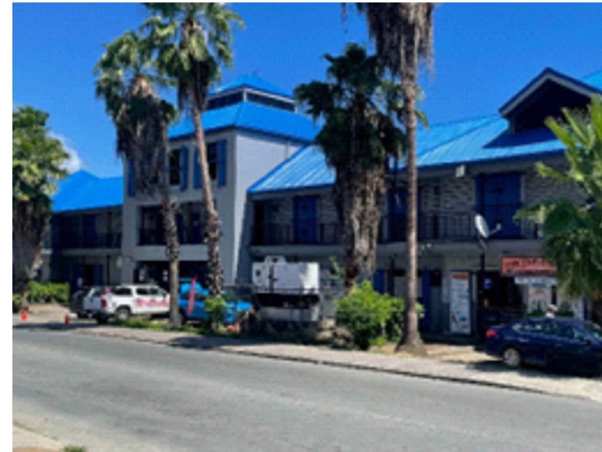
PHOTO 02: VIEW OF NORTH FACADE - BUILDING A
