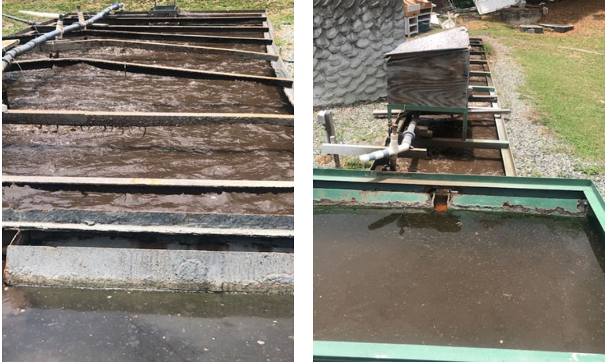
Figure 9-2.- Existing Conditions of WWTP Close-Up
