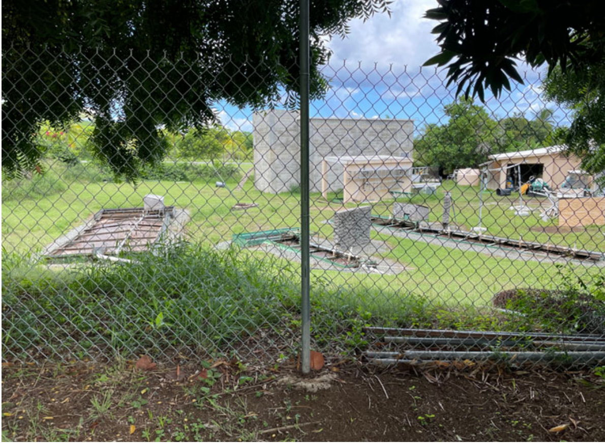
Figure 9-1- Photograph of the Existing WWTP
