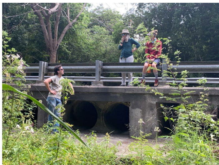
Figure 49. Culverts in the Salt River Bay watershed.
