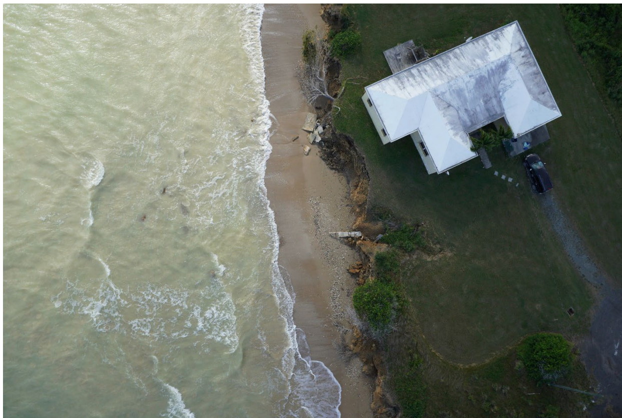
Figure 46. Coastal erosion due to sea level rise threatens stability of homes near the coast.
