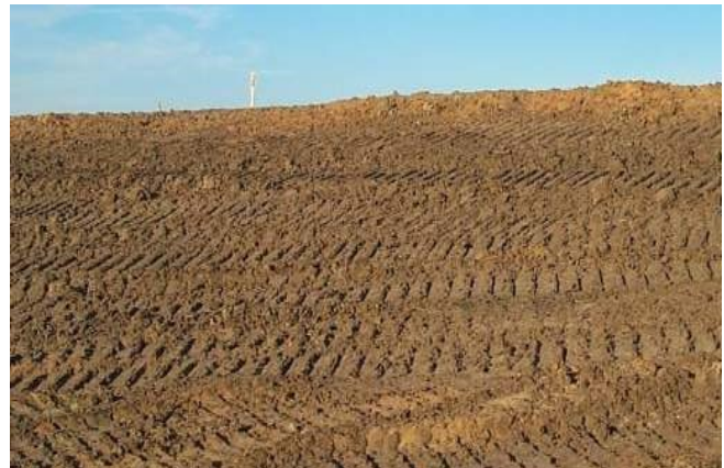
Always roughen surfaces with tracking cleats running parallel to the slope contours (top) rather than perpendicular (bottom) (from Clemson University).
