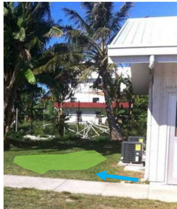
Don't let this clean rooftop runoff go to waste; if there isn't a cistern, direct it to a rain garden or bioretention without needing pretreatment.
