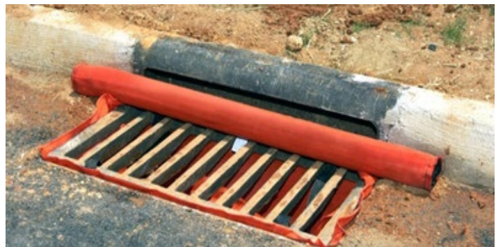
(LEFT) This product is not suited for this type of inlet structure, since "dirty" flows enter drain directly through the grated opening. (RIGHT) An alternative product may be more appropriate.
