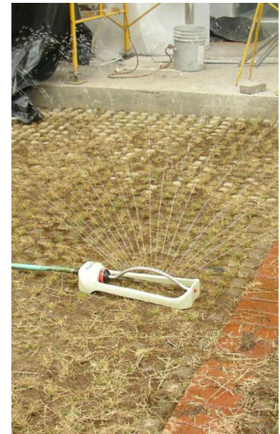
At this installation in American Samoa, soil filled spaces between grass pavers were hollowed out for planting of individual plugs. Using the proper soil mix and providing irrigation helped establish vegetation quickly.
