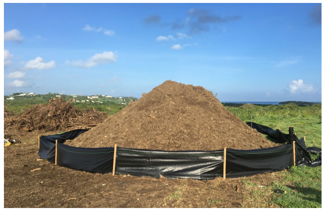
Silt fence or other sediment barrier should be installed around stockpiles.
