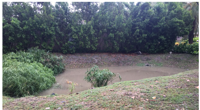
Example of a large basin with outlet structure at St. Croix landfill (top) and a smaller basin with inflow and outflow pipe at a resort on St. Thomas (bottom).
