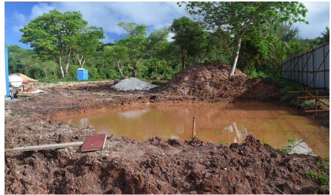
Particulates will settle out of the water column if given enough time. Trapping devices like sediment basins must be sized to manage expected flows and maintained to ensure capacity.
