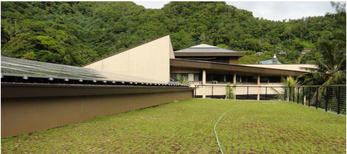
This green roof in American Samoa uses the same grass pavers used in the parking lot which were thought to be heavy enough to stay in place during heavy winds. Installed in conjunction with solar panels, the main function of this green roof is to improve efficiency of the buildings cooling system. This roof now provides a green place for staff to eat lunch.
