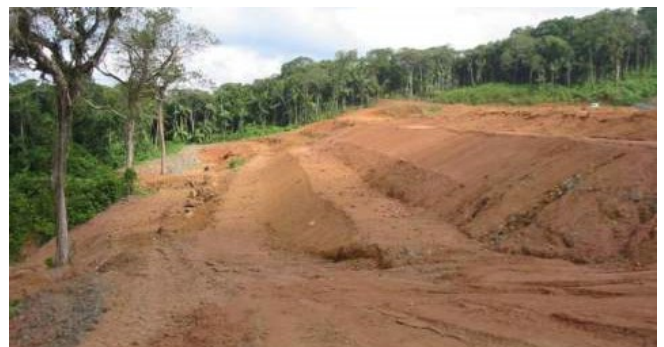
Large-scale benching and terracing prior to planting.
