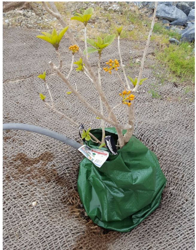
Cordia being planted through jute erosion control blanket on a slope on St. Croix's east end. Consider irrigation needs for plant establishment.
