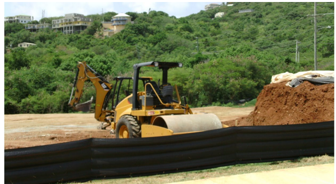
Sediment barriers are perimeter controls used to define the extent of work, protect trees and natural areas from damage, and prevent offsite sedimentation.
