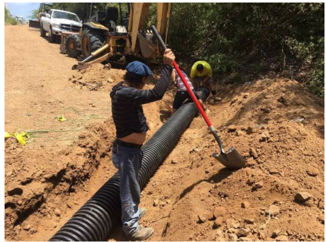
Digging trench for cross drain installation on Culebra, PR. Notice the pipe is laid at a 30–45-degree angle to road to better intercept ditch.
