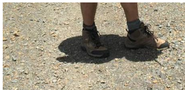
Example of well-graded gravel surface that incorporates fines for better compaction; holds up better to traffic than loose gravel.
