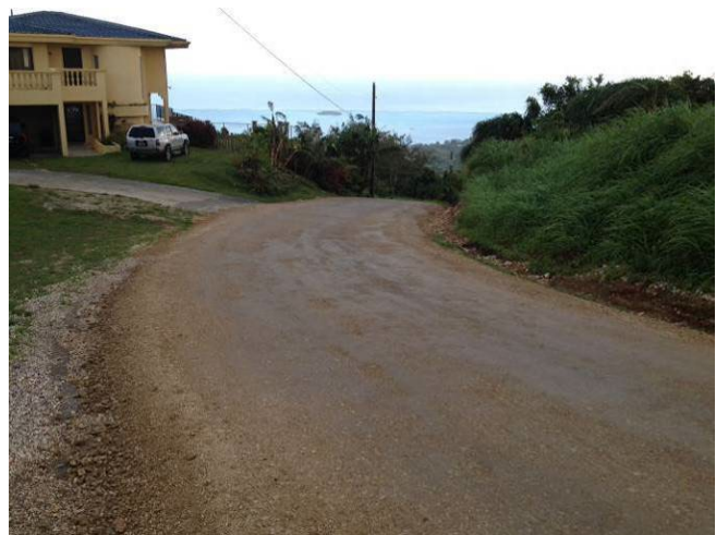
Adding cement-based treatments to the upper layer of soil or aggregate can increase surface longevity for a fraction of the cost of paving.
