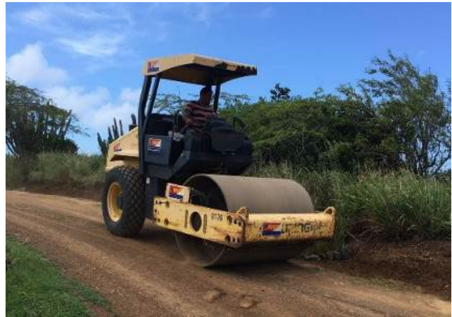
Roller for compacting unpaved road surface (photo credit: Protectores de Cuencas ).
