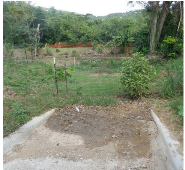
Concrete weir created from old curbing used to create sediment forebay for this bioretention (top); paved concrete flume used as a forebay for a pond in St. John (middle).
