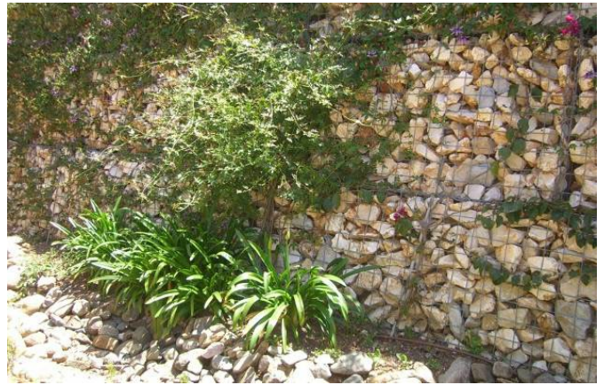
Vegetation may colonize gabion baskets overtime without human intervention.
