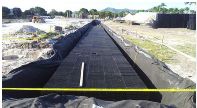
Figure 3.7. The RT Park on St. Croix includes vegetated water quality swales and a large rainwater harvesting system below the parking lot used for irrigation, toilet flushing, and cooling tower recirculation.
