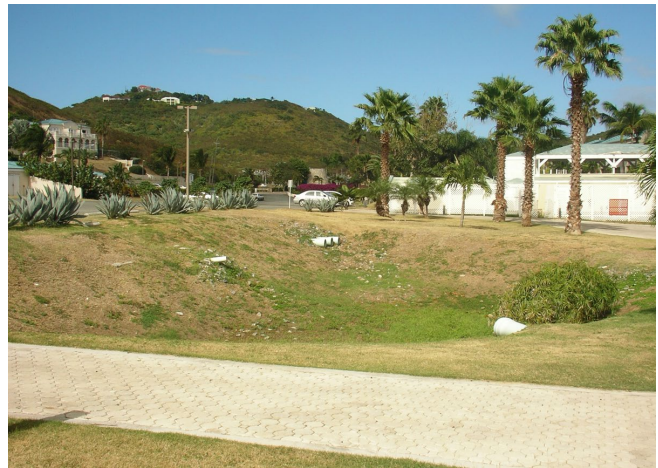
Detention basin at a resort on the east end of St. Croix.
