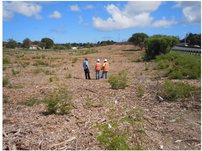
Mulched site material can be spread to temporarily stabilize low slope surfaces.
