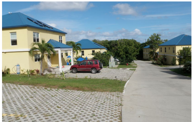
This housing development on St. John used permeable driveways to reduce the amount of runoff volume to be managed downhill.
