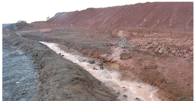
Moving runoff through the site without causing erosion can be a challenge. Limiting drainage area contributions, stabilizing flow paths and slowing velocities are key strategies.
