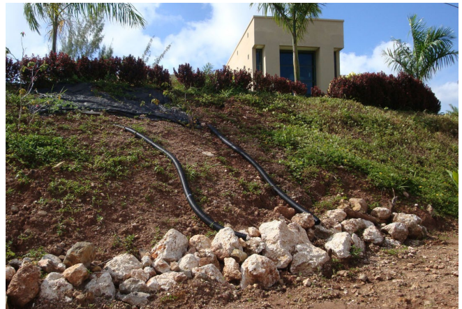
Example of a pipe slope drain used to temporarily convey driveway runoff to stone apron below unvegetated slope.
