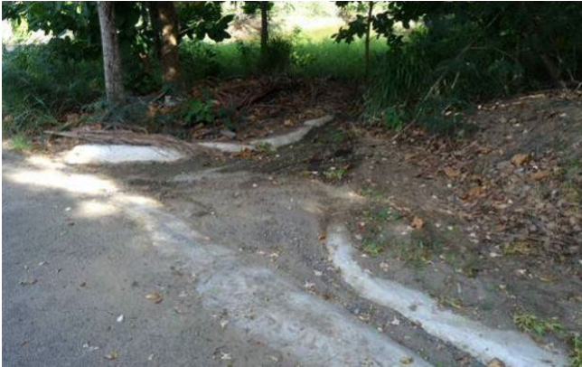
This concrete turnout directs runoff from an unpaved road to a stormwater ponding basin. Sediment deposited in the turnout needs to be removed to ensure continued drainage. Maintenance can easily be conducted with a shovel.
