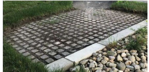
Examples of hardened sediment forebays (with permeable pavers) for easy maintenance that will also drain down after storms.
