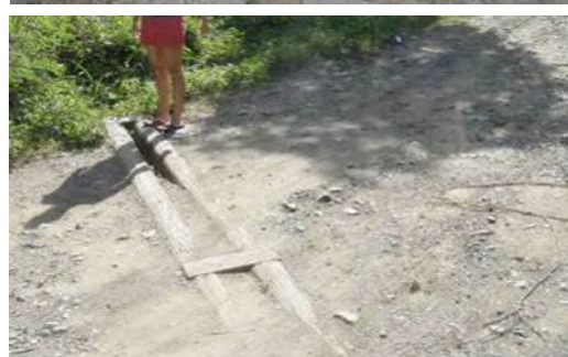
Figure 4.56 Various design alternatives for waterbars. The concrete V-notch and the raised berm & swale options are the most common. Open concrete and timber channels tend to clog quickly. Earthen waterbars are not suitable for highly trafficked roads.
