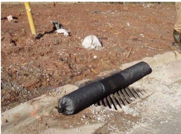
(LEFT) This product is not suited for this type of inlet structure, since "dirty" flows enter drain directly through the grated opening. (RIGHT) An alternative product may be more appropriate.
