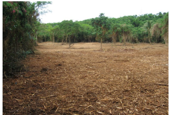
Mulching on site as clearing occurs is standard practice; however, clearing only the area needed for construction (site fingerprinting) and leaving as much natural vegetation in place as possible, is the preferred approach.
