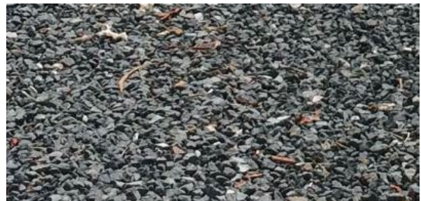
Smaller angular, 3/4" gravel serves as a good void filling component for compacted surface courses and for backfilling check dams.
