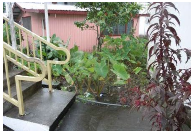
Drainage is directed into a parking median (top) and small taro rain garden between buildings (bottom).
