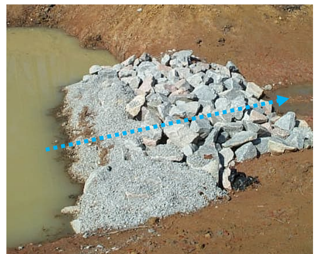
Create a rock filter using smaller sized rock on the inside of rock outlets (Clemson University).
