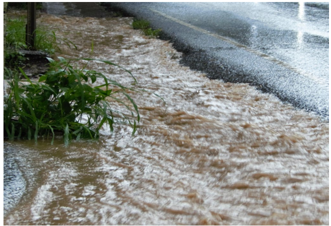
Excessive volume and high velocity runoff conveyed in open channels, pipes, and guts can cause flooding, undermine roads, and lead to other infrastructure damage (photo: Valerie Peters).
