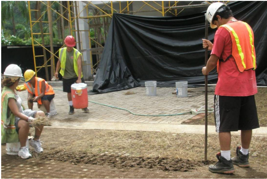
At this installation in American Samoa, soil filled spaces between grass pavers were hollowed out for planting of individual plugs. Using the proper soil mix and providing irrigation helped establish vegetation quickly.
