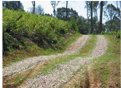
Figure 4.52 Low water crossing with energy dissipator (from FAO Watershed Field Manual).
