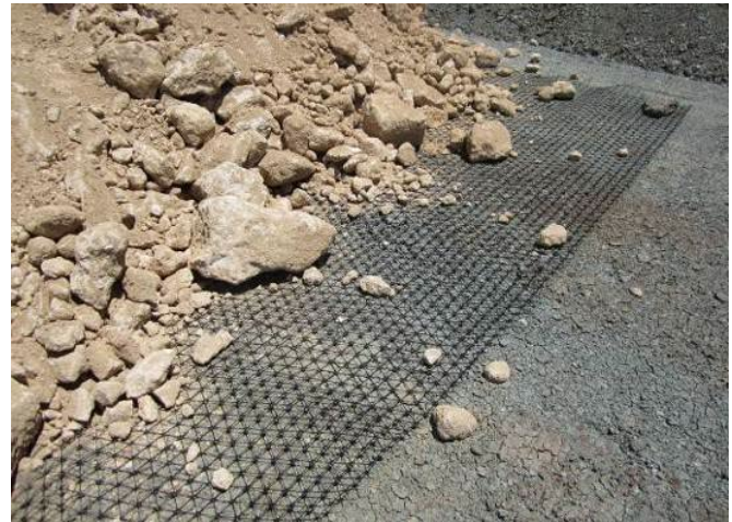
Geoweb installation at Johnnie Horn Rd., St. John (photo: Coral Bay Community Council).
