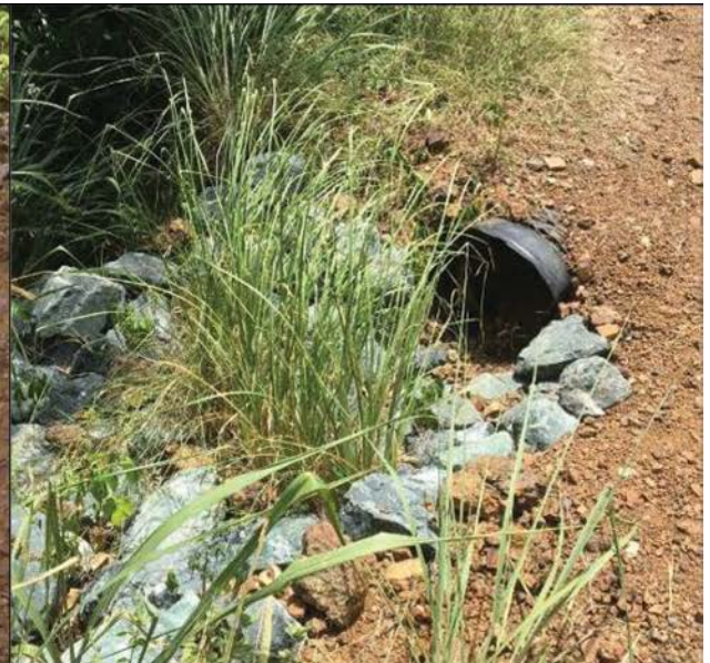
This cross-drain outlet has a stone plunge pool with vetiver grass incorporated into the berm.
