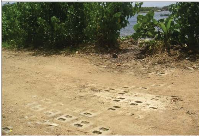
Use of concrete block dip at low point as a cost and more "pervious" alternative to concrete
