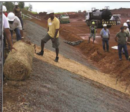
Coir fiber erosion control mat on hydroseeded slope.
