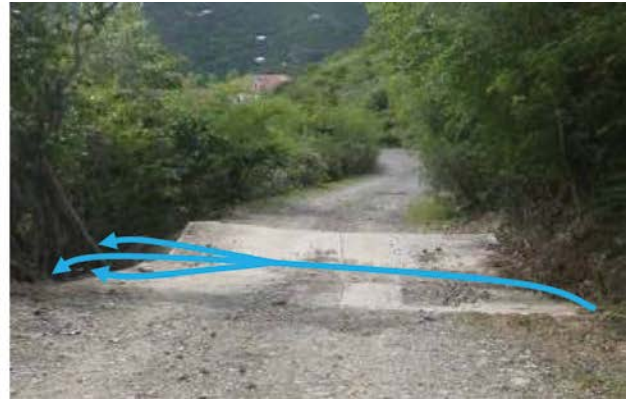
Dip/Low water crossing: broad pad at low point intended to convey and disperse surface flows to an outlet. Sometimes combined with wide berm.
