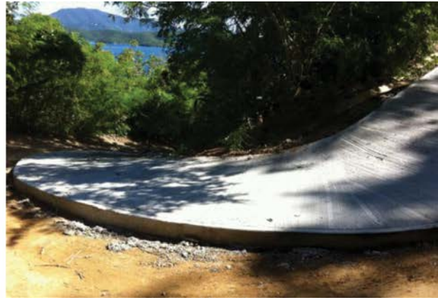
Strategic Paving: Paving sections of road that are highly susceptible to erosion, such as steep inclines and turns.
