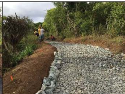
Step 3. Covering geotextile with base course.
