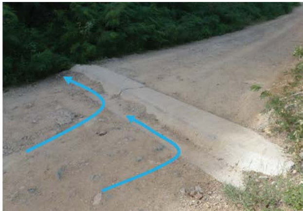
Waterbar: linear berm installed diagonally across travel way designed to intercept flow from the road surface and discharge to stable outlet.
