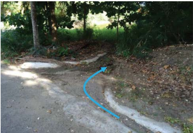
Turnout: designated location where a ditch can discharge and safely disperse flows into vegetated area.
