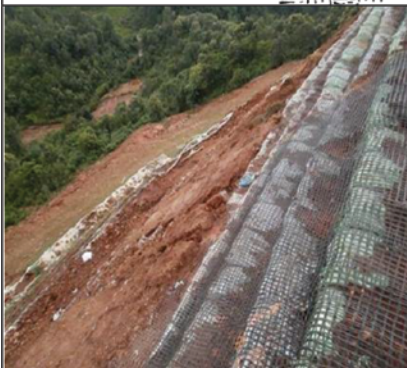
Geogrid layers stacked on a slope.
