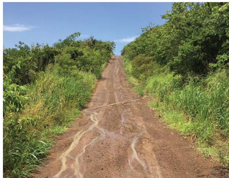
The last place you want concentrated flows is in the travel lane, since this will lead to erosion.
