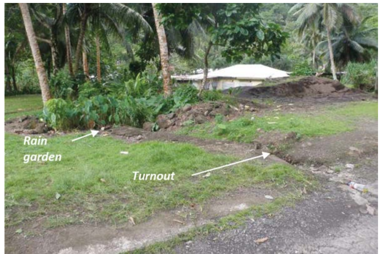
Diverting flows from turnouts into treatment practices such as traps and rain gardens is a good way to filter sediment and reduce runoff volume from roads or driveway tie-ins.
