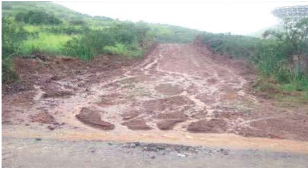
Figure 5. Common Erosion Patterns on Unpaved Road
