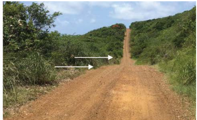
Grade Break: using subtle elevation changes to break up surface drainage areas.
