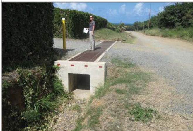
Use headwalls and endwalls (with or without wings) to protect pipe edges from damage and banks from erosion.
