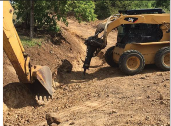
Bedrock can make ditch excavation challenging.
