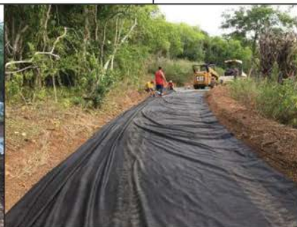
Step 2. Installation of overlapping geotextile fabric.
