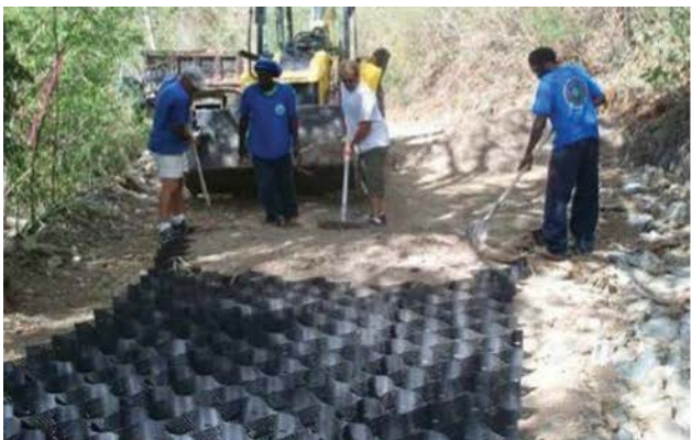
Geosynthetics: grid, mesh, or textile that adds structure to stabilize surface or subbase, distribute vehicular weight, or enhance subsurface drainage.
