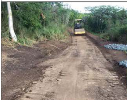
Step 1. Compaction of native subgrade.
