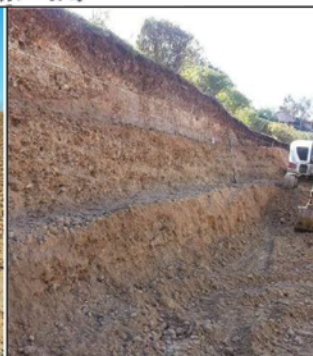
Creating benches on an almost vertical slope.
