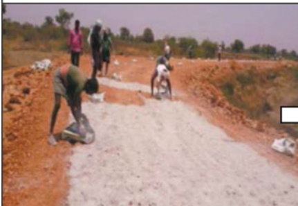
Bags of cement distributed and spread by hand and rake/hand spreader.
