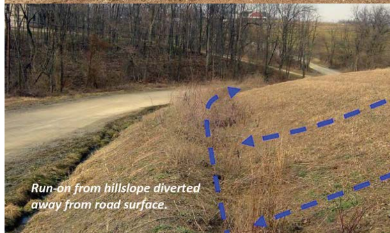
Additional flow coming from the hillside should be intercepted and diverted away from the road surface with a bank bench or interceptor ditch.
