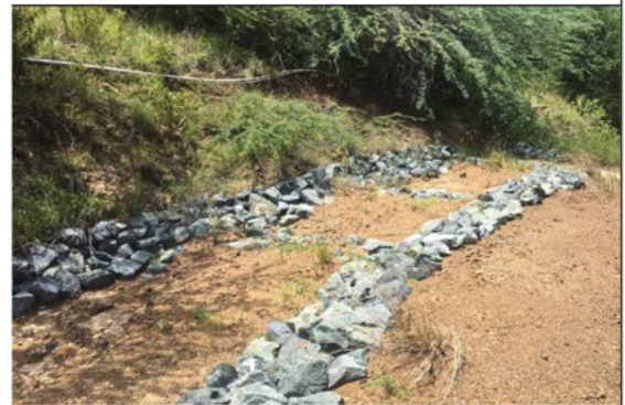
Lined ditch combined with vetiver check dams, full of sediment.
