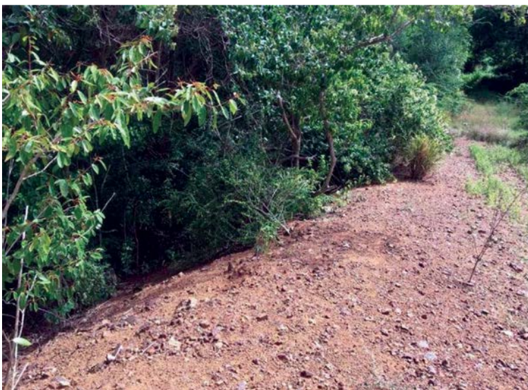
Pre-construction meetings with contractor could help prevent the sidestepping of loose (and erodible) cut material down the outside slope if proper disposal or cut/fill balance is discussed in advance.
