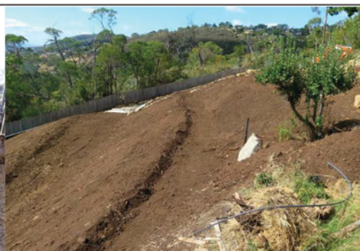
Large scale terracing prior to vegetative planting.
