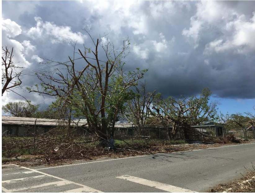
Photo 41: St. Croix Central High School, main façade, primary entrance, looking north:
