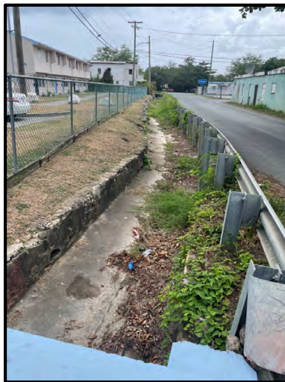
Figure 15: Photograph of rubble masonry storm water Ghut
