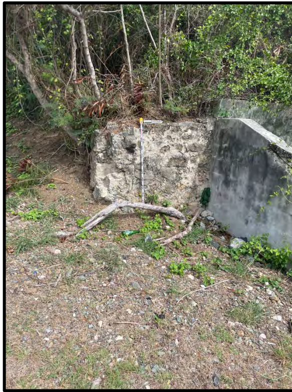
Figure 5: Photograph of a rubble masonry wall and concrete retaining wall.
