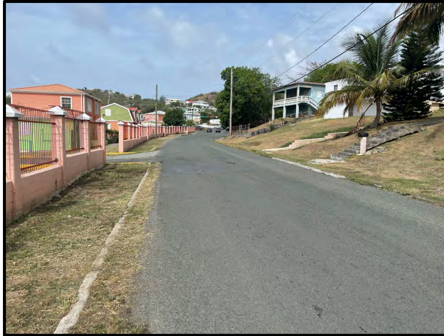
Figure 13: Photograph of Soboetker Lane depicting the cut slopes on its west side and the narrow grassy area on its east side that has been stripped of topsoil and compacted
