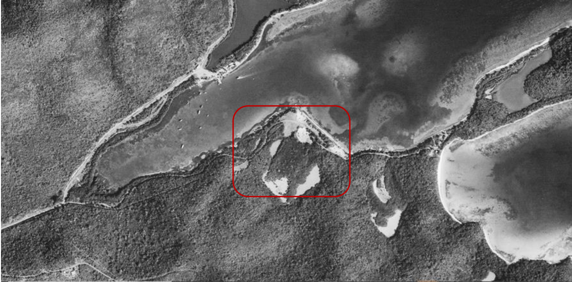
Figure 6.08.1 There were wetlands throughout the site in 1954.
