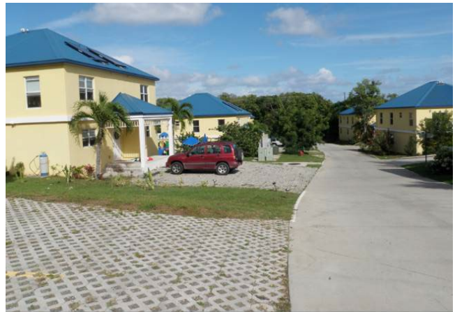
Cisterns and permeable pavers are techniques that can be used to reduce runoff volumes on site.
