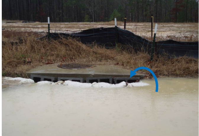
Impermeable sandbags used to protect inlets can lead to localized flooding if the weir elevations are too high or placement prevents any spillover. (Left) Sandbag elevation is lower than roadway and sediment is trapped in paved ditch. (Right) Sandbags do not block curb inlet allowing for passage of high flows into the drainpipe.
