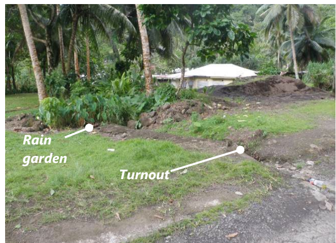
Example of a turnout taking road runoff into a raingarden.
