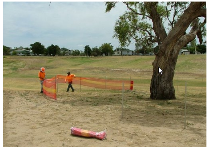
Bright orange construction fencing used for tree protection should be protective of trunk and roots.
