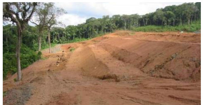
Large-scale benching and terracing prior to planting.
