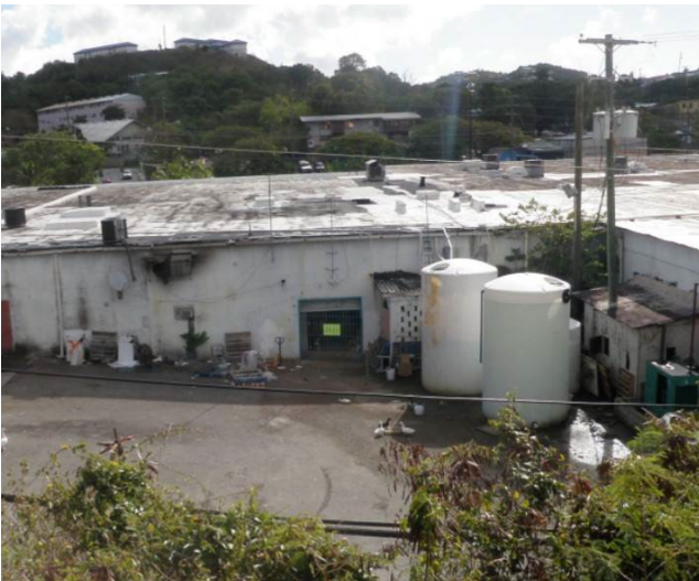
Assuming that rooftop runoff collected in cisterns is "clean" may not always be true, as is illustrated here behind a retail center on St. Thomas.
