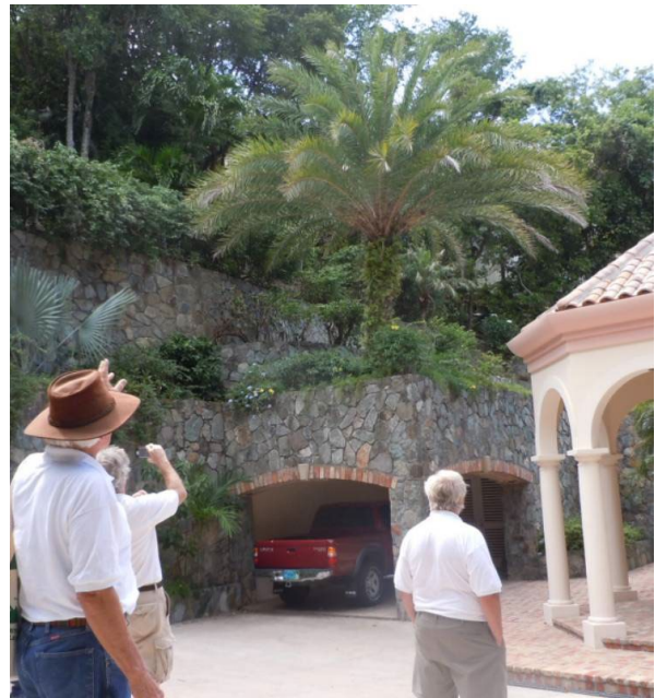
This green roof over a residential garage on St. John shows that large vegetation can be supported if designed and maintained properly.
