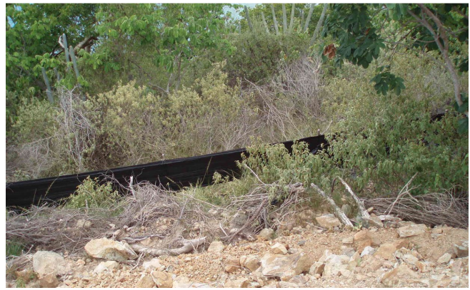
Silt fence is the most common sediment barrier and perimeter control, but also the most difficult to install and maintain over time.
