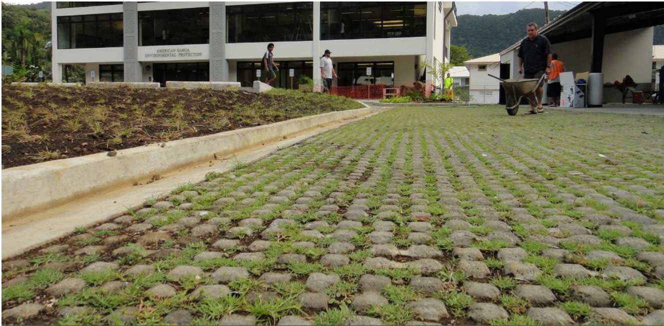
Grass pavers installed at the new American Samoa Environmental Protection Agency office, one of the first LEED-certified buildings in the South Pacific. (photo: Brian Rippy)
