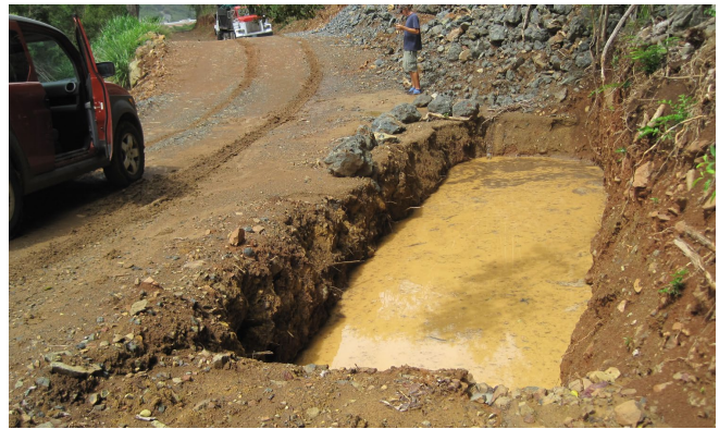
A sediment trap collects runoff from a construction site on St. Thomas East End. .
