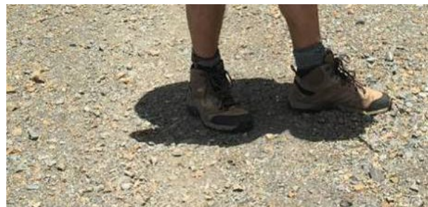
Example of well-graded gravel surface that incorporates fines for better compaction; holds up better to traffic than loose gravel.
