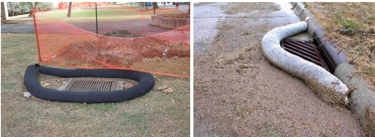
Figure 4.37 Several drain and curbside options for using filter socks for inlet protection (from Filtrexx)
