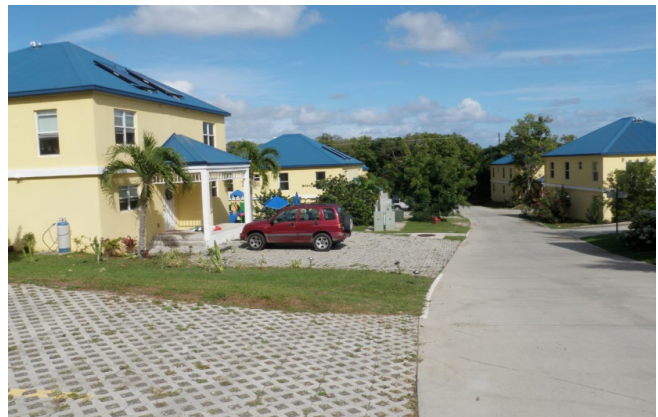
This housing development on St. John used permeable driveways to reduce the amount of runoff volume to be managed downhill.
