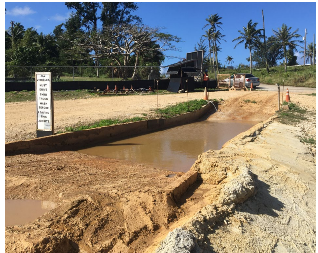
Washing tires of construction vehicles can be a good way to prevent sediment from leaving the site. Tire washes should be designed to manage muddy water.
