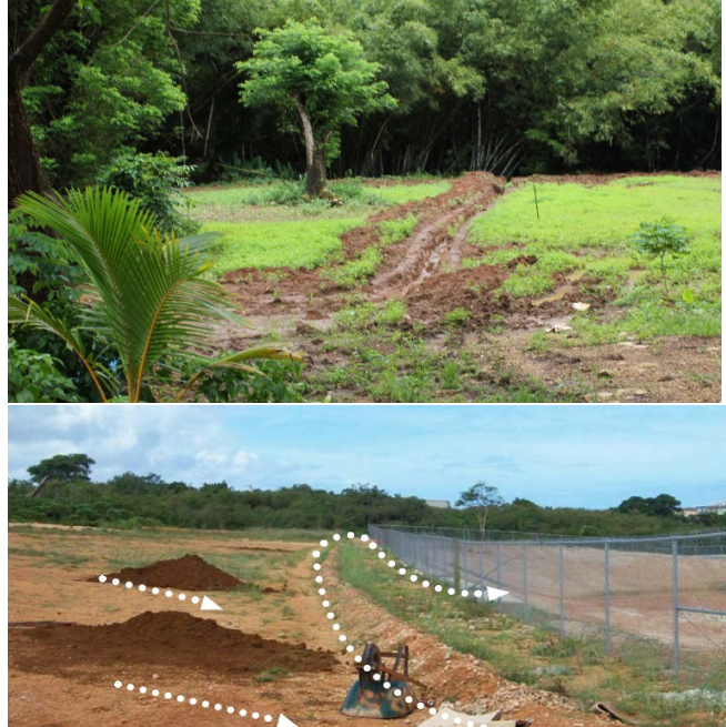
(Top) Diversion swale used to convey off site flows away from construction activity. (Bottom) Berm constructed at the perimeter of sediment basin to convey flows to a stabilized inlet into the basin (Guam EPA). White arrows indicate intended flow paths.
