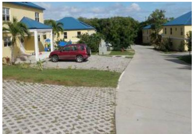
Concrete grid pavers used at multi-family housing complex on St. John.
