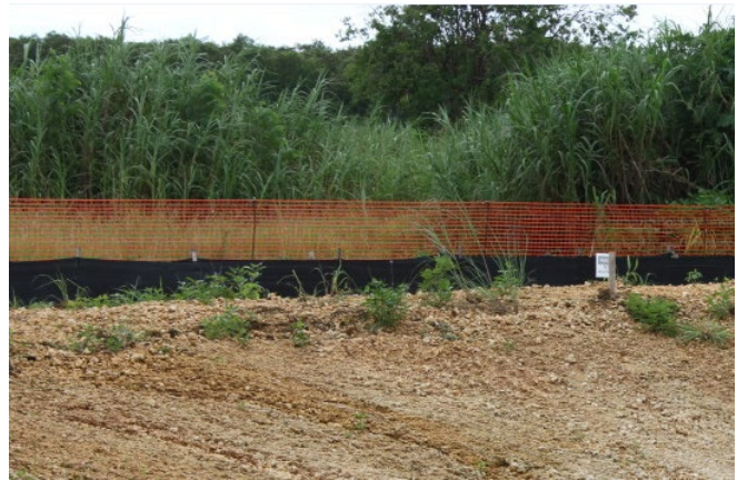
Orange safety fencing denoting the limit of disturbance.
