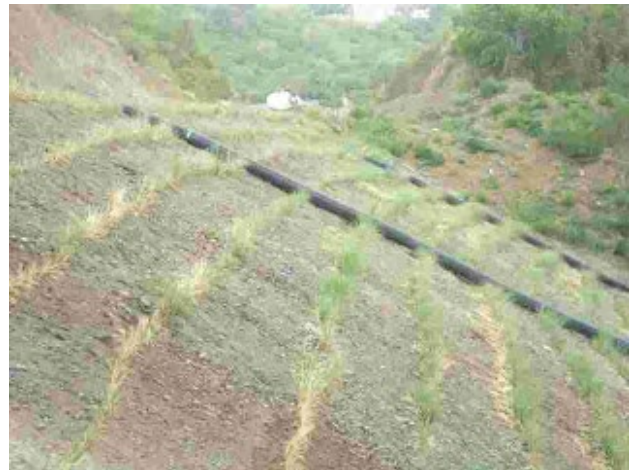
Hydroseeding can be used very cost-effectively for temporary or permanent stabilization of steep slopes (top) and flat terrain (from Protectores de Cuencas). Vetiver plugs and pipe slope drains can be used in combination with hydroseeding to improve stabilization success (bottom).
