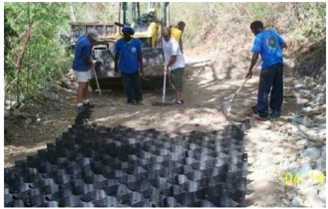
Geoweb installation at Johnnie Horn Rd., St. John (photo: Coral Bay Community Council).
