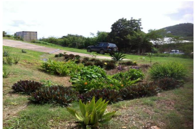
Vegetated filters like rain gardens can be integrated into the landscape and used to clean runoff before it is discharged off site.
