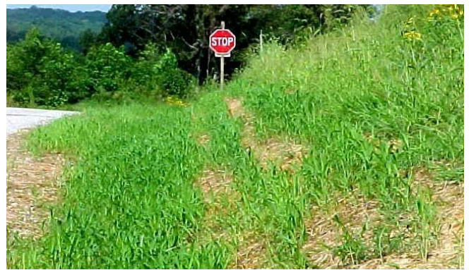
Stair steps used to help establish grass to stabilizing a hillside (photo: Clemson University).
