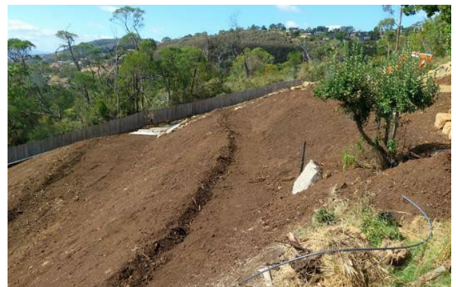
Stair steps used to help establish grass to stabilizing a hillside (photo: Clemson University).
