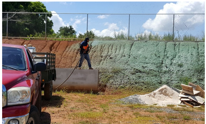
Erosion gullies on an exposed steep slope are being stabilized with vegetation through hydroseeding (photo credit: Protectores de Cuencas).
