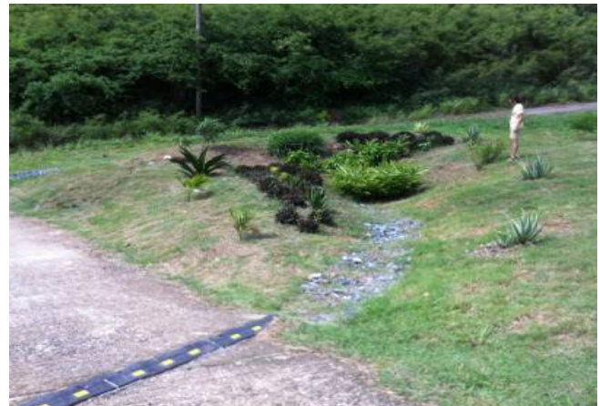
This rain garden in the Hope and Carton neighborhood on the east end of St. Croix intercepts driveway runoff before discharging onto the community's unpaved road.
