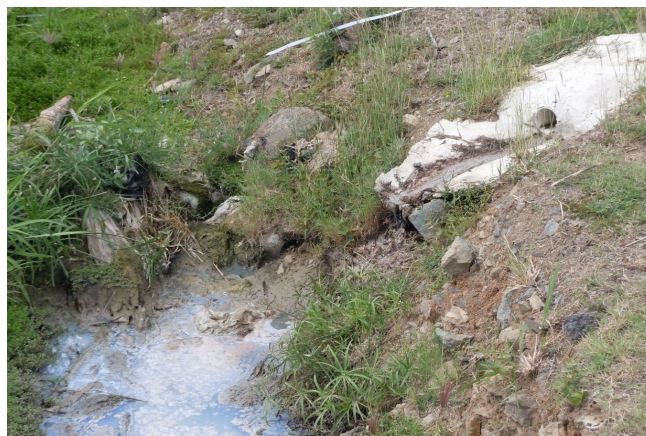
Illicit discharges include non-stormwater discharges (dry weather flow) such as those from leaking septic systems and dry cleaners.
