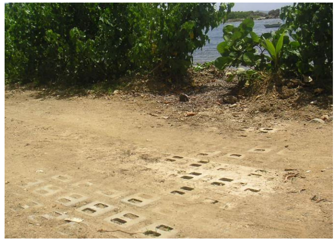
Examples of reinforced dips (from top left to bottom right) made from concrete, concrete with embedded stones for better traction, stone/rock pad that conveys flows to a sediment trap, and drainable concrete blocks.
