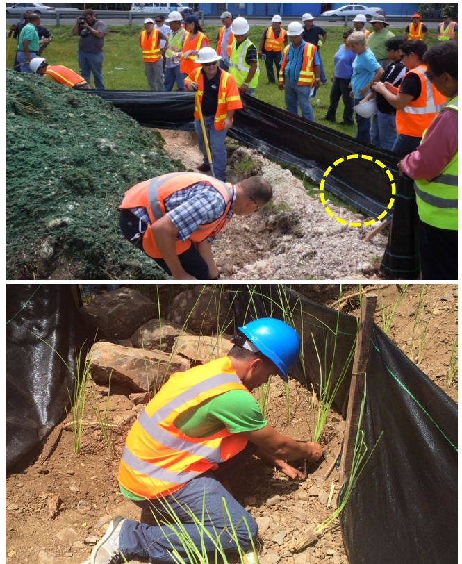
Figure 4.8 Proper silt fence installation requires 6-inch-deep trenching making it difficult to install. Most fencing comes with a line printed on the fabric indicating depth of burial.
