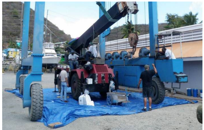
Pollution prevention measures, such as protecting the ground from hydraulic fluids at boatyards, covering dumpsters, or providing secondary containment are an ongoing operational requirement.
