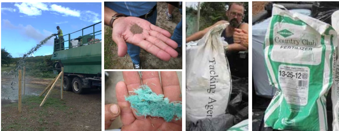
Hydroseeding at Green Cay, STX. Hydroseed mix includes seed, mulch, tackifier, and sometimes fertilizer (source: Protectores de Cuencas).
