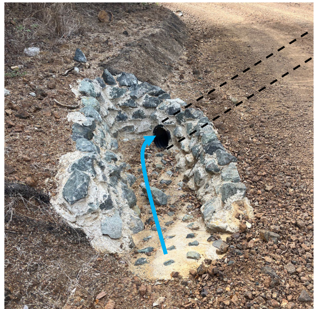
Grouted rock headwall around this cross-drain inlet serves as a ditch block and stabilizes inlet point.
