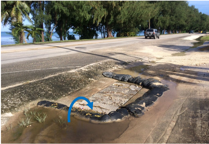
Impermeable sandbags used to protect inlets can lead to localized flooding if the weir elevations are too high or placement prevents any spillover. (Left) Sandbag elevation is lower than roadway and sediment is trapped in paved ditch. (Right) Sandbags do not block curb inlet allowing for passage of high flows into the drainpipe.
