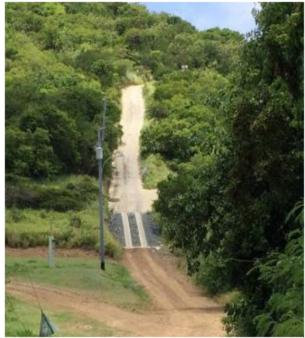
Roads on steep slopes should be paved or stabilized with an aggregate surface (no loose sediment). Note that this road demonstrates paving at the steep section, gravel at mid-slope, and native material where flat.
