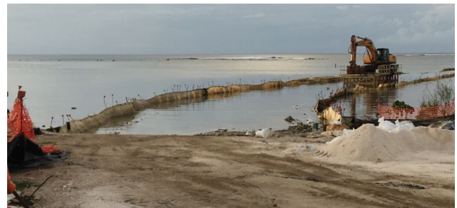
Do not use silt fence in lieu of a turbidity curtain for in-water construction activities.
