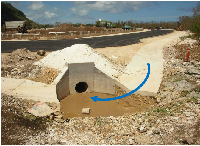
(LEFT) No inlet protection measures installed allows sediments and construction debris to enter drainage pipes prior to site stabilization. (RIGHT) A creative use of temporary wire mesh and geotextile for inlet protection.
