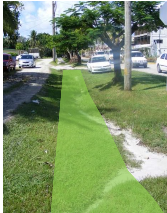
Road rights-of-way are good places to install dry swales to help clean and infiltrate road runoff.
