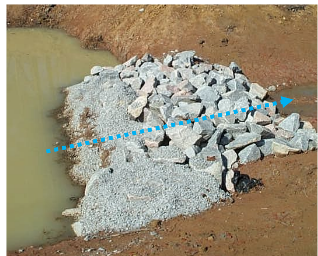
Create a rock filter using smaller sized rock on the inside of rock outlets (Clemson University).
