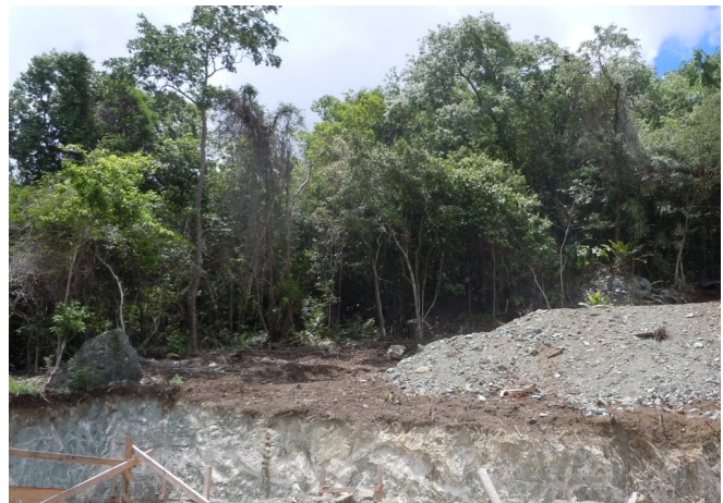
Without a visible demarcation of limits of disturbance, site clearing can unintentionally occur beyond the approved boundary.
