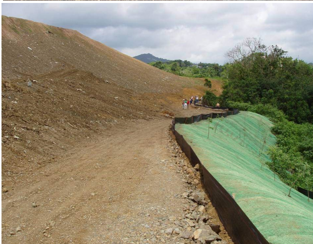
(Top) Installation of straw filled ECB lengthwise down a side slope. (Bottom) Example of a stabilized and unstabilized slope. Lower slope has erosion control blankets with green plastic mesh to protect steep slopes while vegetation becomes established. Think carefully about using plastic as it is not ideal for animals and is relatively permanent.
