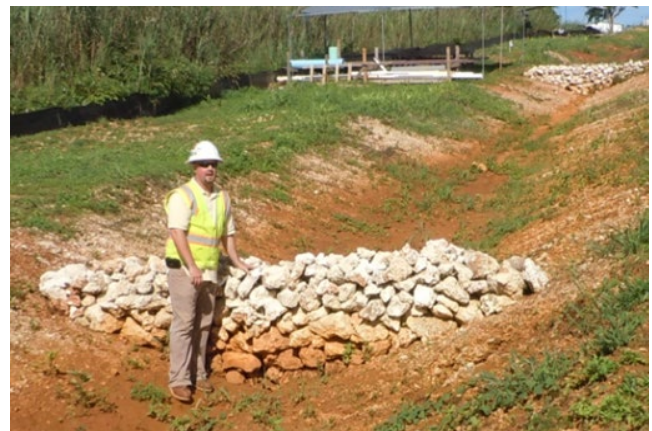
(Top) Series of small check dams correctly "smiling" in a drainage channel. (Bottom) Check dams with a crest elevation equal to side elevations (not smiling) has the potential to create runaround.
