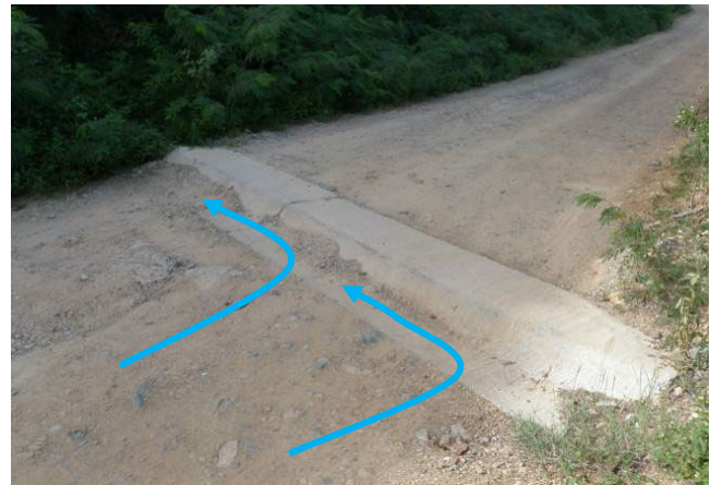
Waterbars are a combination of a raised berm and swale extending the full width of the road. They intercept and direct surface flows to a stabilized turnout.
