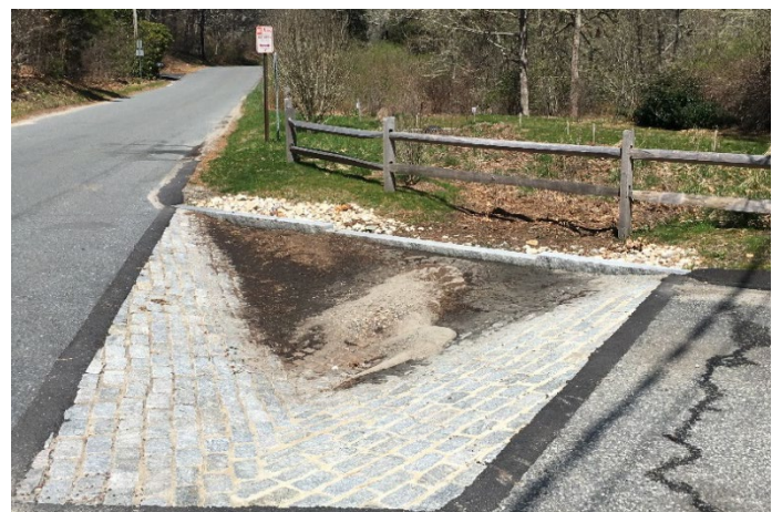
Use a shovel to sediment and debris from the forebay.
