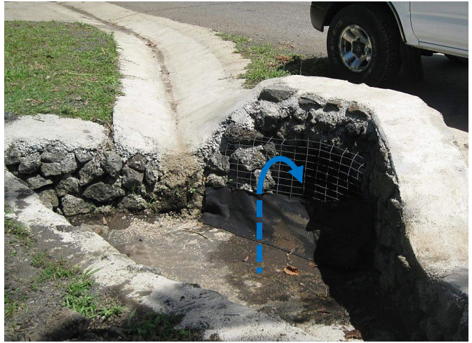
(LEFT) No inlet protection measures installed allows sediments and construction debris to enter drainage pipes prior to site stabilization. (RIGHT) A creative use of temporary wire mesh and geotextile for inlet protection.
