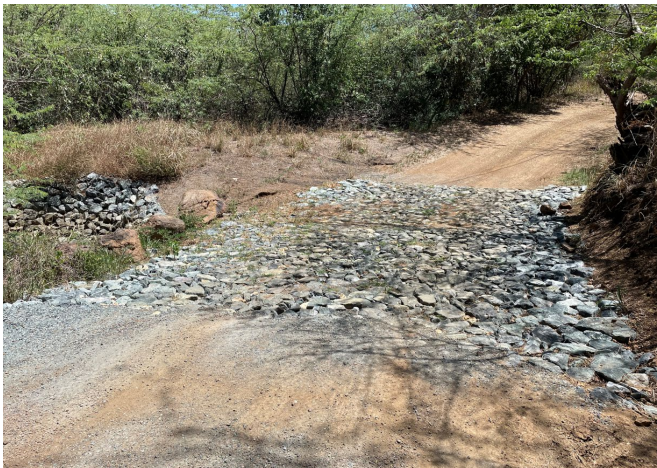
Examples of reinforced dips (from top left to bottom right) made from concrete, concrete with embedded stones for better traction, stone/rock pad that conveys flows to a sediment trap, and drainable concrete blocks.
