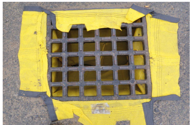
Figure 4.36 Silt Sack™ Catchbasin Protection Detail
