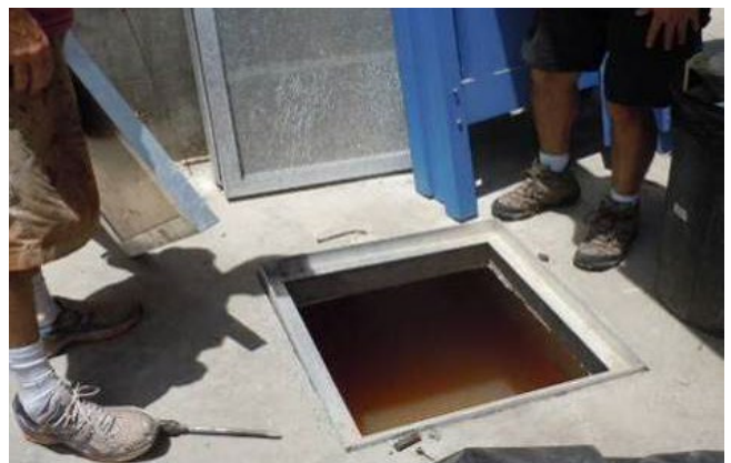
Cisterns and tanks are commonly used in the VI for rainwater harvesting.
