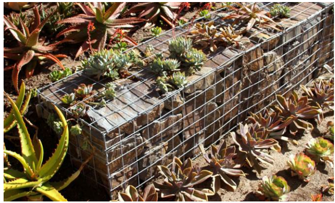
Living walls and bioengineered systems combine structural elements with plants for enhanced slope protection and long-term aesthetics (Gardendrum.com).
