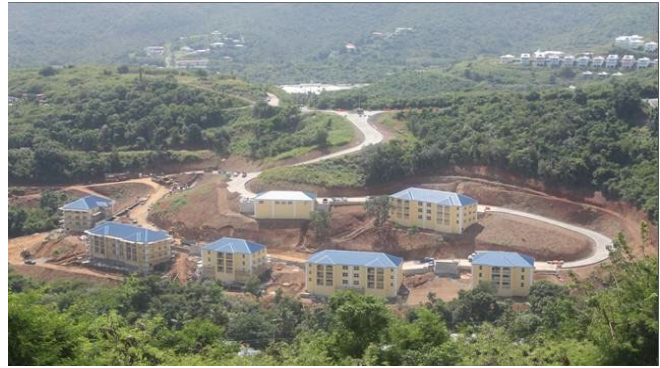
The extent of exposed soils at this steep-sloped construction site on St. Thomas illustrates why proper use of ESC measures is important for protecting downstream resources.
