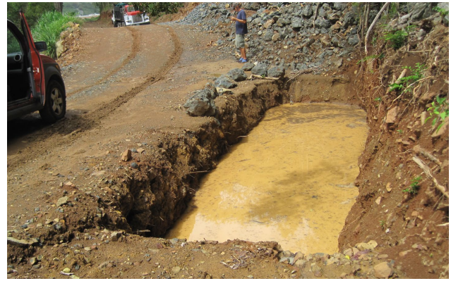
Sediment trap excavated along a construction access road on the east end of St. Thomas.
