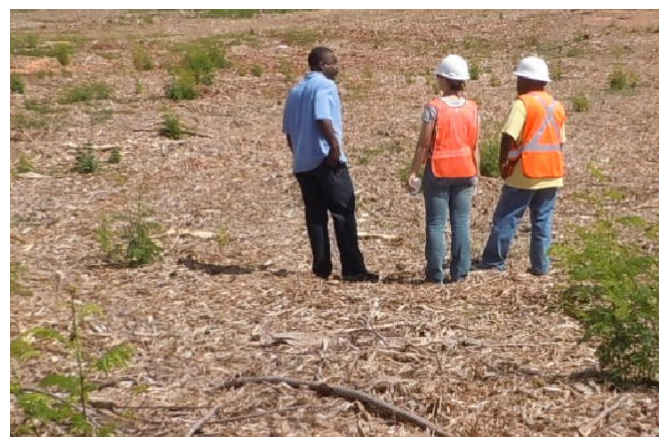
Chipped wood generated during site clearing for a solar farm on St. Croix was spread at this site to cover exposed soils to prevent erosion.
