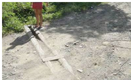
Figure 4.56 Various design alternatives for waterbars. The concrete V-notch and the raised berm & swale options are the most common. Open concrete and timber channels tend to clog quickly. Earthen waterbars are not suitable for highly trafficked roads.
