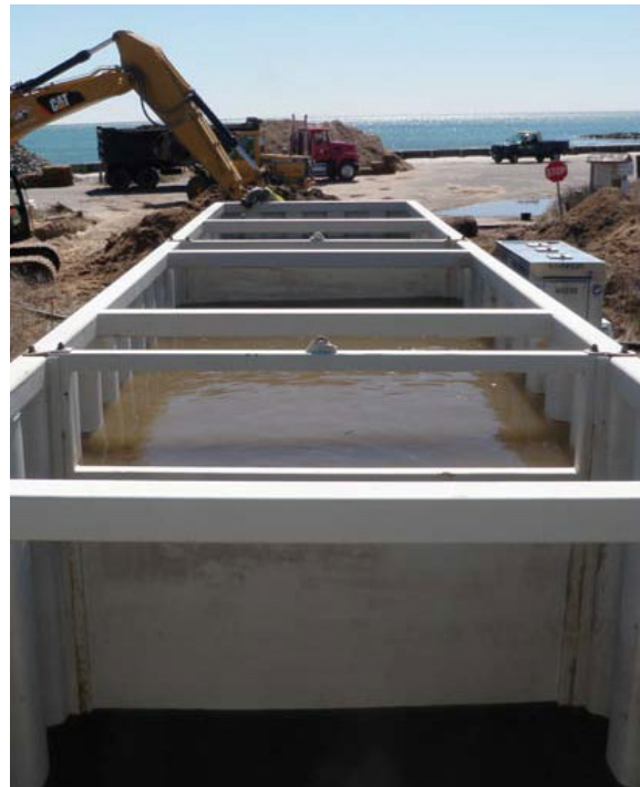
Weir tanks are divided into compartments by baffles or weir walls that trap sediment. The longer the residence time provided, the cleaner the discharge water will be.
