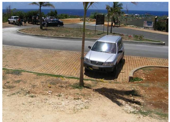
Protect permeable pavements from sediment-laden run-on, particularly from erodible areas where vegetation has not yet established.
