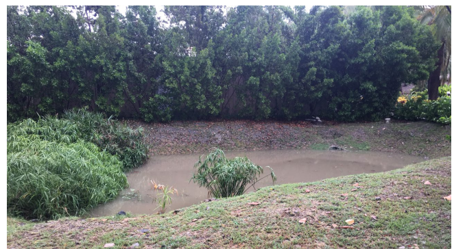
Example of a large basin with outlet structure at St. Croix landfill (top) and a smaller basin with inflow and outflow pipe at a resort on St. Thomas (bottom).
