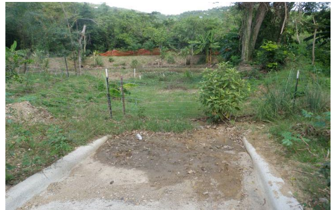
This sediment forebay to a detention pond in Coral Bay will require ongoing maintenance to remove accumulated sediment for the basin to properly function.
