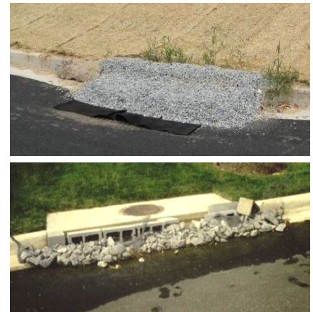
Figure 4.40 Schematic drawing of rock curb inlet protection and examples of using concrete blocks for curbside inlets. .
