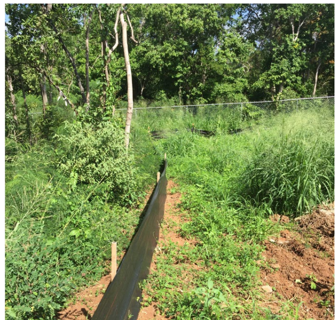
Silt fence or other sediment barrier should be installed around stockpiles.
