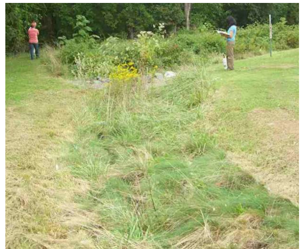
A pretreatment grass channel leading from parking lot to bioretention.
