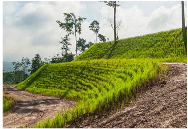
Vetiver grass planted in tight rows can stabilize an exposed slope.
