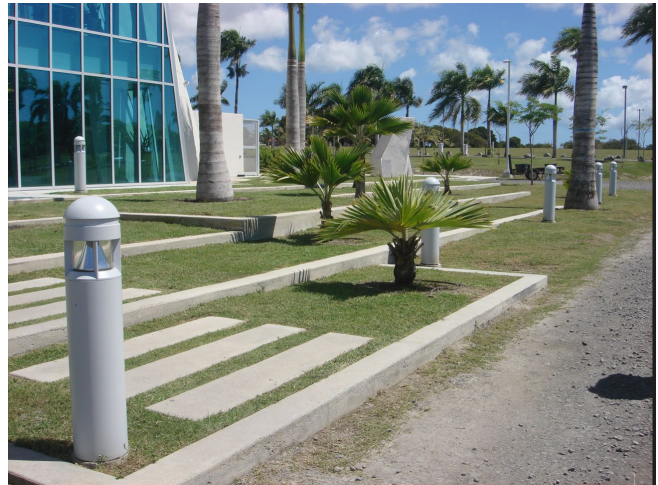
Swap out hot pavement for cooler grass in areas where pedestrians walk. Smaller areas of impervious can drain to pervious areas for runoff reduction.
