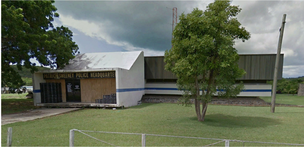
Photo 1 – Front View of Administrative Office Site – Looking Southwest
