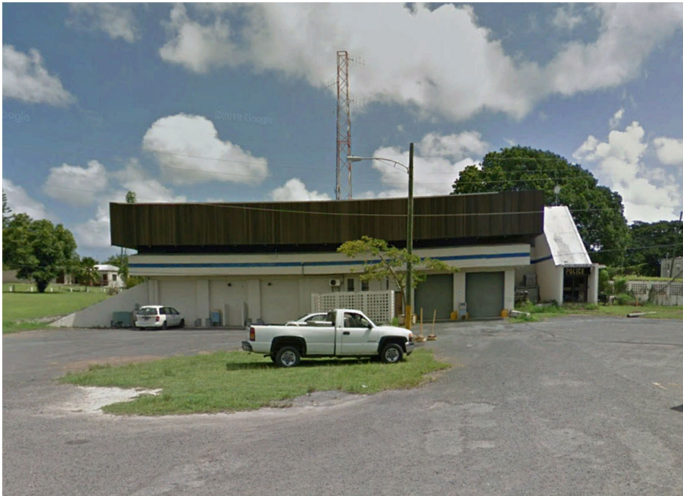
Photo 2 – Rear View of Administrative Office Site – Looking Northeast
