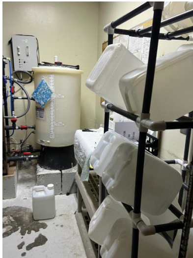
Figure 4 of 6: Hemodialysis department existing reverse osmosis system
