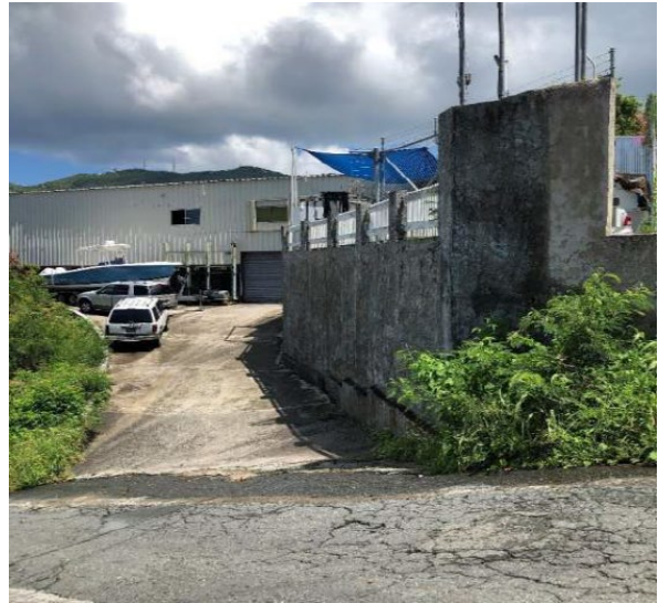
Figure 4 Woodworking Business, Lot 106
