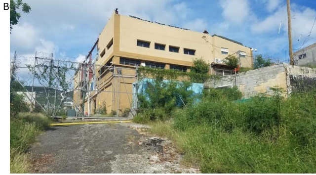
Figure 1 Swan Annex Building
