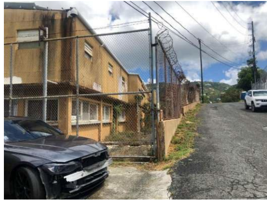
Figure 2 Swan Annex Building
