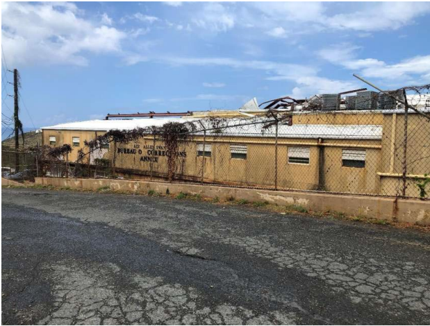
Figure 3 Swan Annex Building
