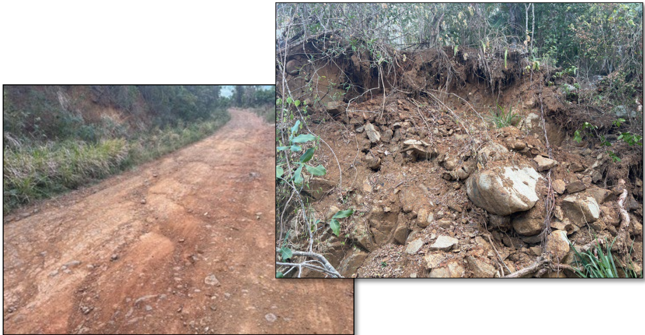
Figure 37. Road erosion (left) and undermined slope due to unmanaged stormwater (right).
