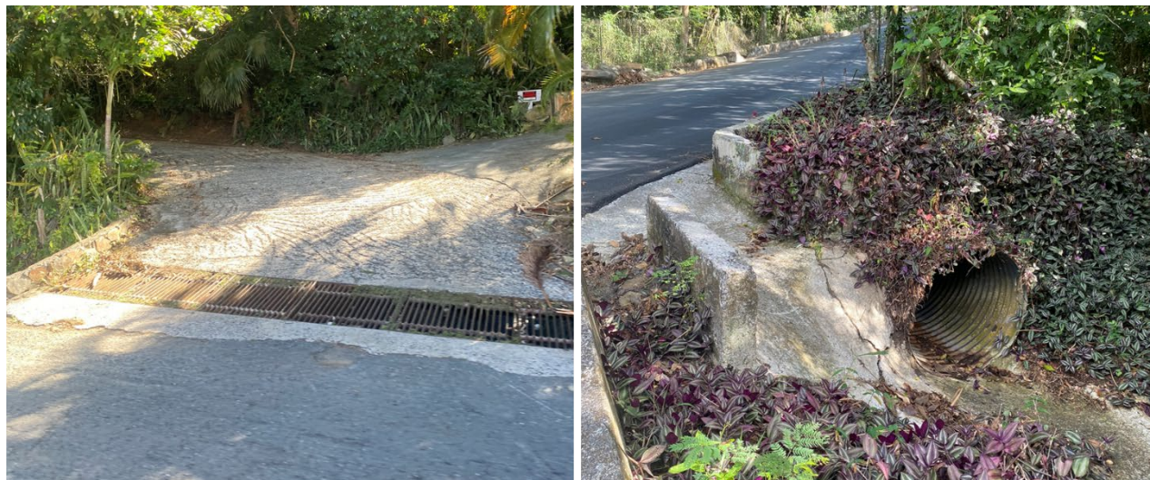
Figure 46. Examples of stormwater infrastructure. A trench drain (left) and a culvert (right).
