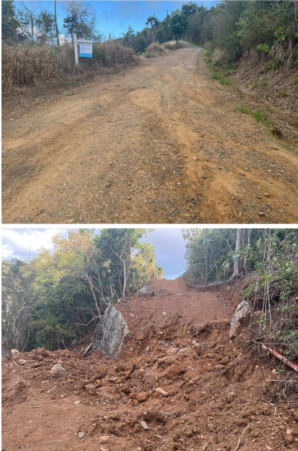
Figure 63. Stormwater runs down the road in many locations (upper) and new construction has not followed proper sediment and erosion control practices (lower).
