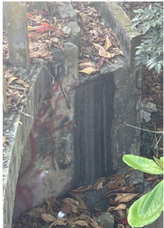
Figure 40. Suspected illicit discharge in gut.
