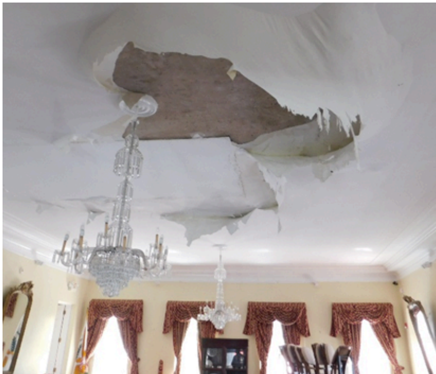
ATTNMENT RECORD Peppino Mangravite Murals, Government House USVI Page 1 [ONGOING TREATMENT] | Removal of protective facing material after vacuum consolidation.
