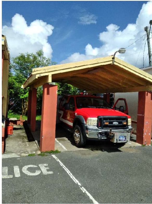
Photo 3 – Vehicular Garage Canopy Structure
