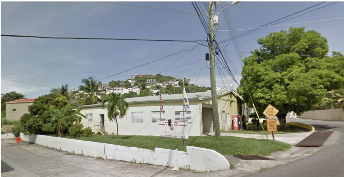
Photo 4 – Side View of Existing Facility – (West Elevation)
