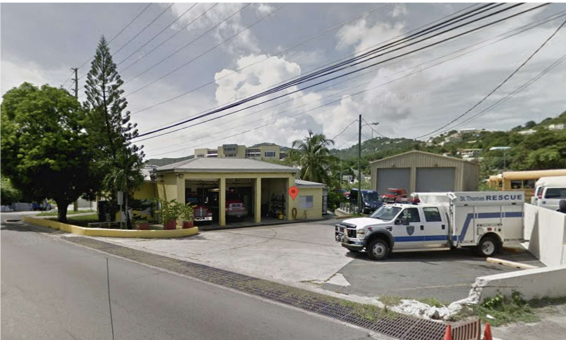
Photo 2 – Side View of Existing Facility – (East Elevation)
