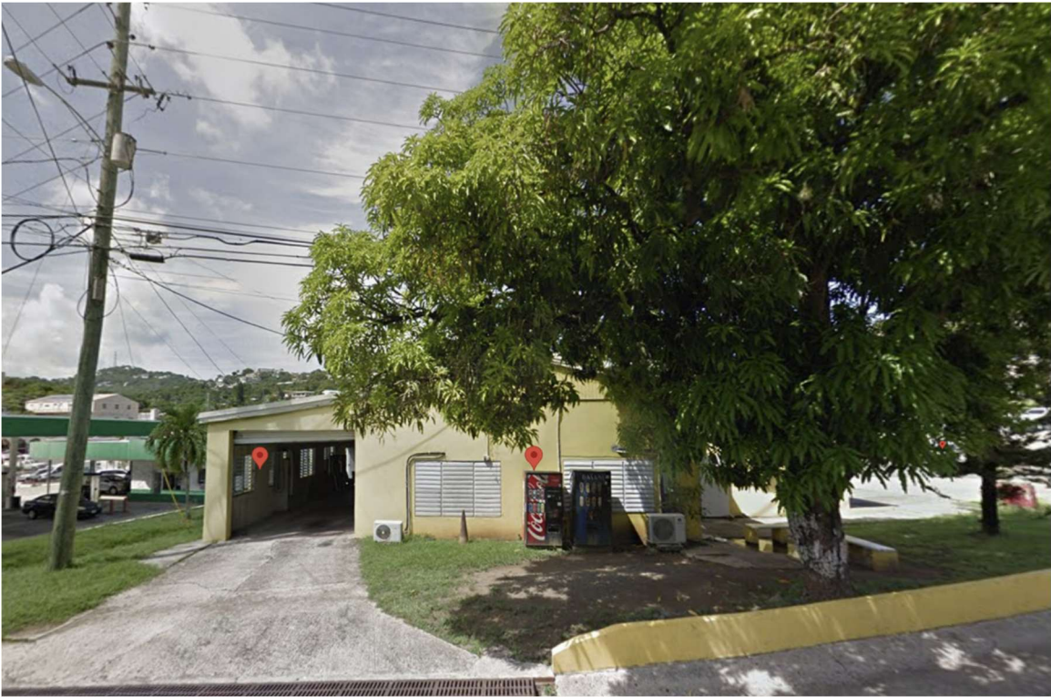
Photo 1 – Front View of Existing Facility – (South Elevation)
