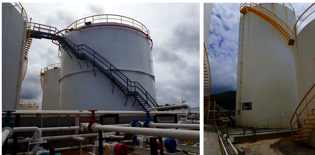
Figure 5.02.03.01 Five large steel tanks occupy most of the property. Three hold Jet Fuel, one holds diesel oil and a fifth tank is not in use.
