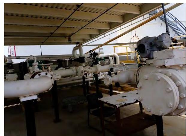
Figure 5.02.03.10 Two pipelines emerge from beneath the concrete slab to fill the Jet Fuel and diesel tanks at the facility. Only one line is currently used. The second is for redundancy and a back-up in case something happens to the other.
