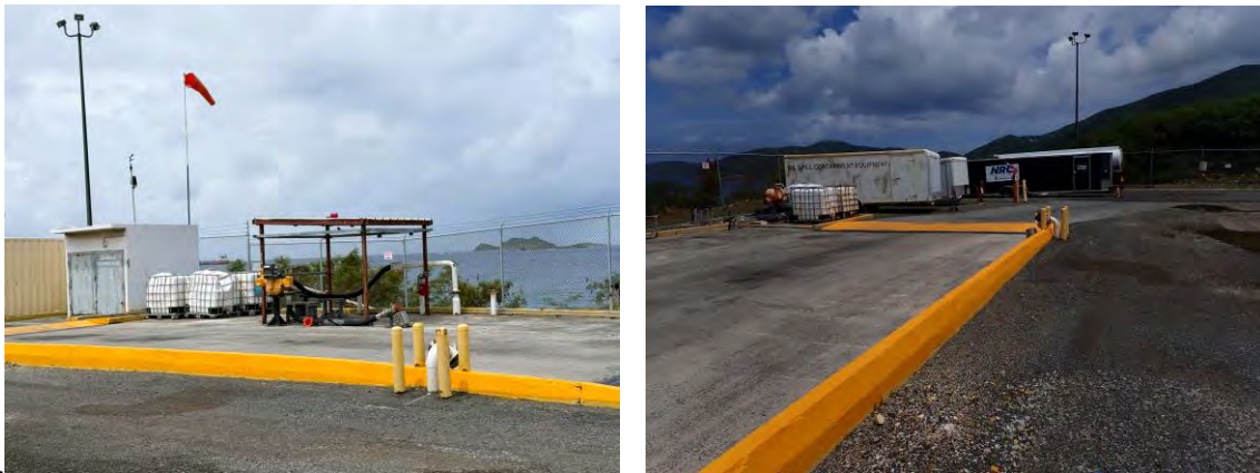
Figure 5.02.03.06 The Jet Fuel filling area is located west, across the site, along the coastal area of the property. A containment wall surrounds all piping and filling areas.
