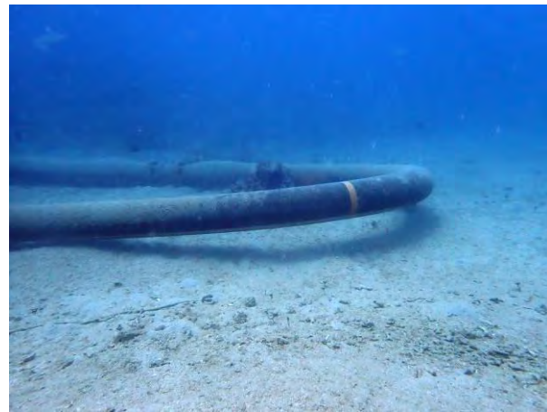
Figure 5.02.03.09 The pipelines are held to the seafloor with SubMar concrete mats until the free terminal ends where they are free to be picked up by tankers and used to transfer fuel.
