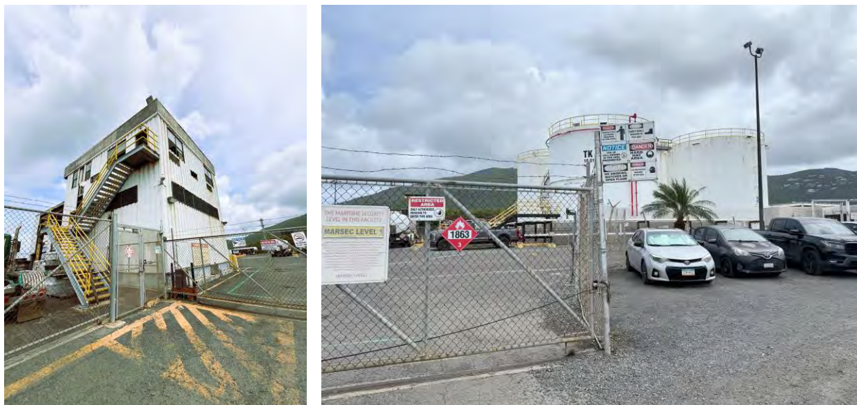
Figure 5.02.02.2. At the site the road is gated off and a chain link fence runs the periphery of the property.
