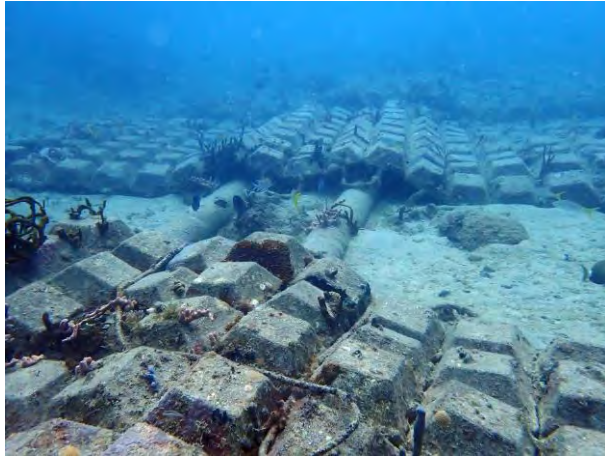
Figure 5.02.03.09 The pipelines are held to the seafloor with SubMar concrete mats until the free terminal ends where they are free to be picked up by tankers and used to transfer fuel.
