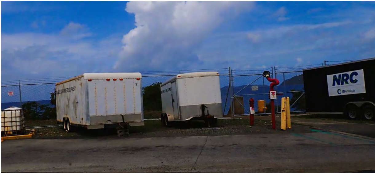
Figure 5.02.03.12. On the western edge of the property near the pipelines are trailers that hold oil spill equipment and supplies.
