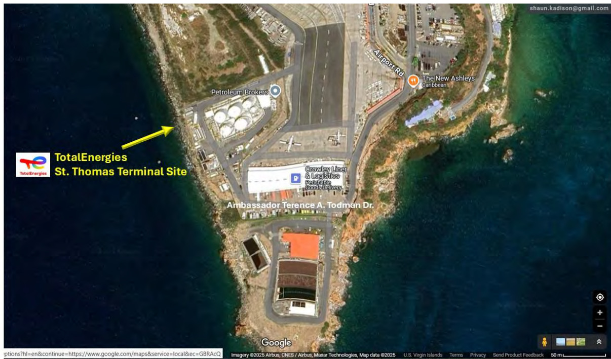
Figure 5.02.02.01 Airport Road runs south along the Cyril E King airport and becomes the Ambassador Terence A. Todman Rd, which accesses the fuel depot site.
