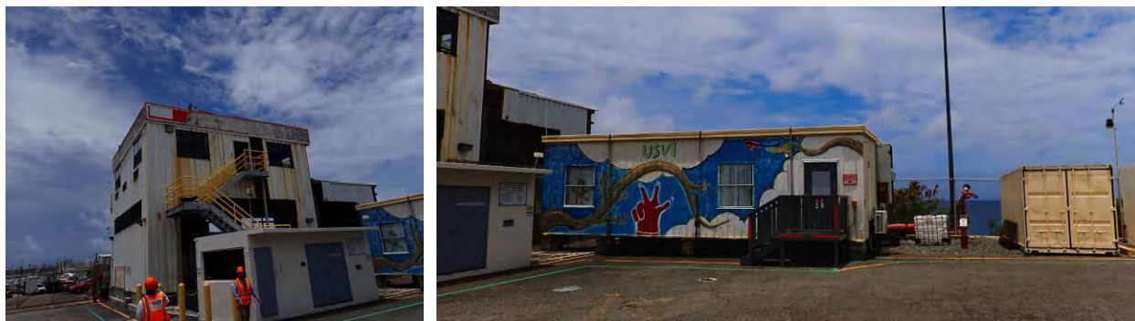
Figure 5.02.01.10. The old administration building was damaged in the storms of 2017 and now sits abandoned on the SW corner of the property. A trailer beside it currently serves as the administrative building. Next to it is a container with firefighting equipment which is not currently used. The depot now uses the Aircraft Rescue Fire Fighters (ARFF) based out of the adjacent Airport for emergency fire and explosion incidents. Improvements planned by TotalEnergies include reconstructing the administrative building and equipping the facility with a dedicated Firefighting system.
