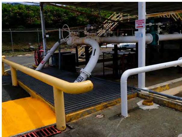
Figure 5.02.03.10 Two pipelines emerge from beneath the concrete slab to fill the Jet Fuel and diesel tanks at the facility. Only one line is currently used. The second is for redundancy and a back-up in case something happens to the other.
