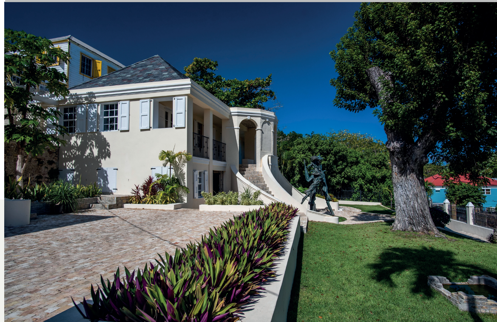
Restored building with landscaping in Christiansted
