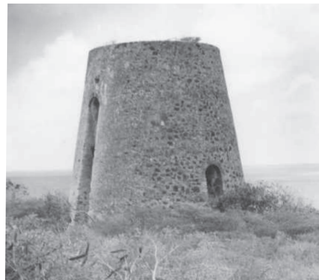
A coat of limewash can help to protect the surface of stone structures such as these.
