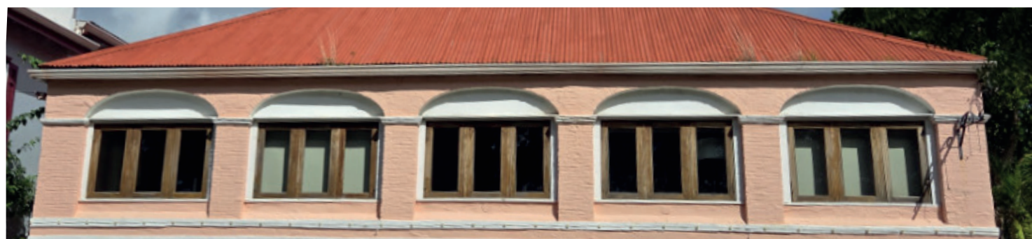
Strand Street 17, Frederiksted
