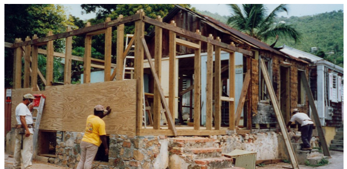
Lapped weatherboard and "German" or novelty siding.
