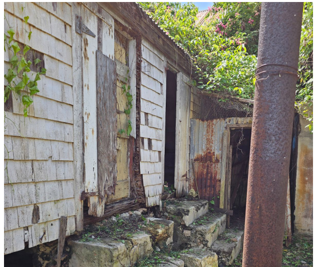
Illustration of wood rot before repairs.
