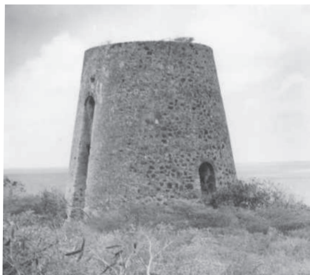
A coat of limewash can help to protect the surface of stone structures such as these.
