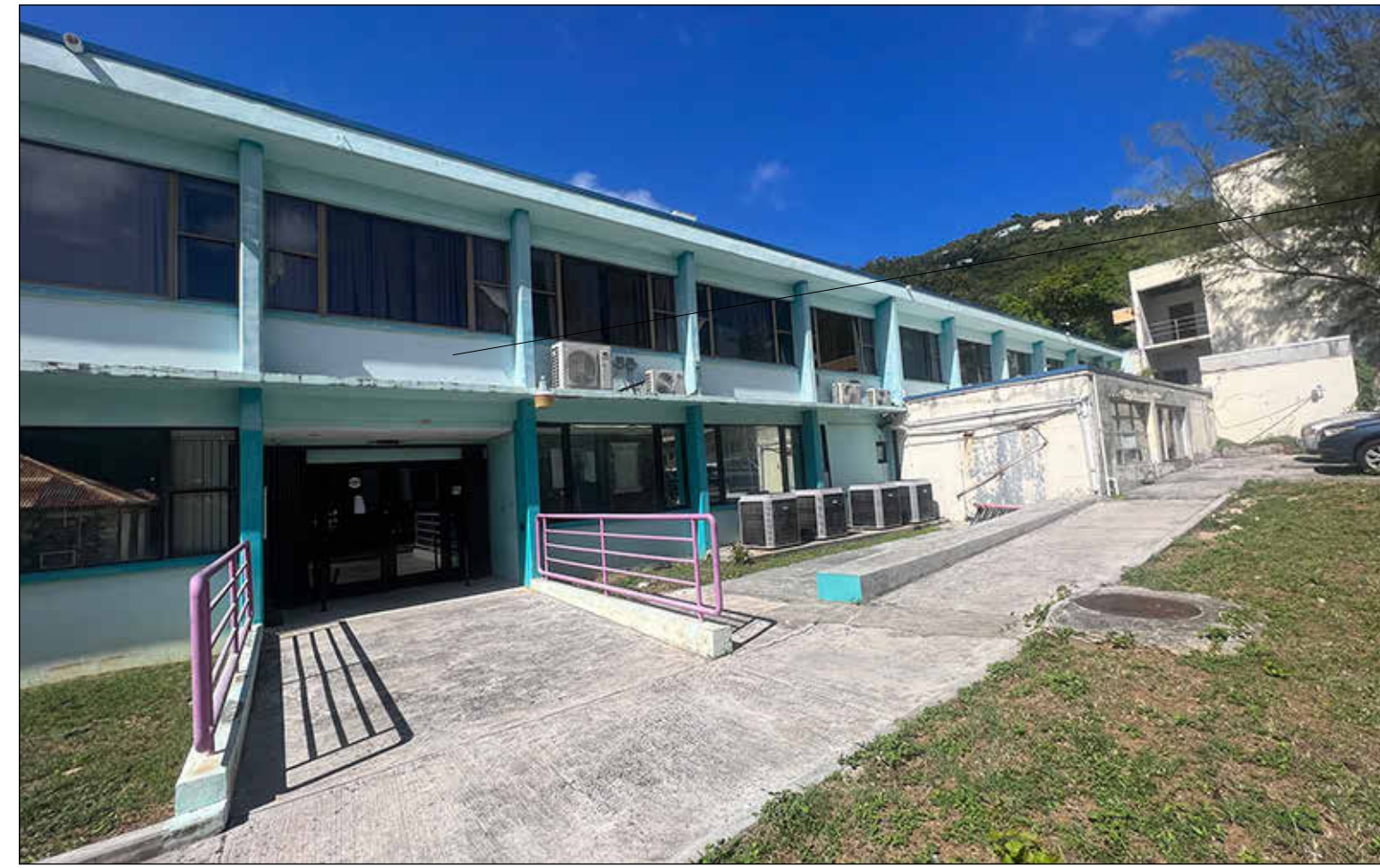
DHS KNUD HANSEN BUILDING - EAST FACADE (C)
