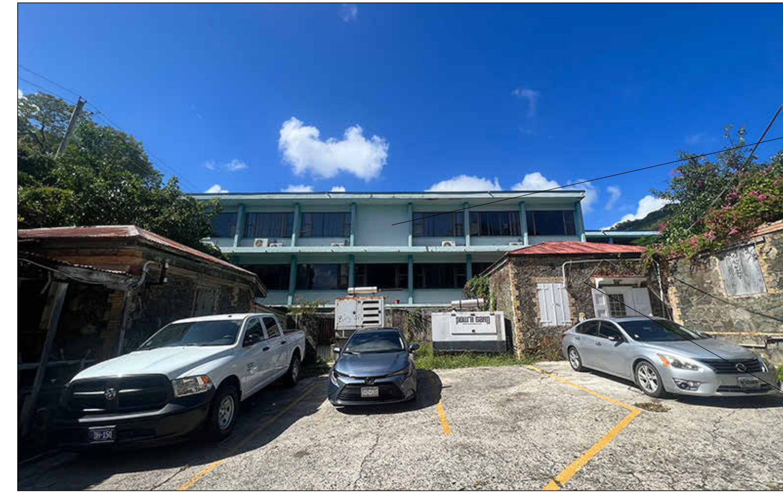
DHS KNUD HANSEN BUILDING - EAST FACADE (E)
