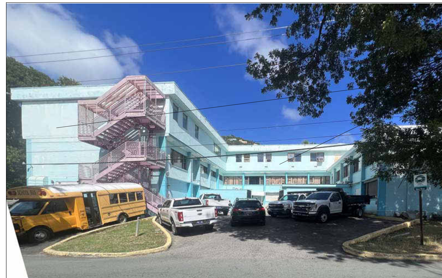
DHS KNUD HANSEN BUILDING - SOUTH FACADE (I)
