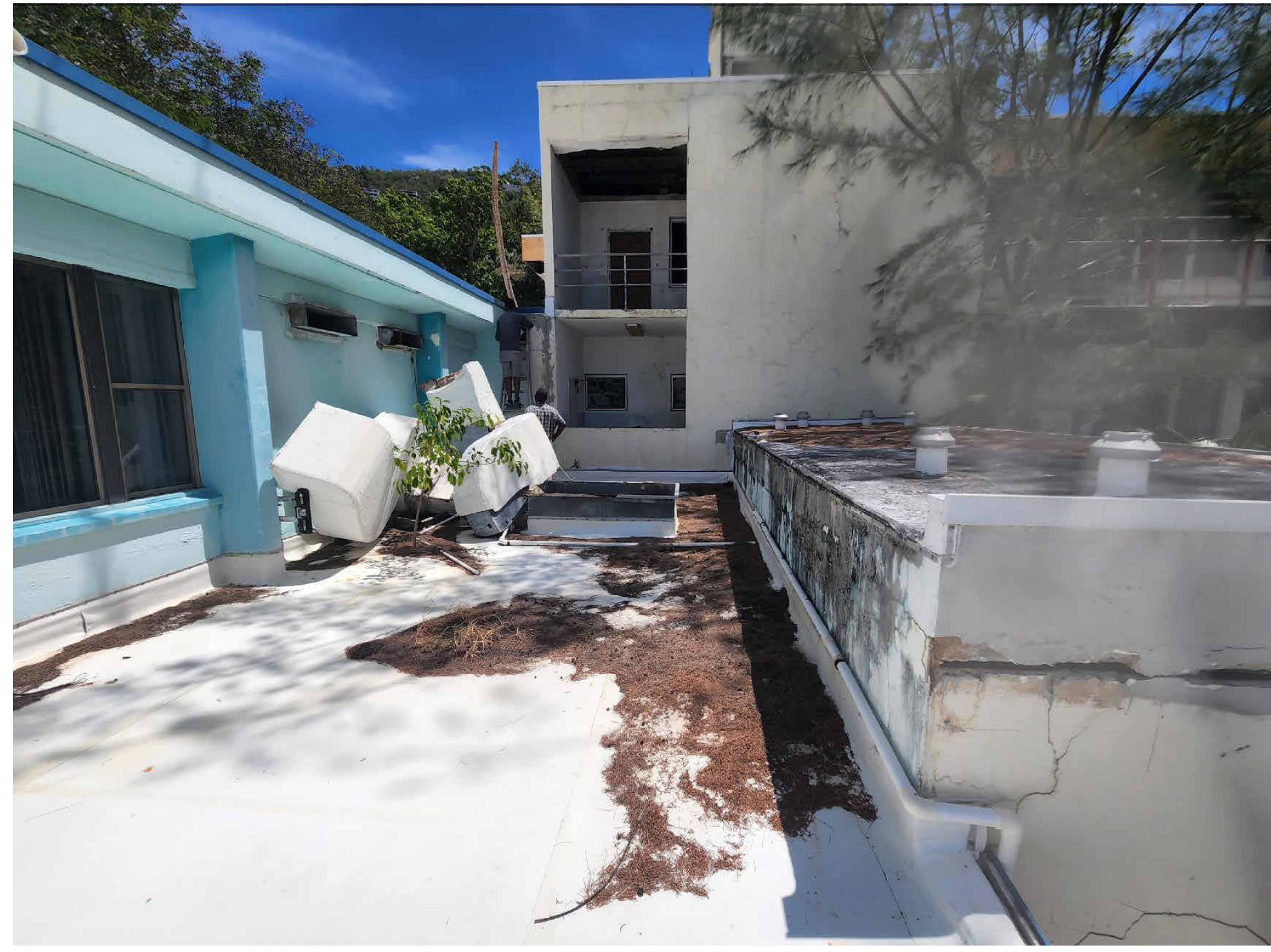
NORTH VIEW @ STORAGE ROOF
