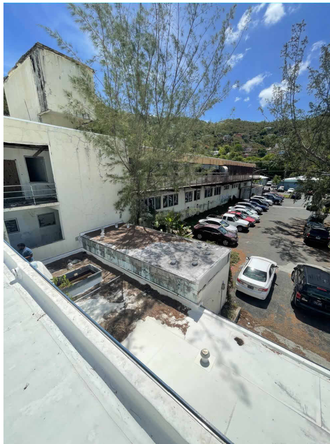
NORTH EAST VIEW @DHS ROOF
