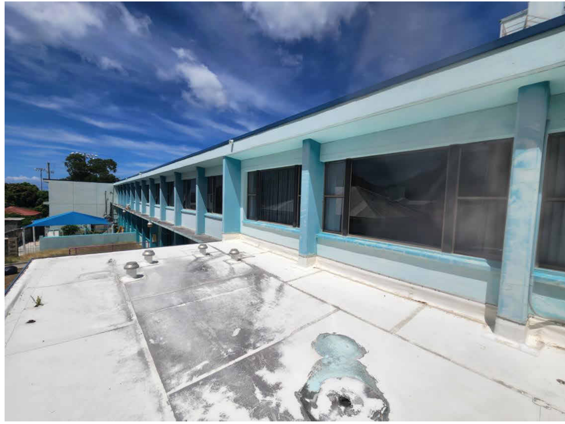
SOUTH VIEW @ STORAGE ROOF
