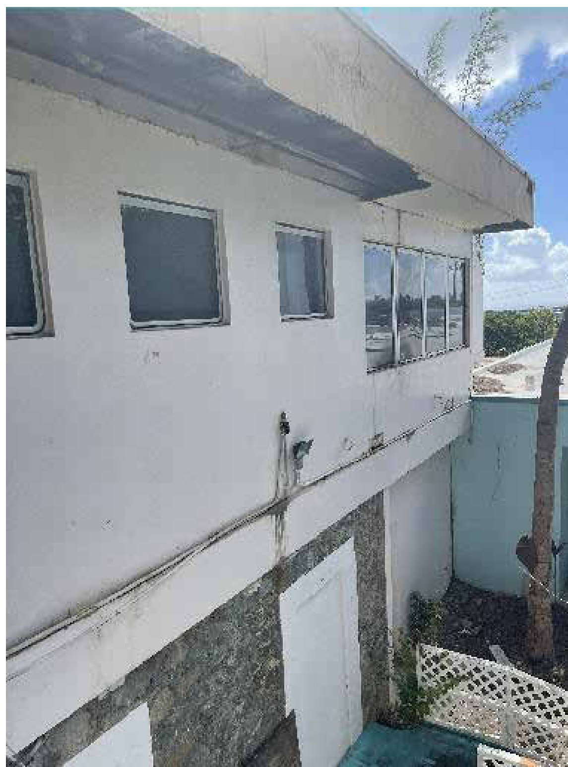
SOUTH VIEW @ CISTERN ROOF
