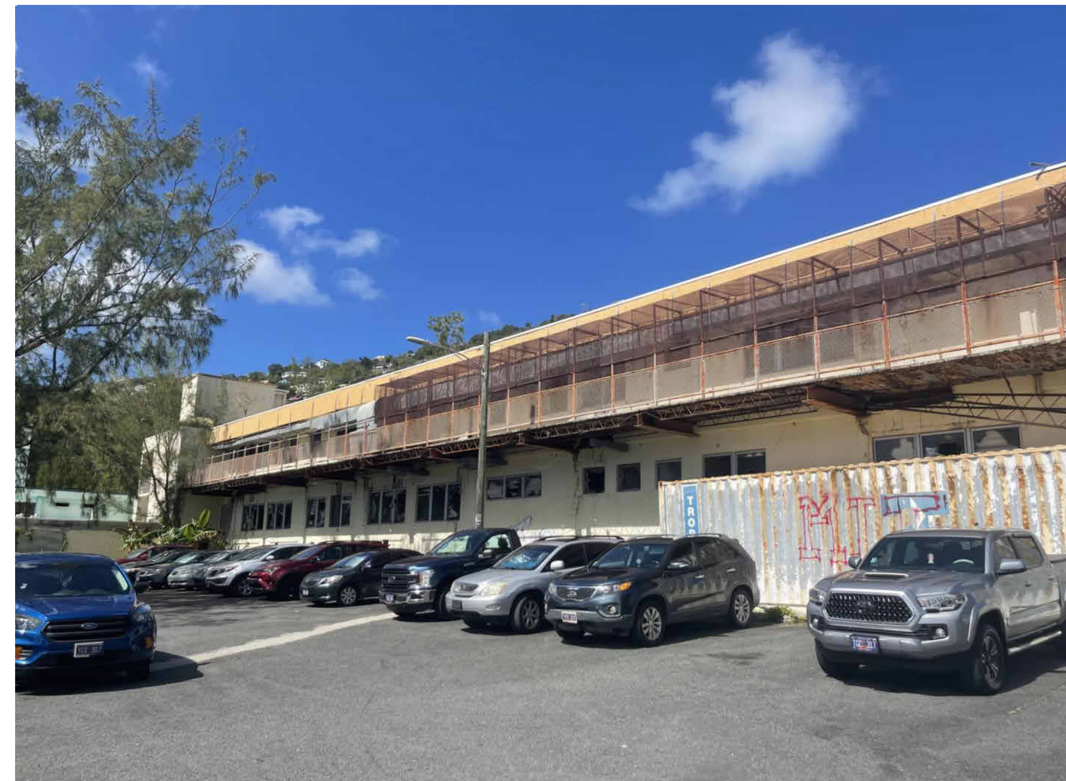
SOUTH ELEVATION OF THE OMH BLDG.
