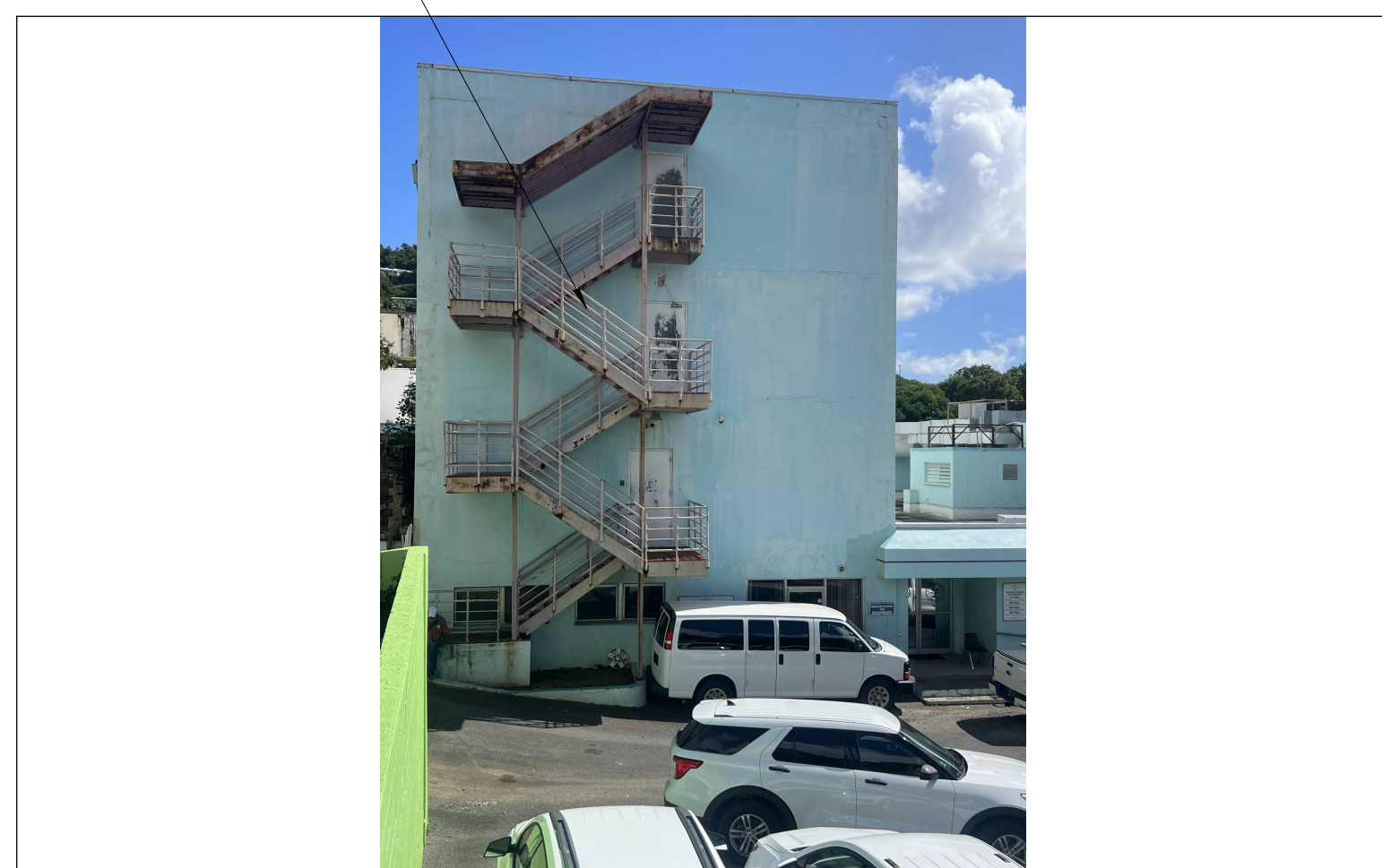
WEST FACADE STAIR TOWER, DOH KNUD HANSEN TOWER
