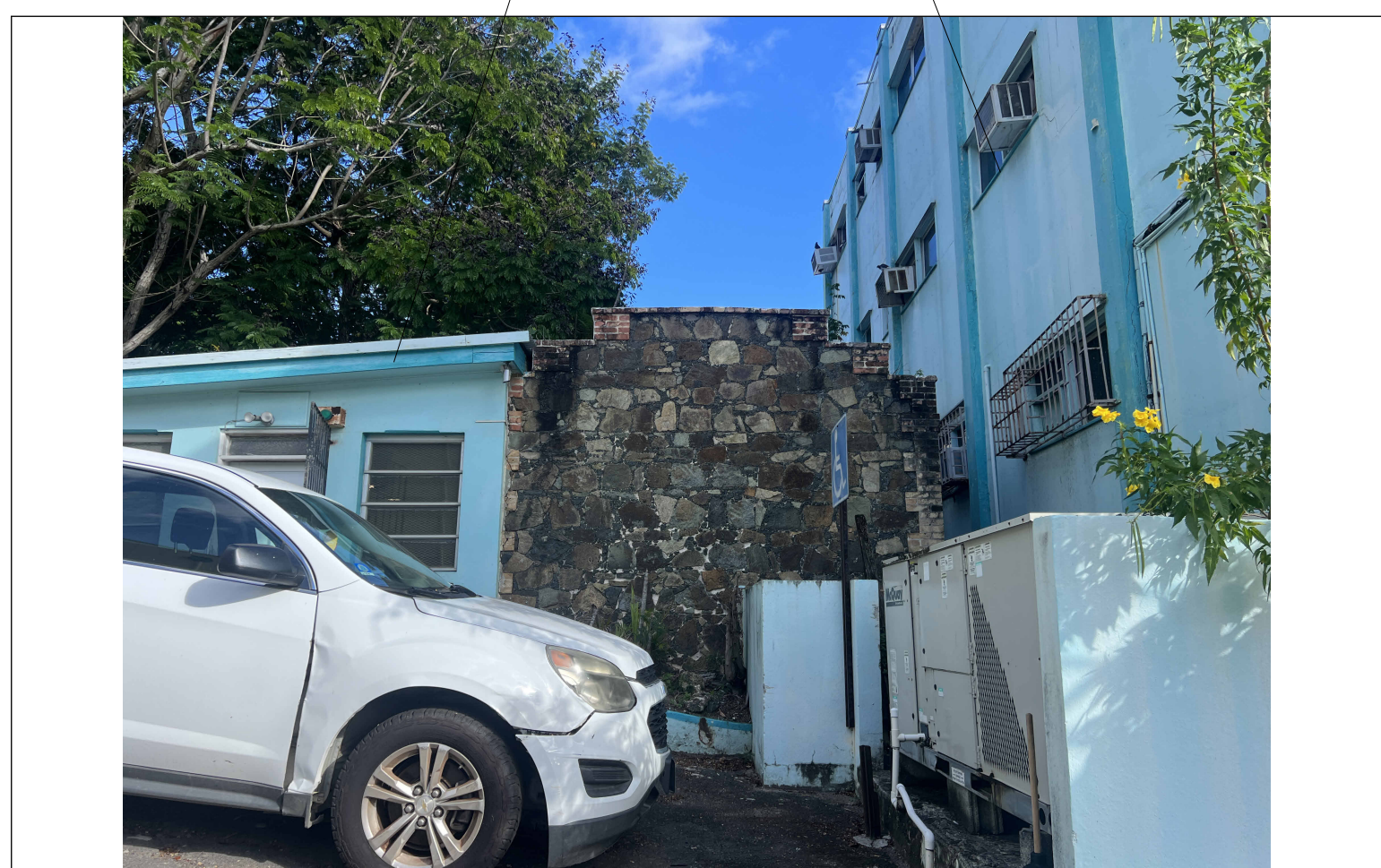
ADJACENT STRUCTURES, DOH KNUD HANSEN TOWER
