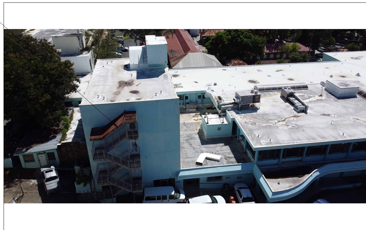
WEST FACADE & ROOF, DOH KNUD HANSEN TOWER
