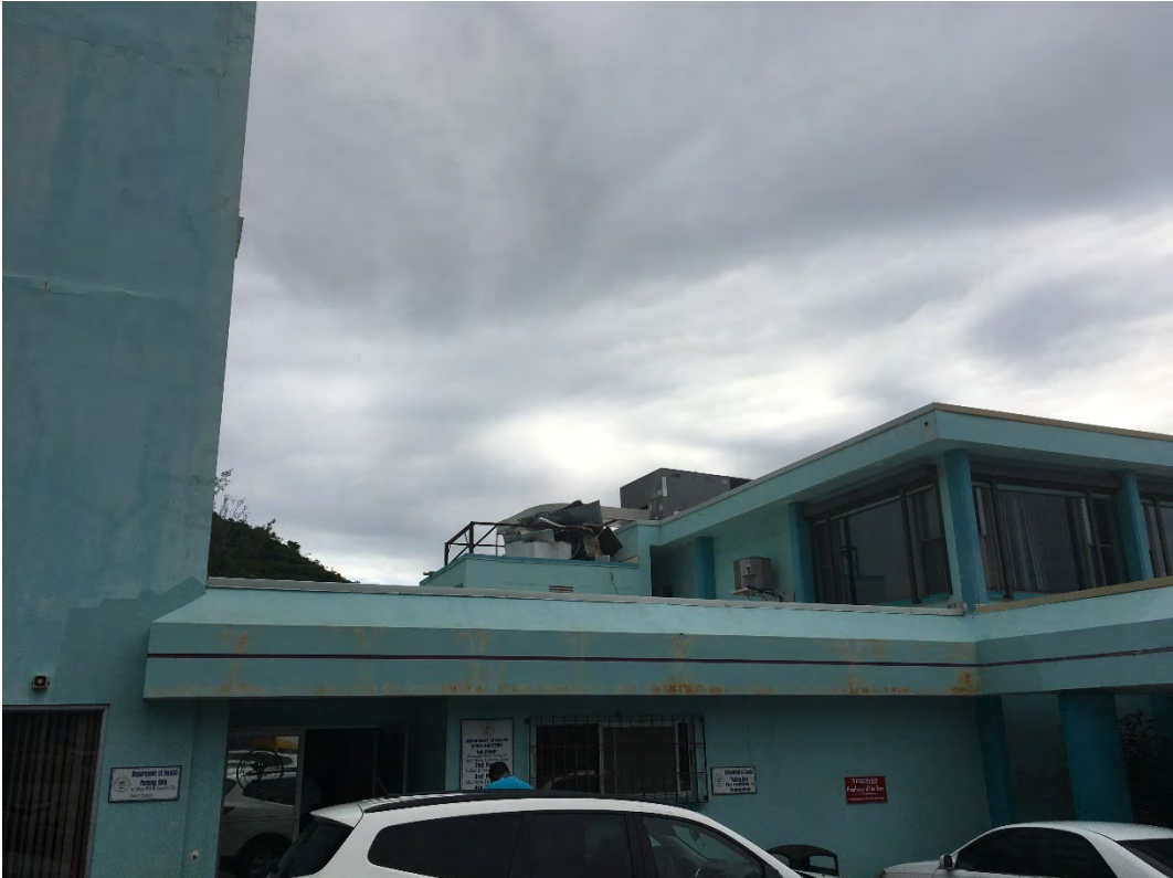
Photo 9: Knud-Hansen Tower west elevation
