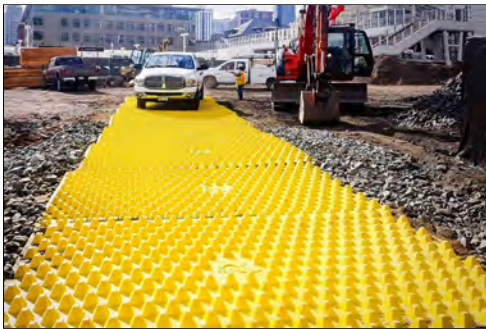
Trackout Control Mat
