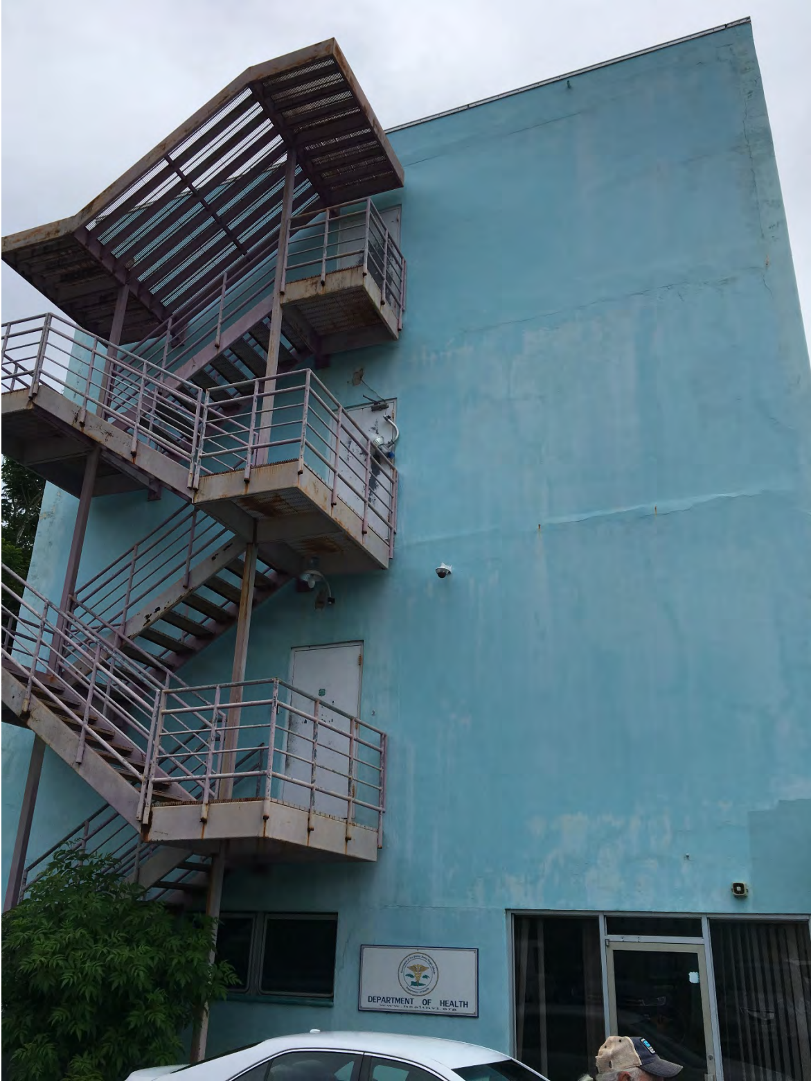
Photo 8: Knud-Hansen Tower west elevation
