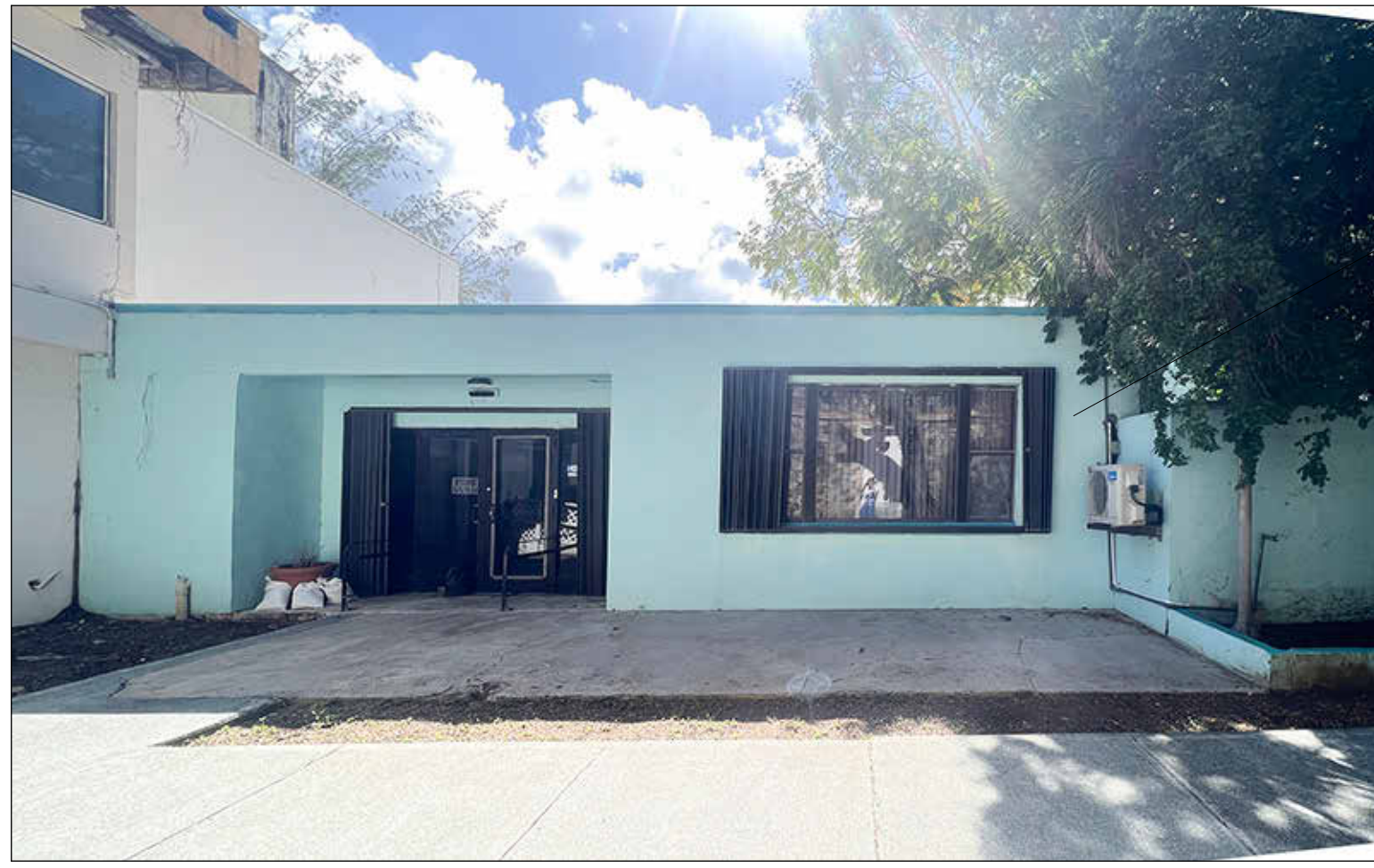
DHS KNUD HANSEN BUILDING - NORTH FACADE (B)
