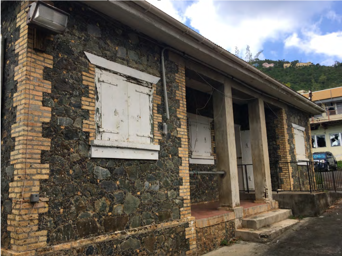
Photo 20: Moorehead Hospital Building 6 (F) – Communicable Disease Admin.
