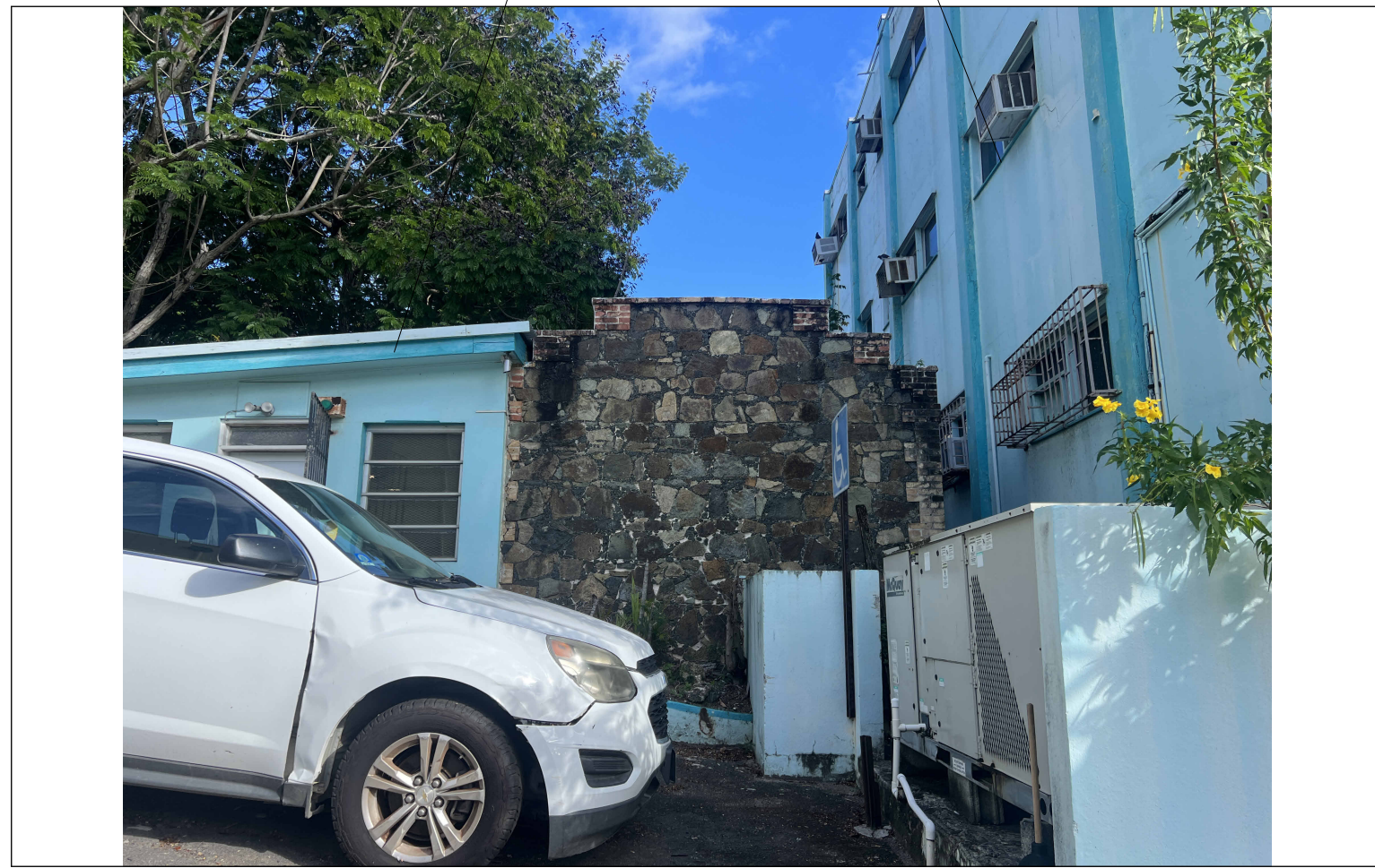
ADJACENT STRUCTURES, DOH KNUD HANSEN TOWER
