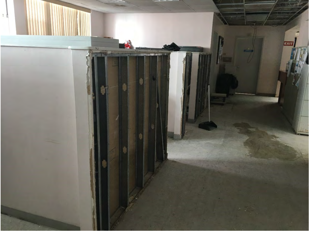
Photo 12: Knud-Hansen Tower interior
