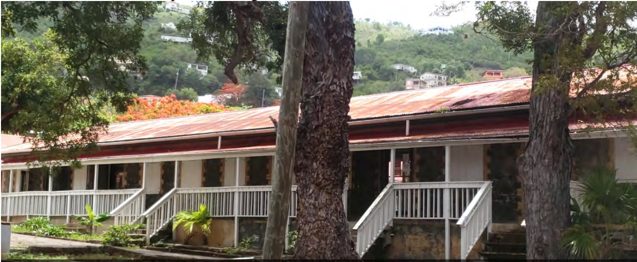
Photo 25: Moorehead Hospital Building 9 (I) – Communicable Disease Clinic
