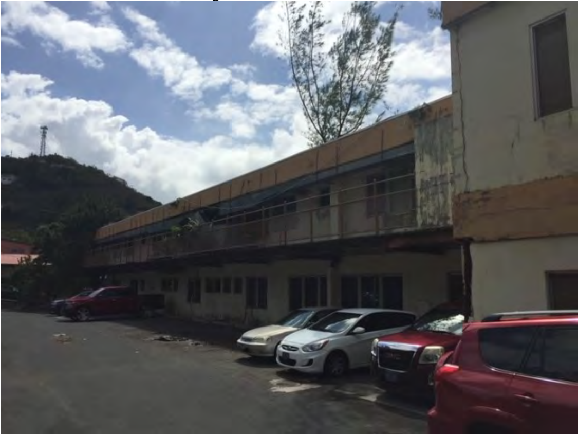
Photo 5: Mental Health Building north elevation
