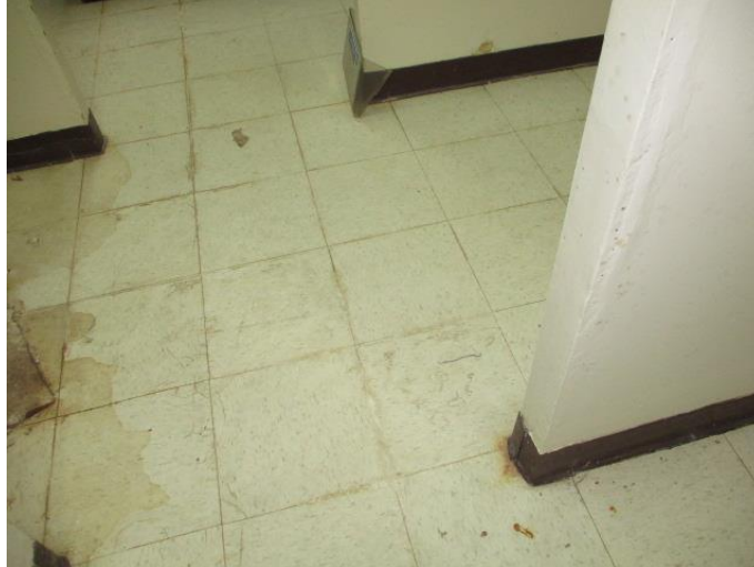
FLOORS 2, 3, 4; VYNIL FLOOR TILES WITH BLACK MASTIC; CREAM; APPROX. 6,000 SF
