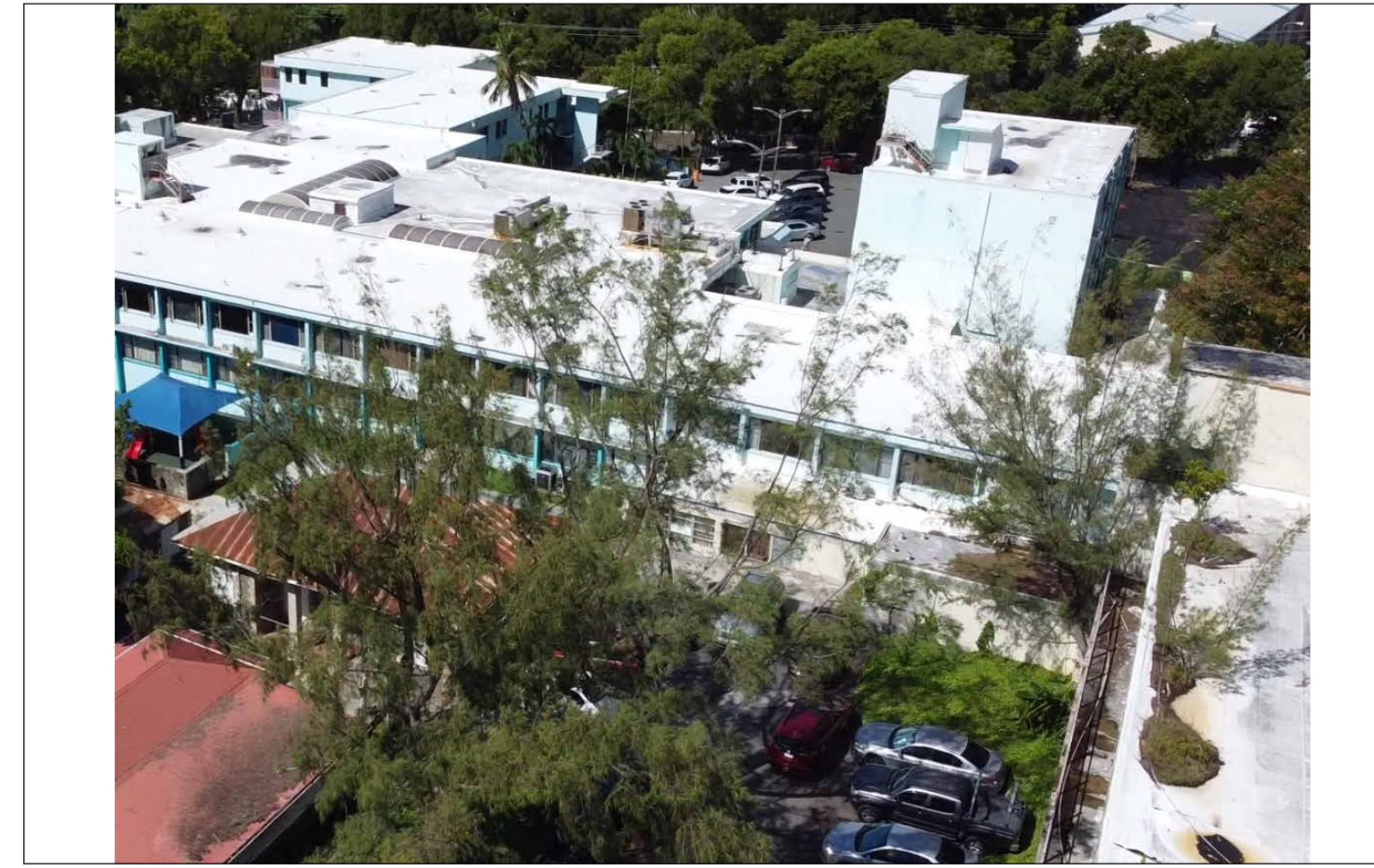
EAST FACADE, DOH KNUD HANSEN TOWER
