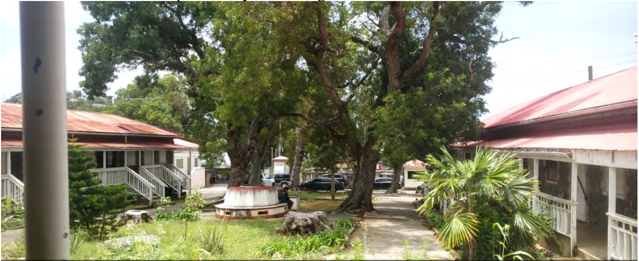
Photo 14: Moorehead Hospital courtyard looking south
