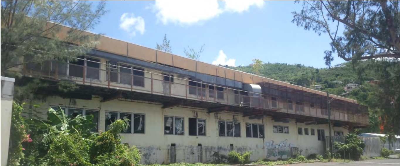
Photo 2: Mental Health Building south elevation
