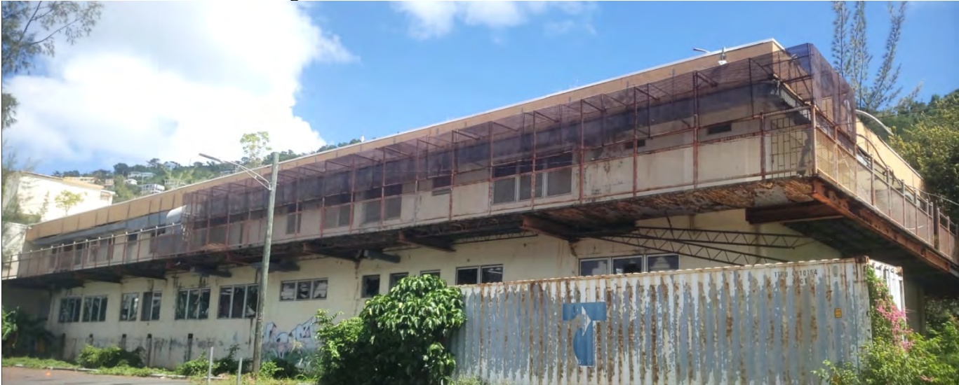
Photo 3: Mental Health Building southeast elevation
