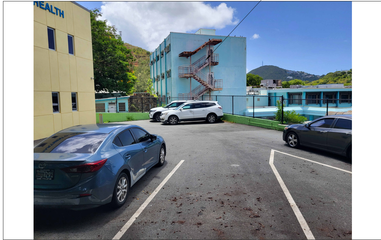
WEST FACADE, DOH KNUD HANSEN TOWER
