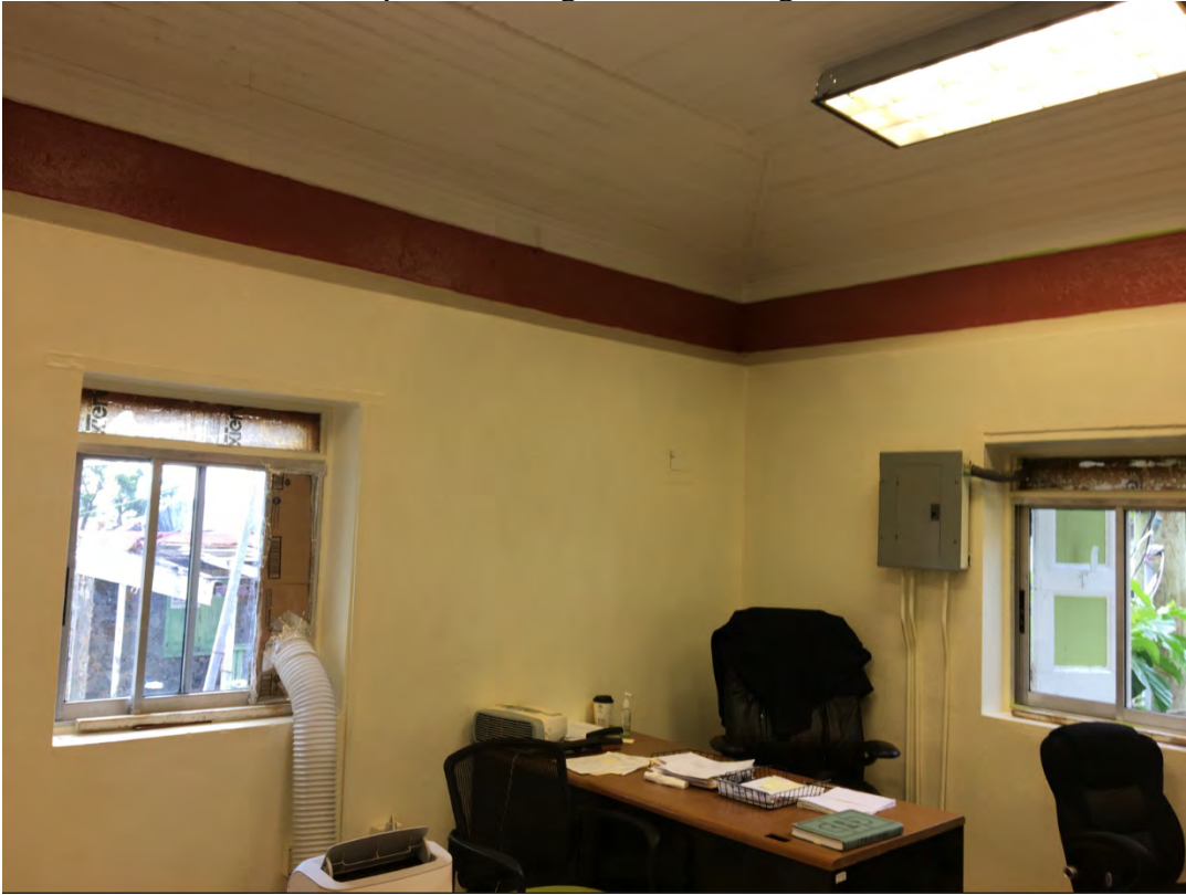
Photo 30: Moorehead Hospital Building interior ceiling
