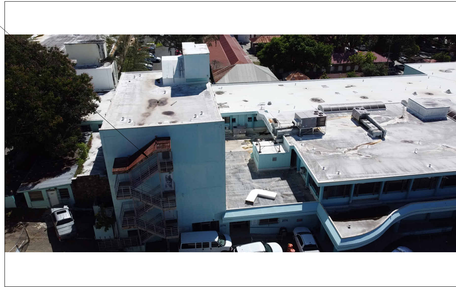
WEST FACADE & ROOF, DOH KNUD HANSEN TOWER
