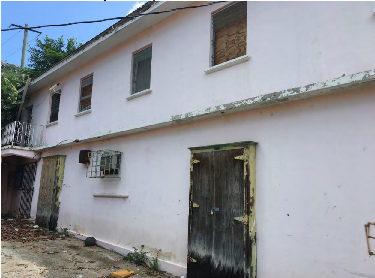
Photo 29: Moorehead Hospital Building 12 (L) – Women’s Resource Center west elevation
