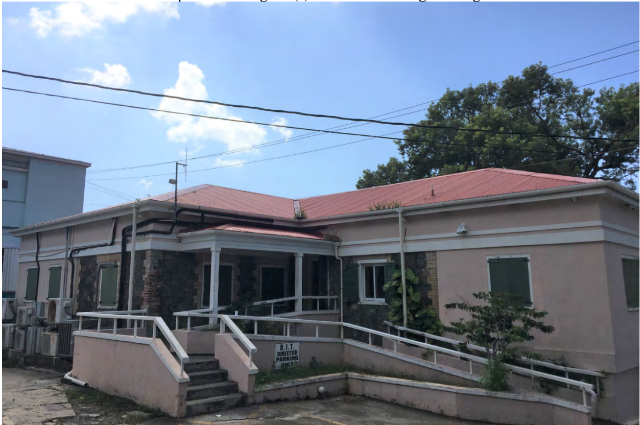
Photo 27: Moorehead Hospital Building 10 (J) – H.I.T. Building looking SE
