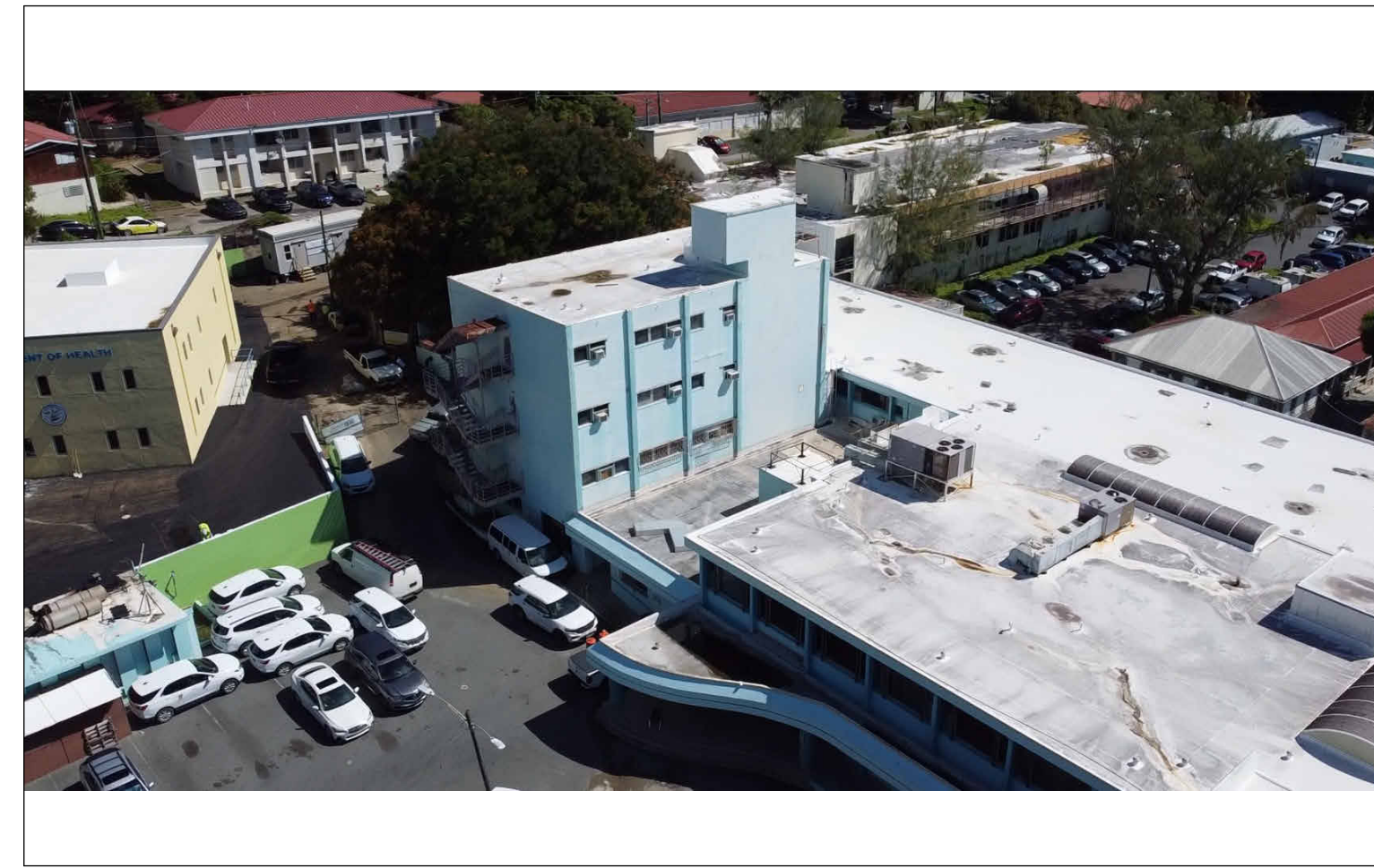
SOUTHWEST FACADE, DOH KNUD HANSEN TOWER
