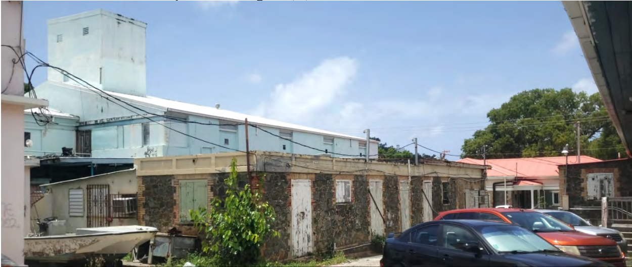
Photo 28: Moorehead Hospital Building 11 (K) – Maintenance
