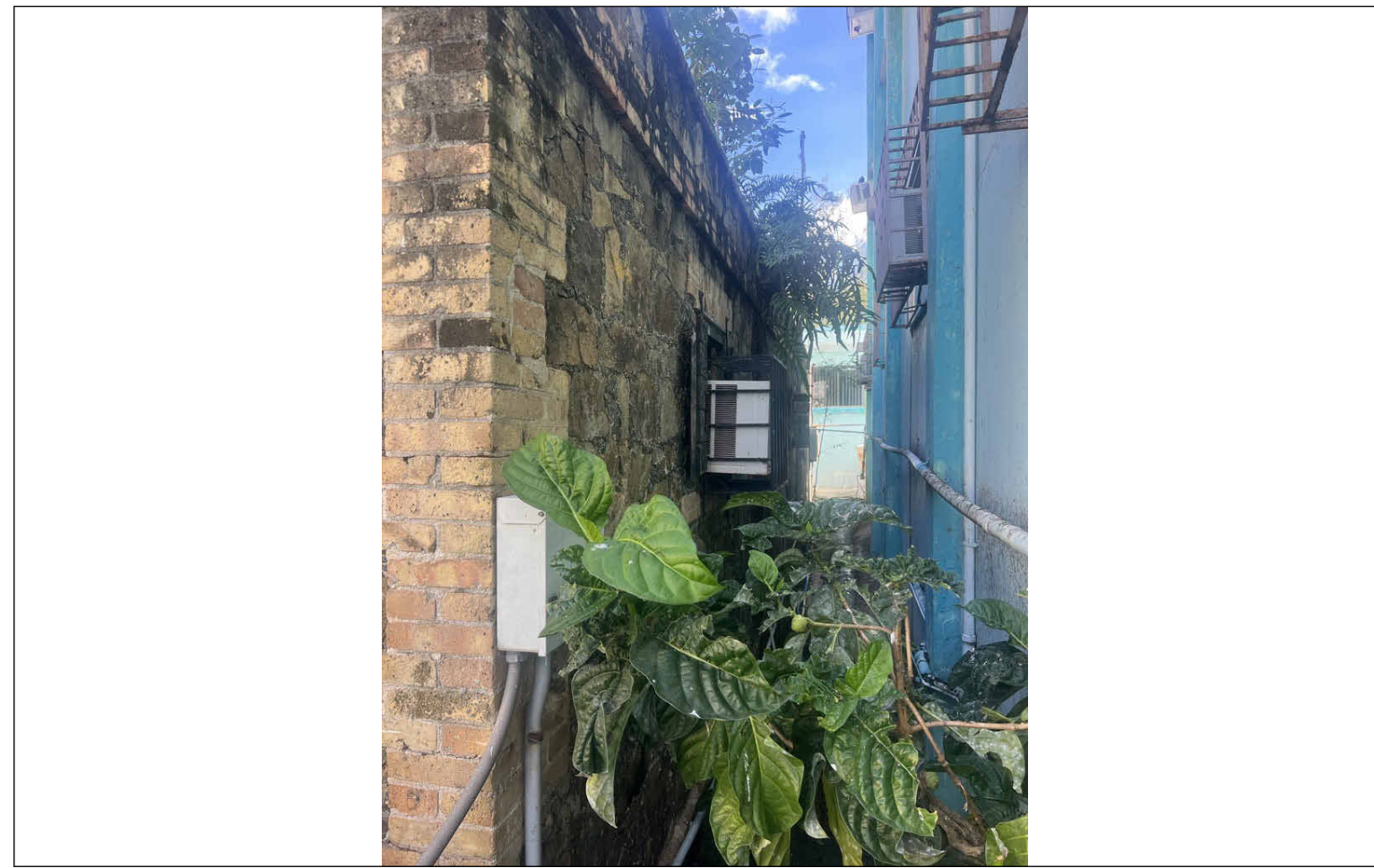
BETWEEN HISTORIC STRUCTURE & TOWER, DOH KNUD HANSEN TOWER
