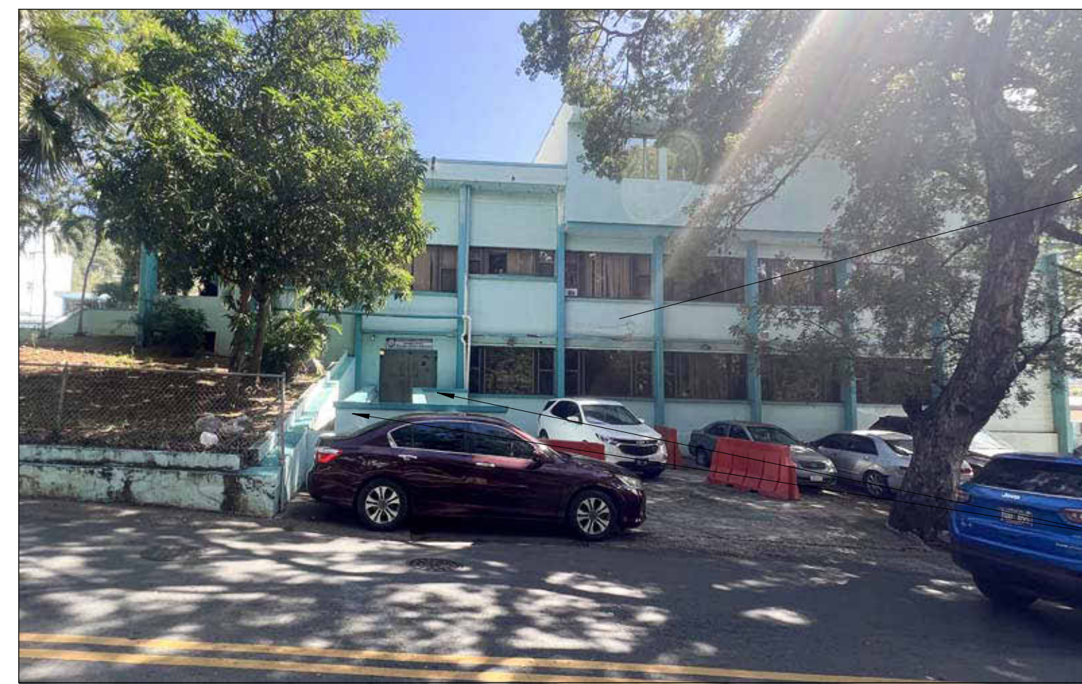
DHS KNUD HANSEN BUILDING - WEST FACADE (J)
