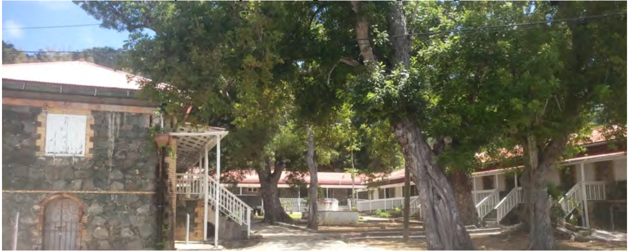
Photo 13: Moorehead Hospital courtyard looking NE showing buildings G, H, and I
