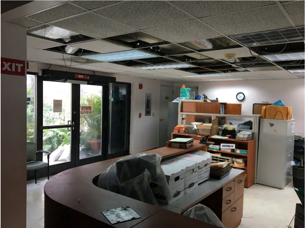
Photo 11: Knud-Hansen Tower interior
