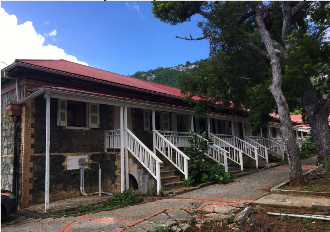
Photo 21: Moorehead Hospital Building 7 (G) – Environmental Health looking north
