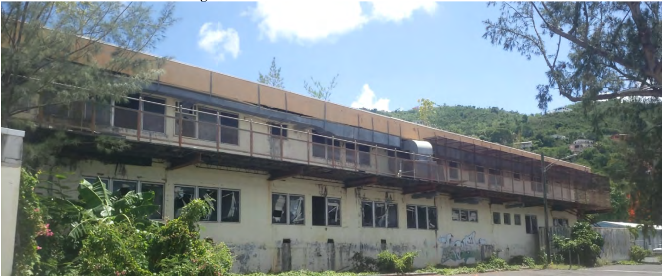
Photo 2: Mental Health Building south elevation
