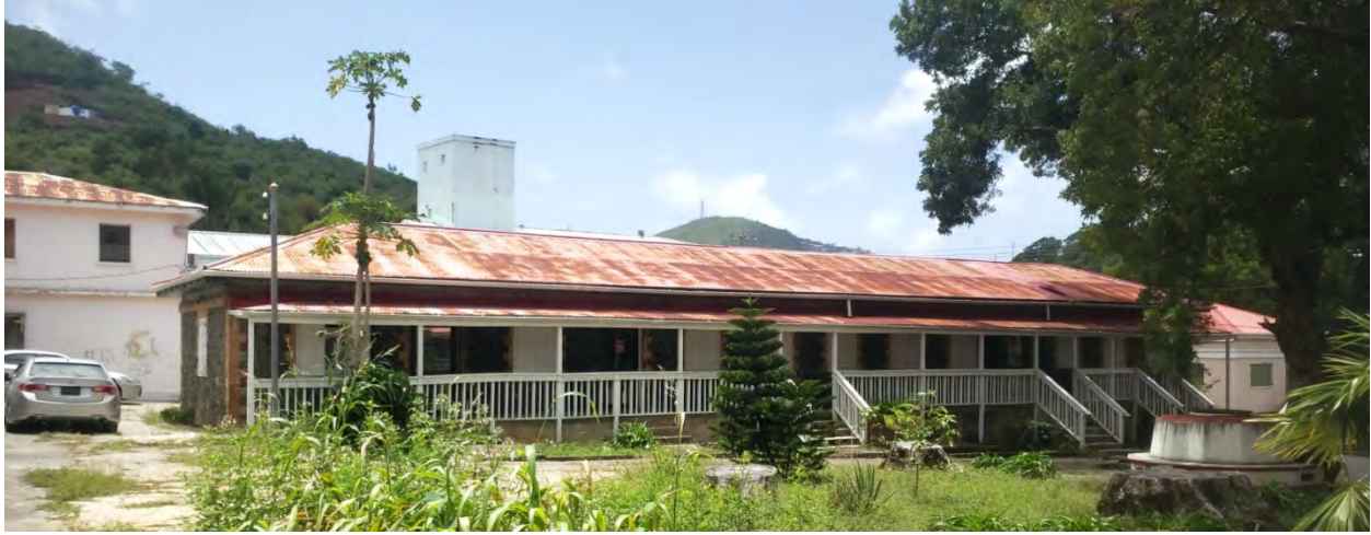
Photo 26: Moorehead Hospital Building 9 (I) – Communicable Disease Clinic (with Building 12 (L) to the left and Building 10 (J) to the right in the background)
