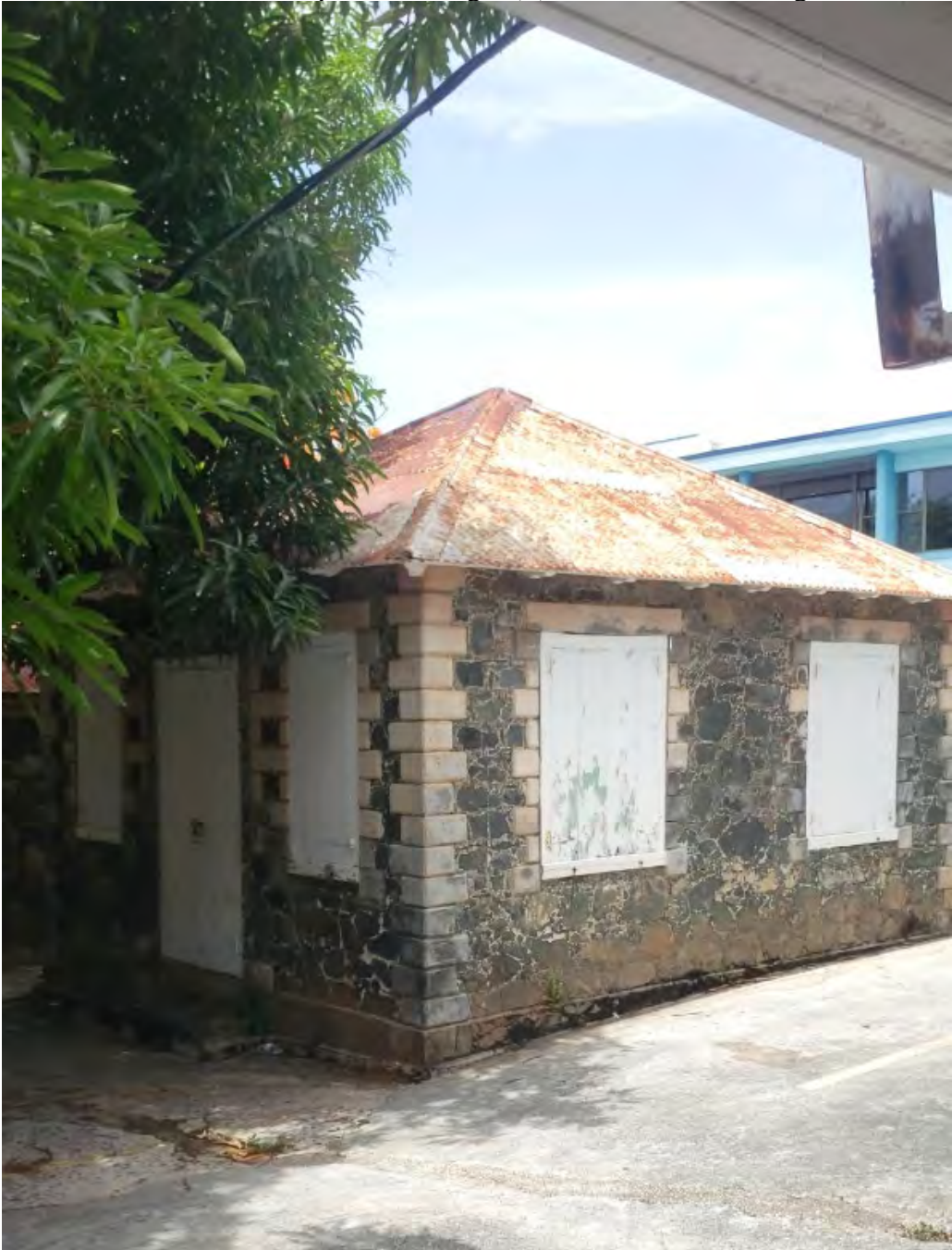
Photo 19: Moorehead Hospital Building 5 (E) – Director’s Building
