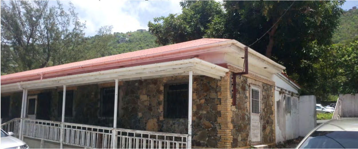
Photo 24: Moorehead Hospital Building 8 (H) – Vital Statistics looking west
