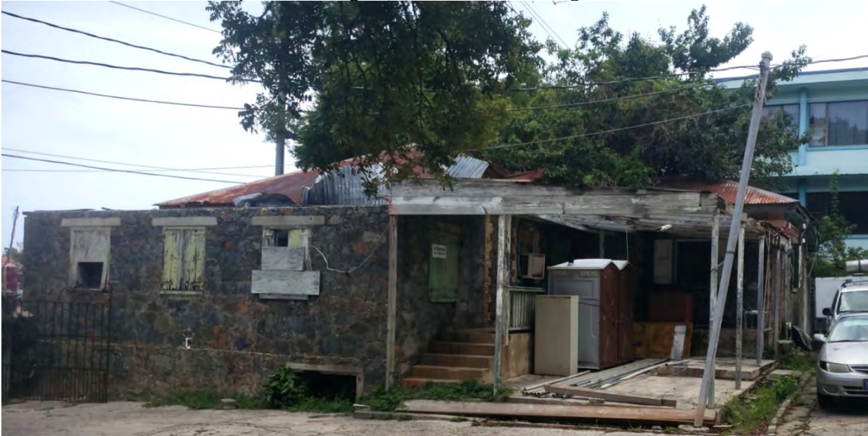
Photo 15: Moorehead Hospital Building 2 (C) – Chemical Storage
