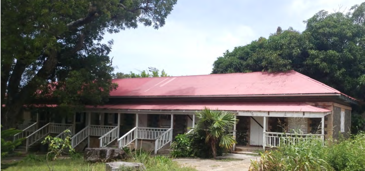
Photo 22: Moorehead Hospital Building 7 (G) – Environmental Health looking west
