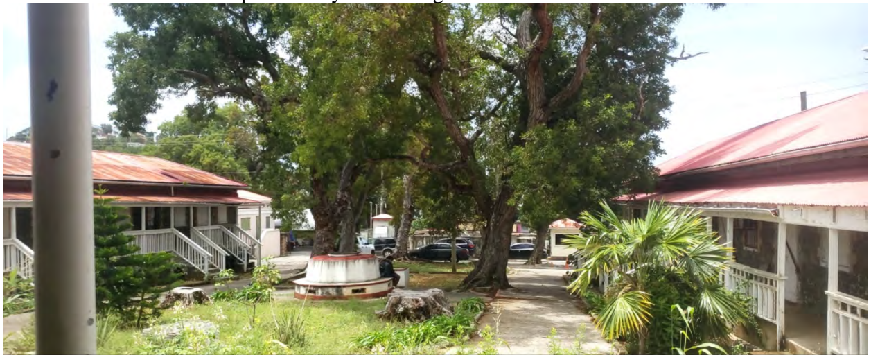
Photo 14: Moorehead Hospital courtyard looking south
