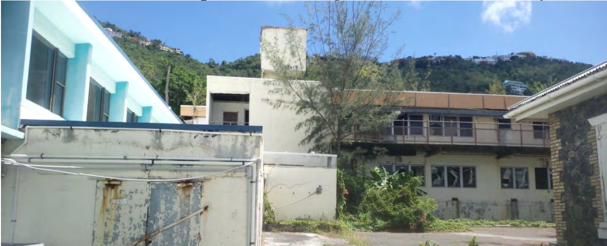
Photo 1: Mental Health Building south elevation and junction with Knud-Hansen complex
