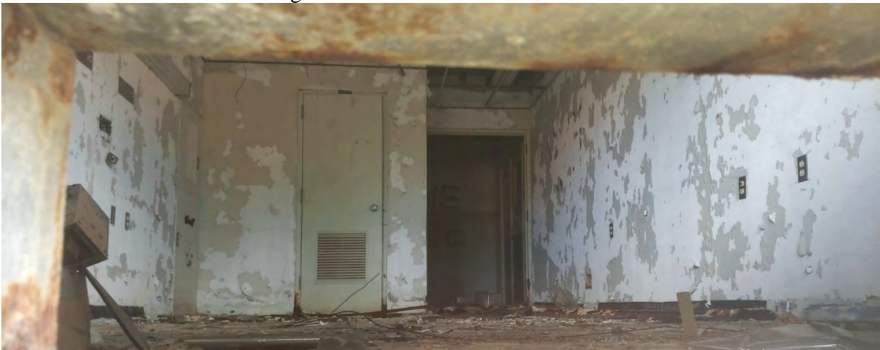
Photo 6: Mental Health Building interior
