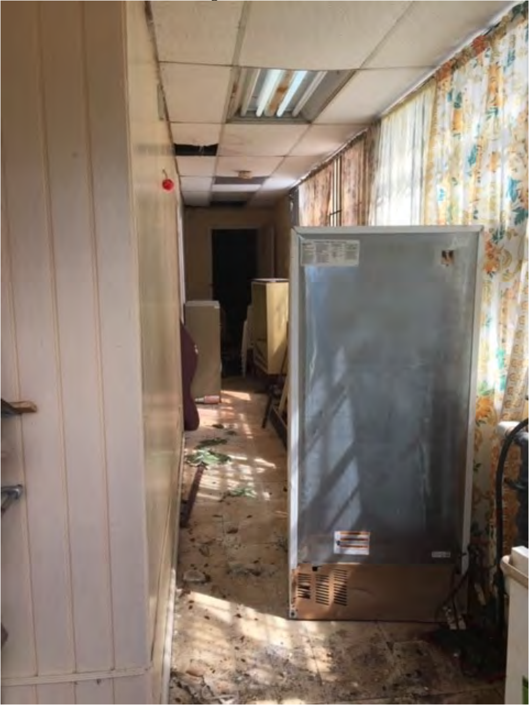
Photo 7: Mental Health Building interior
