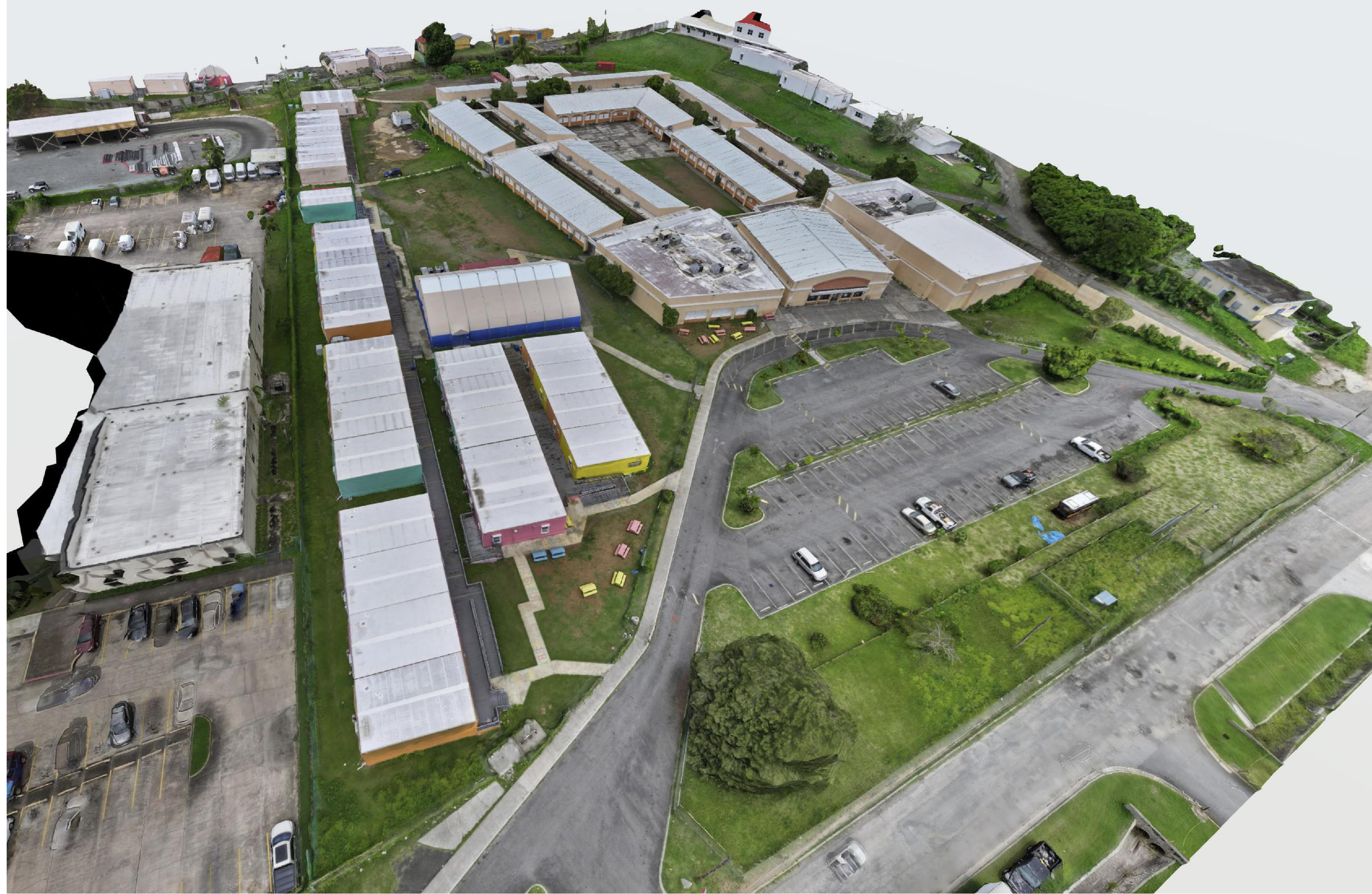
EXISTING SITE PHOTO FACING NORTHWEST Copy
