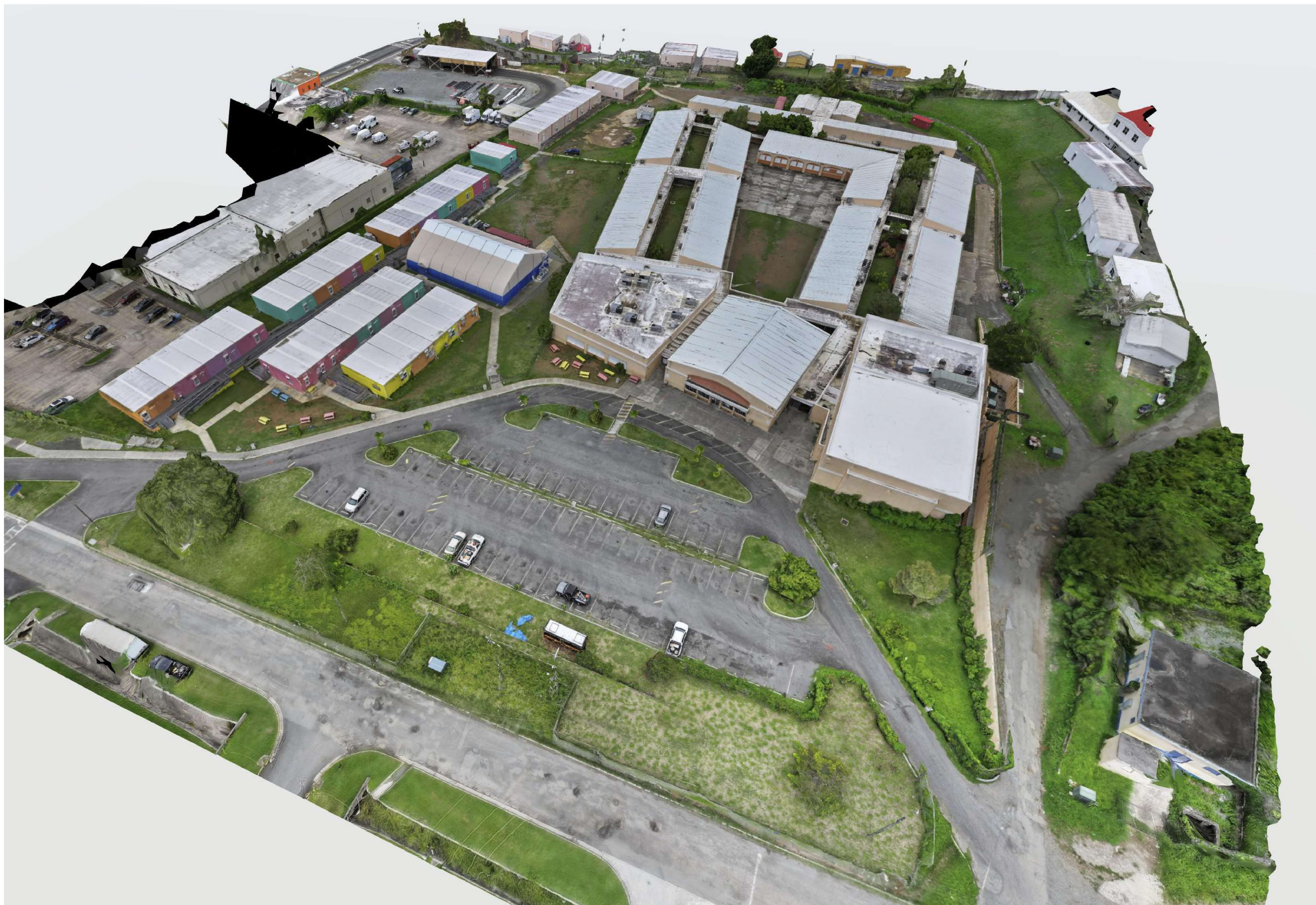
EXISTING SITE PHOTO FACING SOUTHWEST Copy
