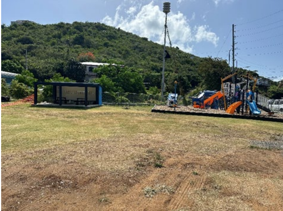
Photo 2: Looking at the Ballpark and the renovated dug-out
