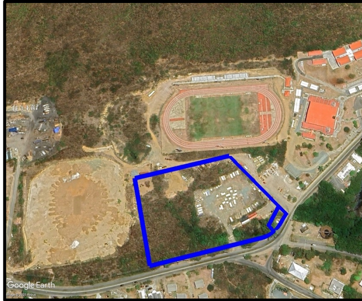
Figure 6: Google Earth image depicting existing conditions at the subject property (outlined in blue) in 2023.
