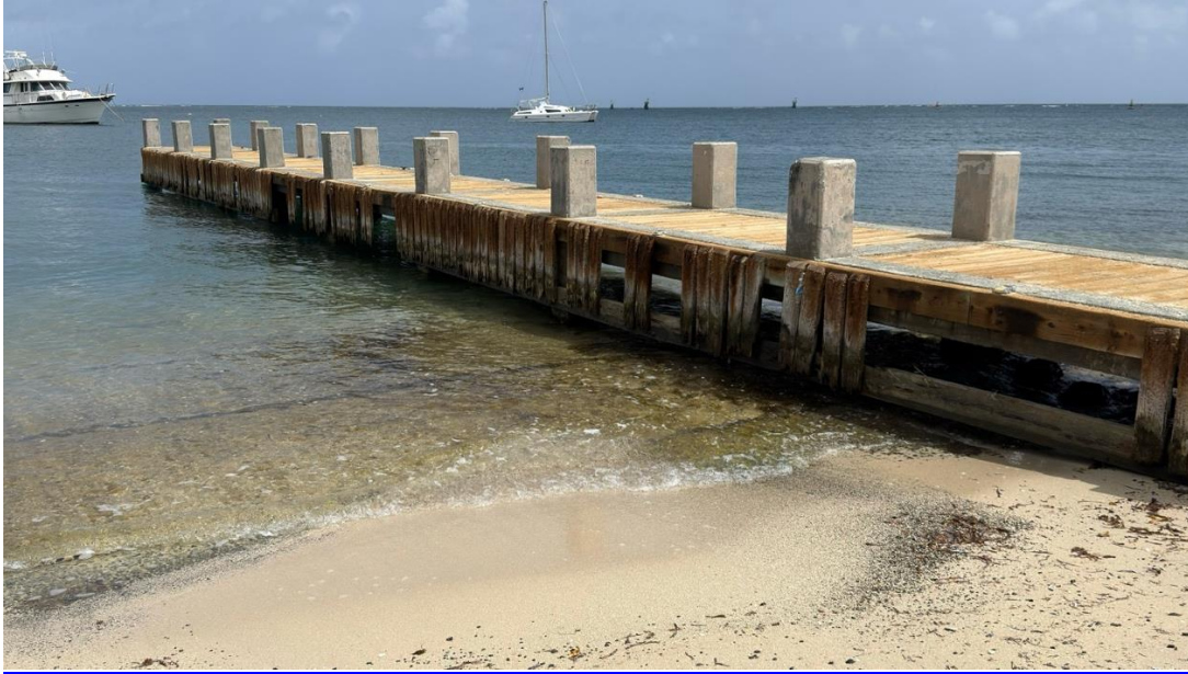
Figure1. Altona Lagoon dock prior to renovations taking place.
