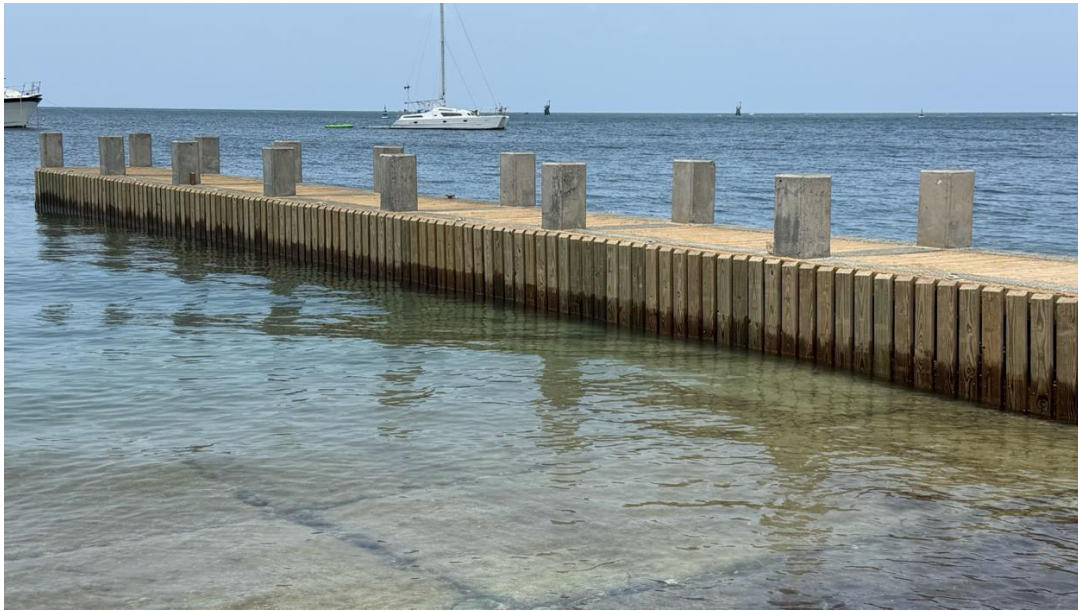
Figure 2. Altona Lagoon dock after installation of new beam and skirting woods.
